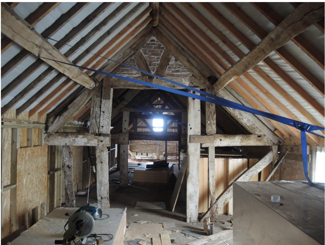
Figure 1 - Part of the timber frame construction to shippon 1 which might originate in the C16
