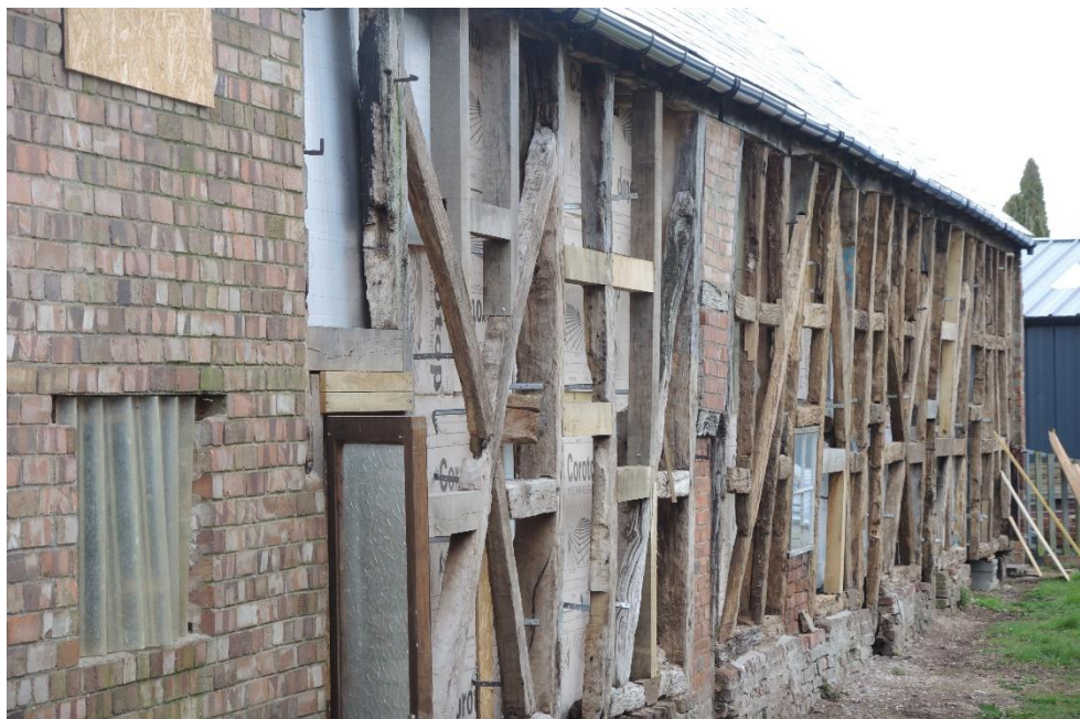
Figure 4 - Image of the NE facing elevation and the timber frame structure of shippin 1
