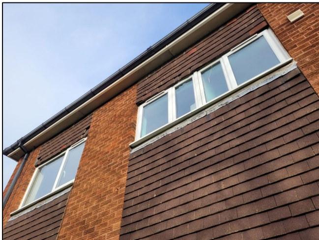
Photograph 3 Example of raised vertical tiles and view of soffit box and brickwork
