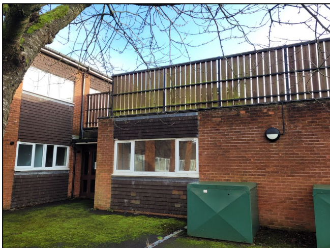
Photograph 4 The balcony area on the south-west of the building
