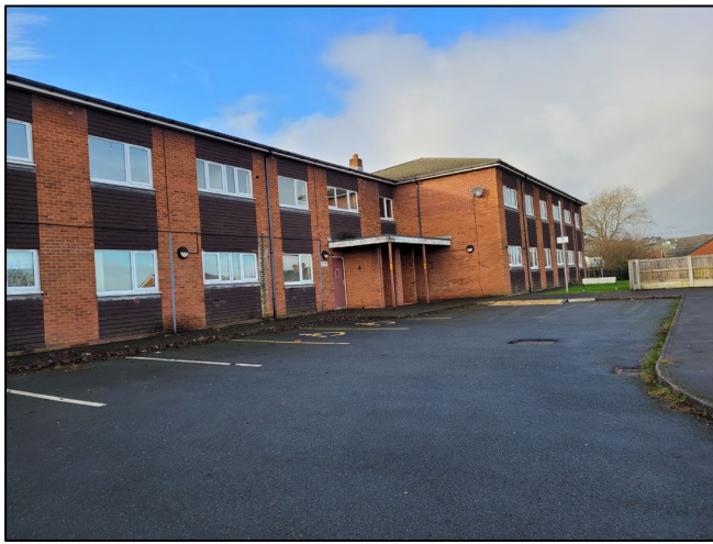
Photograph 1 The building and car park from the north of the site
