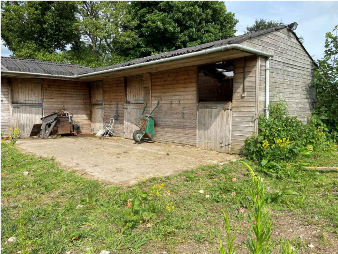
View 4 - View of existing stables to be utilised for bicycle storage.
