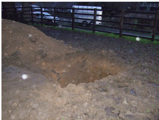
Percolation test pit
