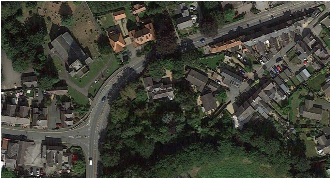
Current Aerial view
