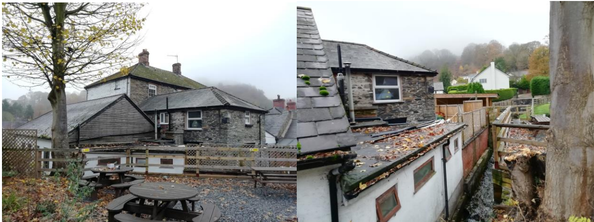
Fig. 4&5 – Rear Elevation / flat roof
