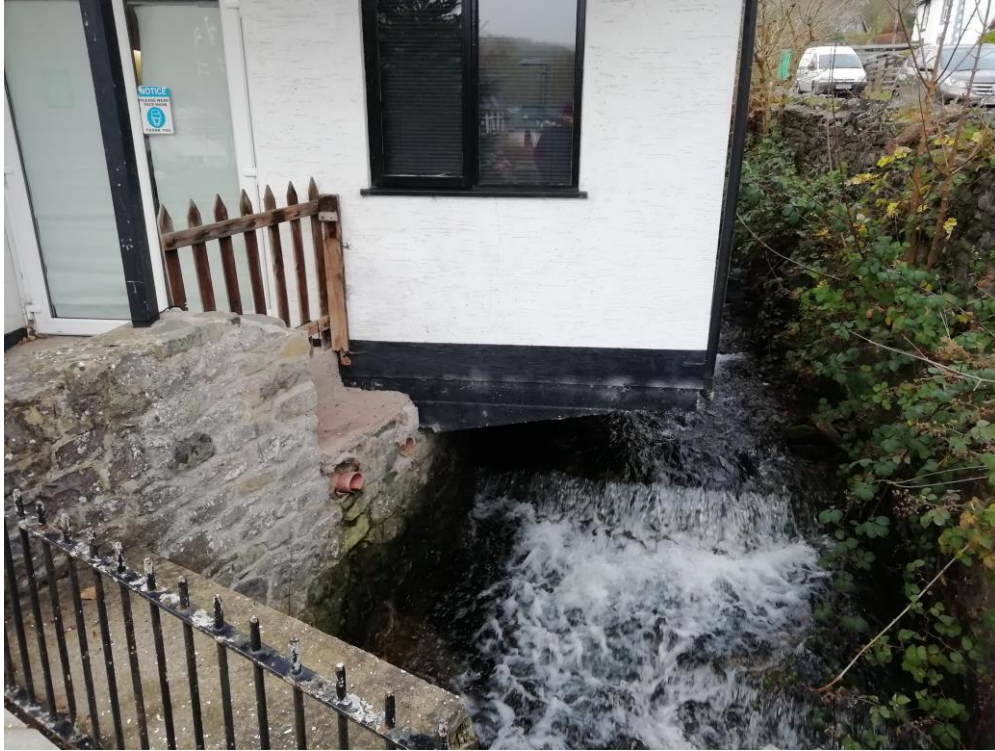
Fig. 3 – Cantilevered floor construction
