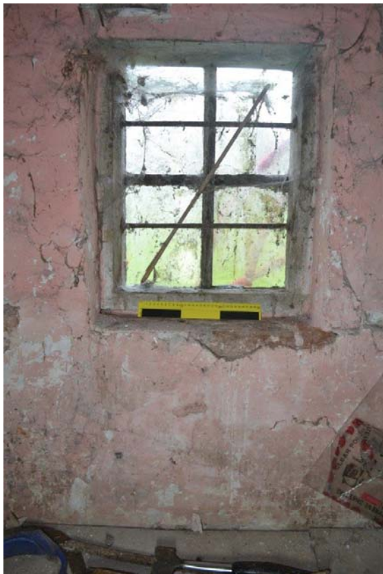
Plate 39: Ground floor, pantry. Window to rear elevation, timber frame, four lights, fixed. Security bars to inside. Scale = 30cm.
