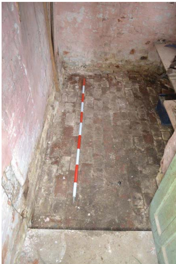
Plate 41: Ground floor, pantry. On-bed bricks forming sunken pantry floor. Scale =2m.
