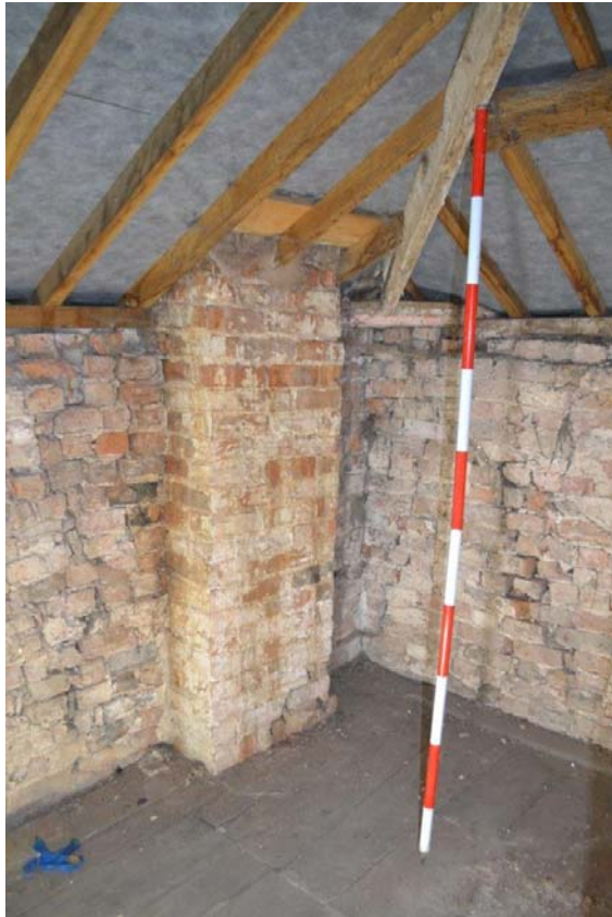
Plate 54: First Floor, Bedroom 3. Sightline to chimney. Also shows hip rafter, purlin and creeper rafters below the underfelt.
