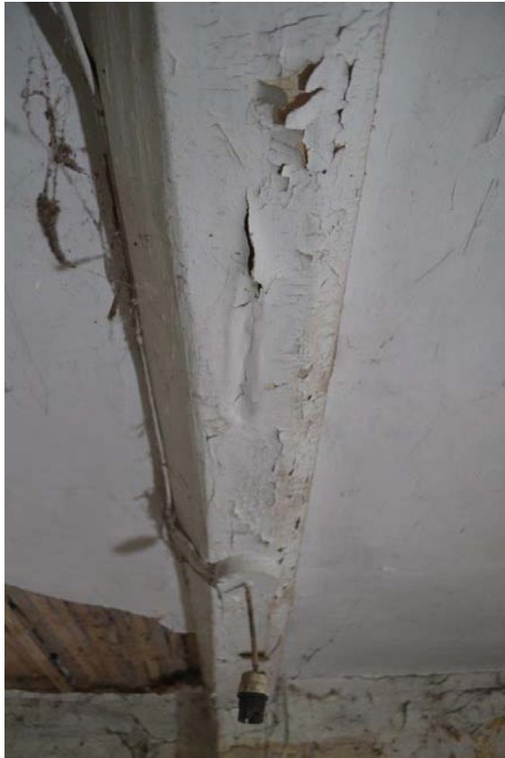
Plate 24: Ground Floor, Private Room. The bearer beam for the first floor joists.
