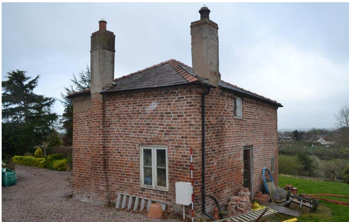
Plate 8: Oblique sightline to the south-west showing the east-facing and north-facing elevations. The chimneys betray the side-wall and rear-wall fireplace locations. The chimney to the east-facing elevation projects from the elevation face and punctures the roof at the eaves. It is rendered above eaves level and has a single, plain pot with mesh guard. There is a single, ground floor casement window to the east-facing elevation. The chimney to the north-facing elevation served the kitchen at ground floor level, projects from the elevation face and punctures the roof at the eaves. It is rendered above eaves level and has a single, plain pot with mesh guard. Scale =2m.
