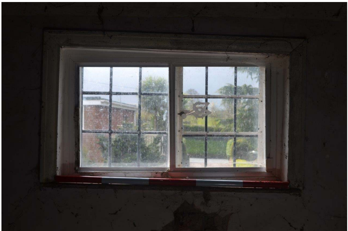
Plate 53: First Floor, Bedroom 2. Multi-paned casement window. Scale = 1m.
