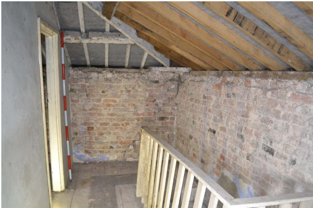
Plate 43: First Floor, Landing.
