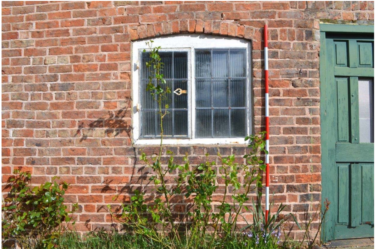
Plate 5: Sightline to the ground floor window serving the parlour, under a cambered, single-course, rowlock segmental arch head to the left of the entrance door. Window is a single, timber-frame casement, with lead comes dividing each light into 9 rectangular panes. Scale = 2m.
