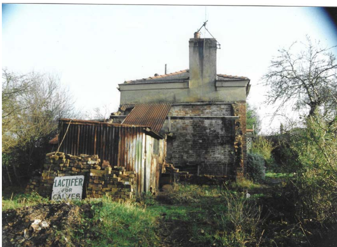
Applicant Images 3 and 4 (note S-shaped tie plate to the north-facing elevation of the lean-to on the west-elevation)
