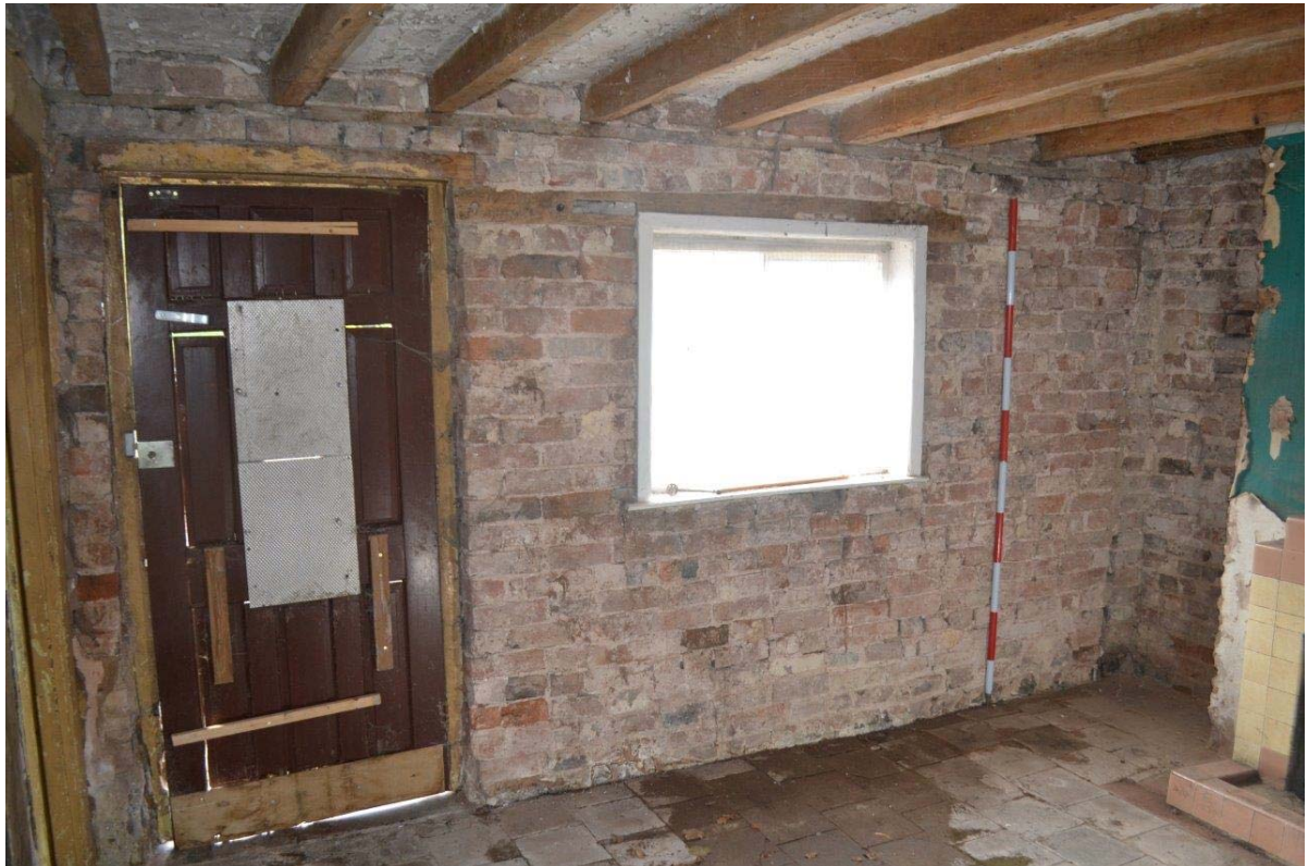
Plate 14: Ground Floor, Principal Living Room, looking towards the inner face of the brick wall forming the principal façade, the entrance door and the casement window. Scale = 2m
