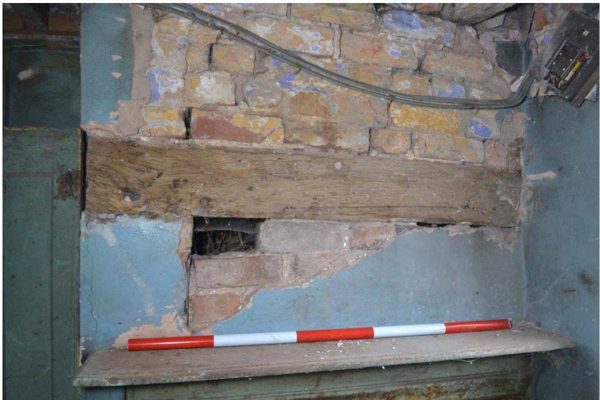
Plate 29: Ground Floor Kitchen. Detail of bressummer beam above cooking range. Scale = 1m.
