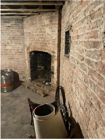
View of the ground floor front room.
