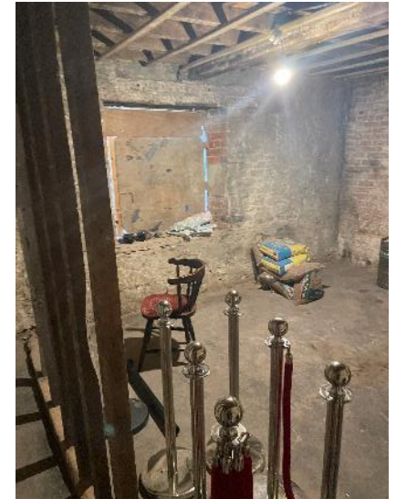
View of the ground floor front room
