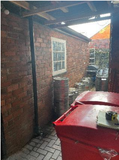
View of the window in the single storey rear block.
