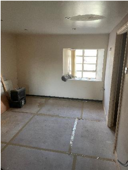
View of the first floor rear room.
