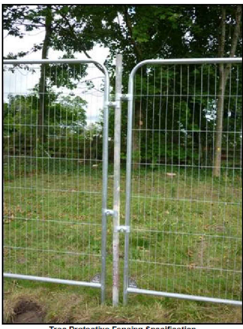
Tree Protective Fencing Specification
