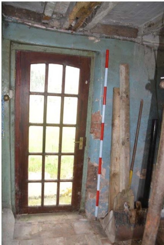
Plate 33: Ground Floor Kitchen. Sightline towards rear door. Scale = 2m.
