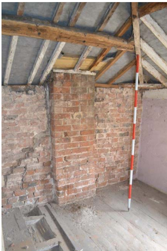
Plate 49: First Floor, Bedroom 2. Sightline to the chimney in the east-facing external wall. Also visible canted purlin, hip rafter and creeper rafters and underfelt. Scale = 2m.
