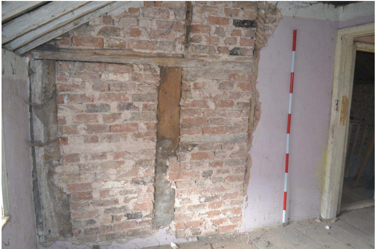
Plate 50: First Floor, Bedroom 2. Internal wall separating Bedroom 2 from Bedroom 1, highlighting the studs and rails with horizontal brick noggin. Scale = 2m.
