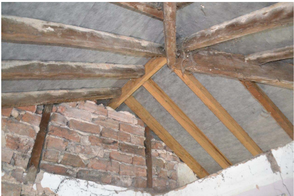
Plate 51: First Floor, Bedroom 2. Detail of roof truss construction showing replacement ridge beam, hip rafters, common rafters and reused rafters with underfelt above.
