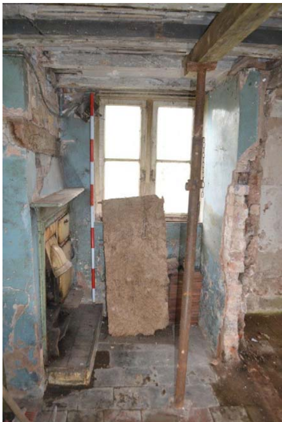
Plate 27: Ground Floor Kitchen, showing the casement window to the east0facing elevation and the cooking range to the left. Scale = 2m.
