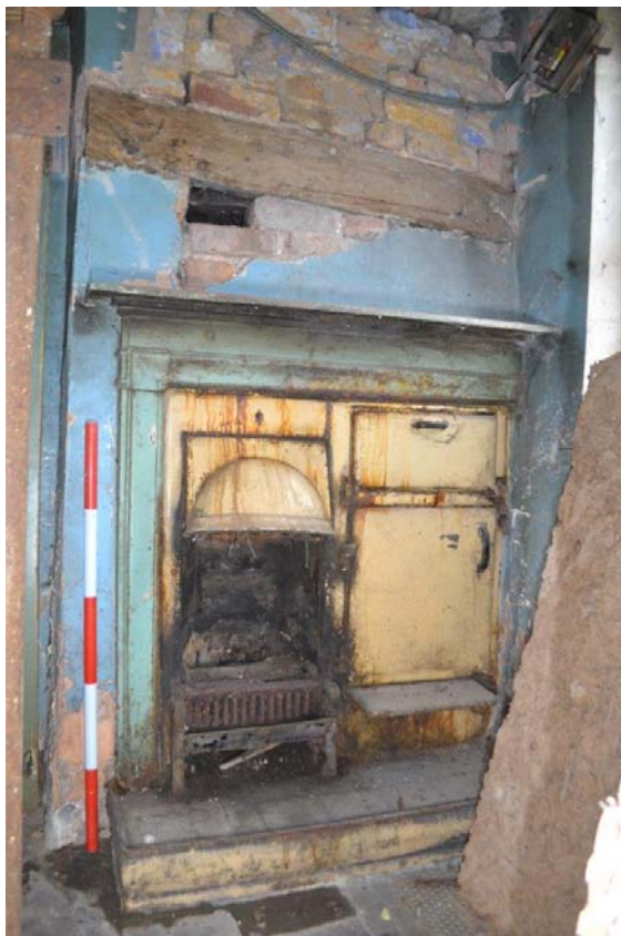
Plate 31: Ground Floor Kitchen. Detail of early/mid-20 th century fire/cooking range. Scale = 1m.
