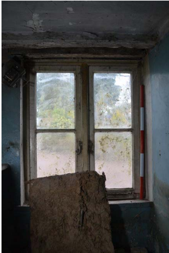
Plate 30: Ground Floor Kitchen. Detail of timber, four-light double casement window with monkey-tail handles. Scale = 1m.
