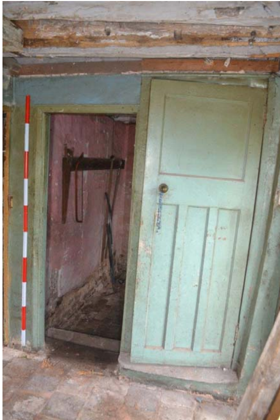
Plate 32: Ground Floor Kitchen, looking towards the pantry and the door to the staircase to the first floor. Scale = 2m.
