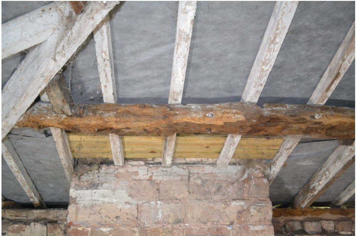
Plate 46: First Floor Bedroom 1. Detail of chimney breast exit point through roof with waney purlin, hip rafter, replacement/reused machine-sawn creeper rafters and underfelt.
