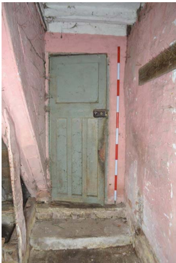
Plate 40: Ground floor, pantry. Looking back up the stone steps to the timber door into the through passage. Underside of staircase to first floor to left. Scale = 2m.
