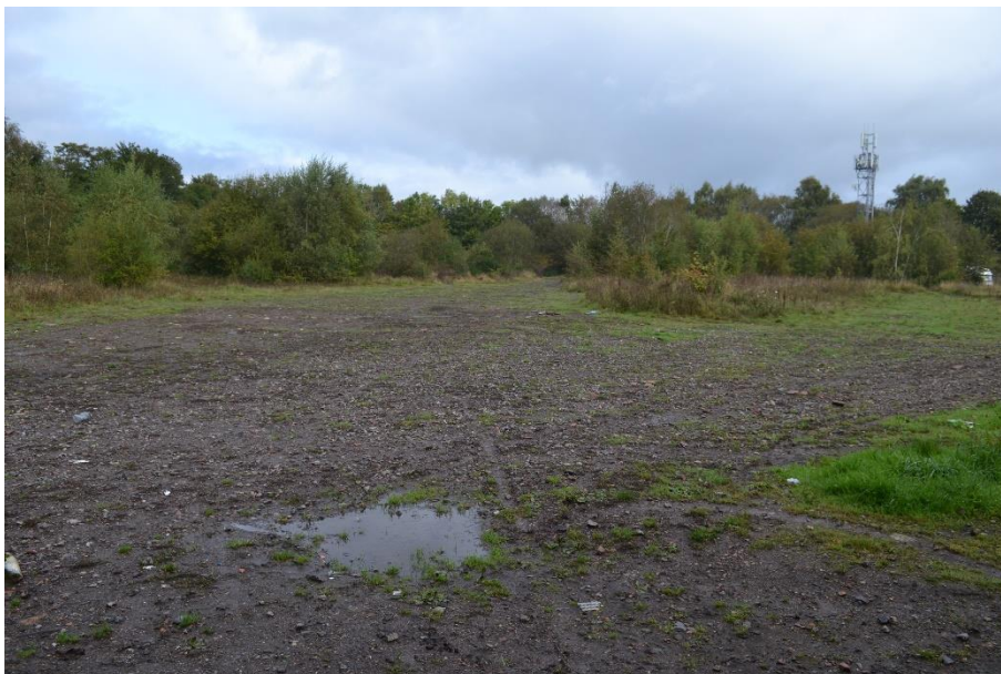
Figure 4.1 Overview of site
