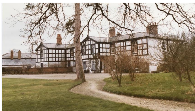
Photograph showing north elevation, circa 1970's
