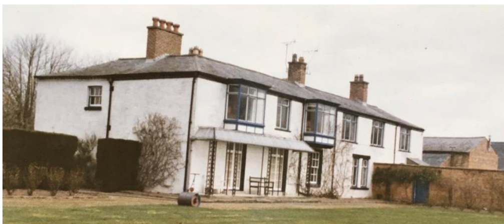
Photograph showing south elevation, circa 1970's
