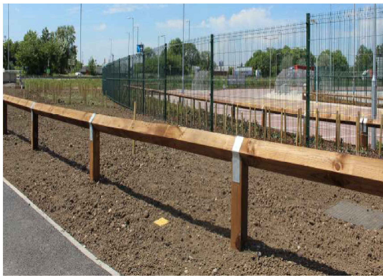
Insert 1 Proposed Lockable Timber Knee Rail Fence.
