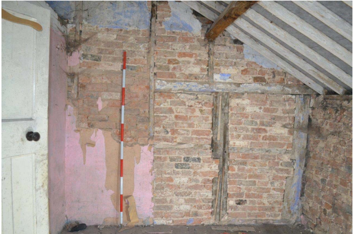
Plate 44: First Floor Bedroom 1. Internal wall separating Bedroom 1 from Bedroom 2, highlighting the studs and rails with horizontal brick noggin. Also visible a canted purlin above which are replacement/reused machine-sawn common rafters
