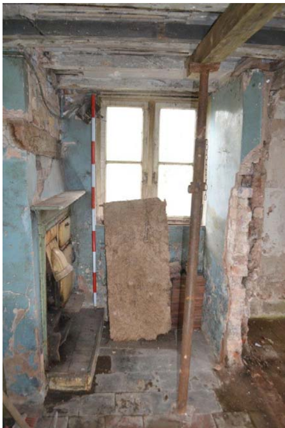
Plate 27: Ground Floor Kitchen, showing the casement window to the east-facing elevation and the cooking range to the left. Scale = 2m.
