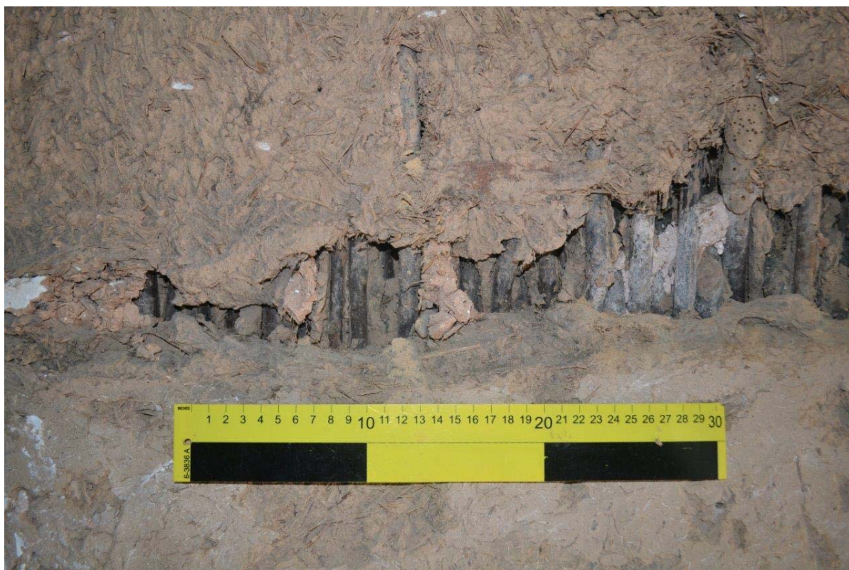
Plate 20: Ground Floor, Principal Living Room. Detail of the wattle and daub panel in the internal wall separating the principal living room from the private room. It's not strictly wattle as there are no visible vertical staves and the wattles (possibly hazel) are not woven horizontally- they are closely packed and vertically arranged. Scale = 30cm
