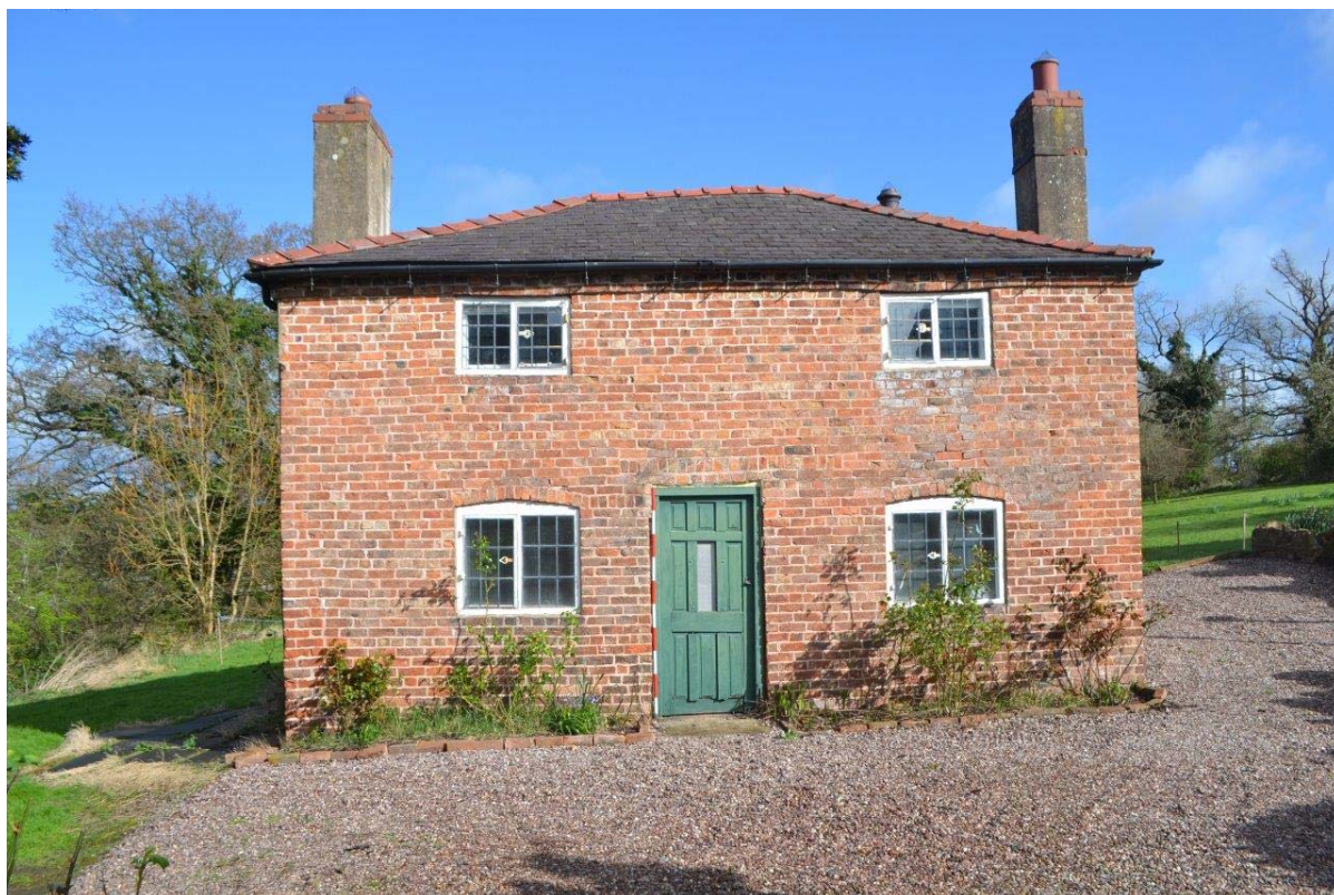
Plate 3: Sightline to the south-facing, entrance façade highlighting the central entrance door, hipped roof, chimneys and the asymmetric fenestration to ground and first floors. Brickwork is in the Raking English Garden Wall Bond. Scale = 2m.
