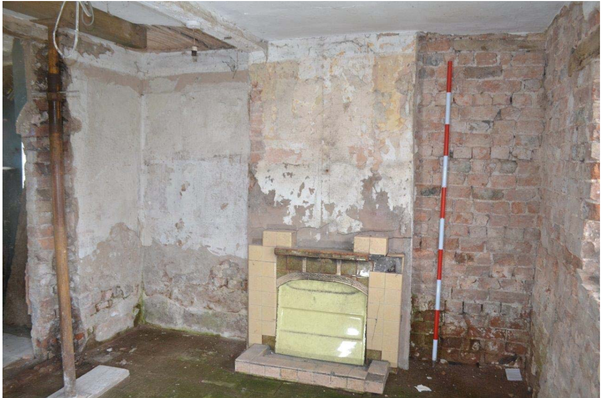
Plate 22: Ground Floor, Private Room. Chimney breast and mid-20 th century fireplace. Scale = 2m
