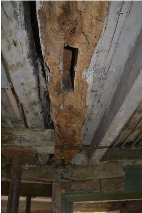
Plate 36: Ground Floor Kitchen. Mortice in waney bearer beam tying the internal wall separating the kitchen from the private room into the rear wall.
