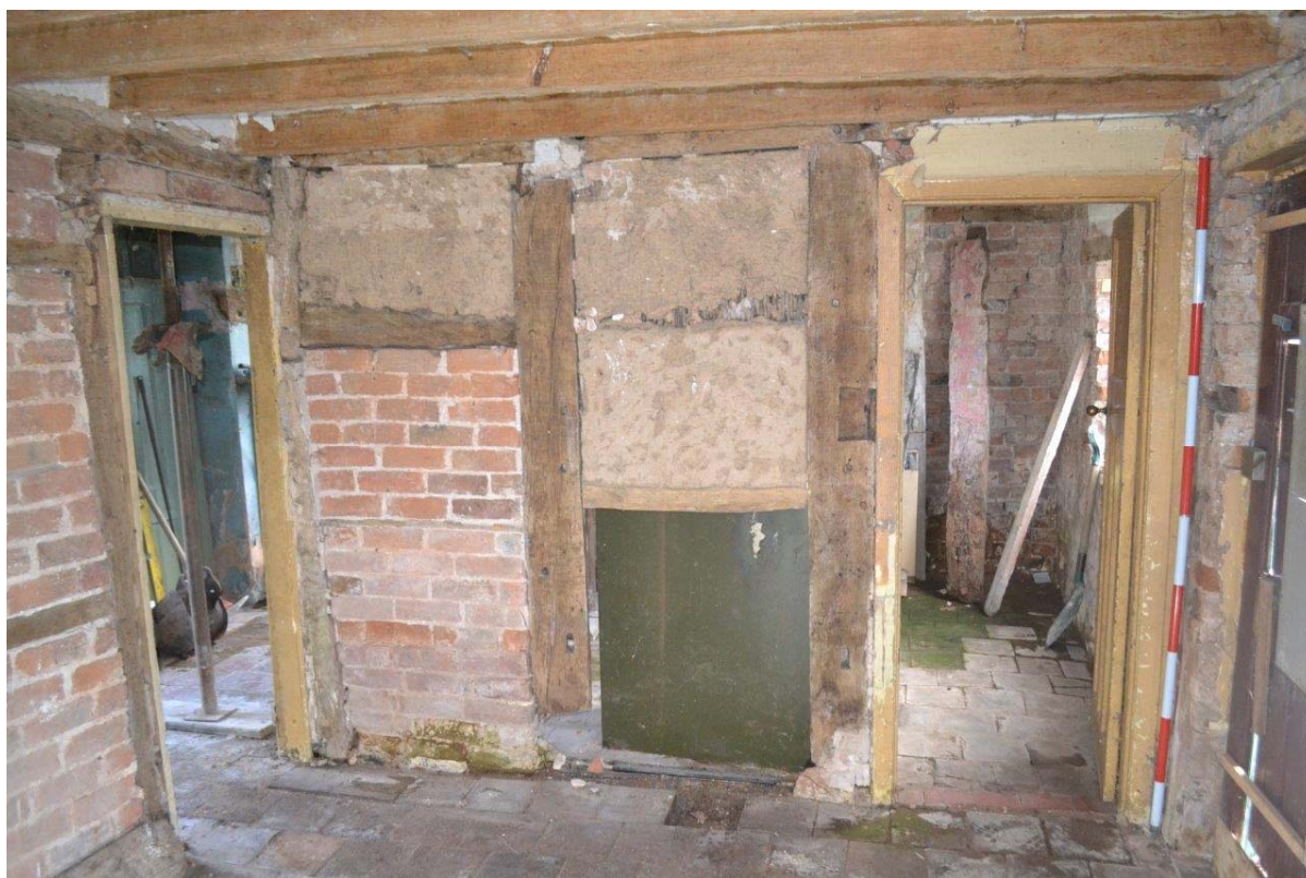
Plate 16: Ground Floor, Principal Living Room. The internal wall separating the principal living room from the private room. Constructed from timber studs and rails with infilling brick nogging and also two panels of wattle and daub. Scale = 2m
