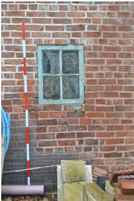
Plate 12: Sightline to the south highlighting the four-light fixed window in the north-facing (rear) elevation, serving the pantry. Scale =2m.
