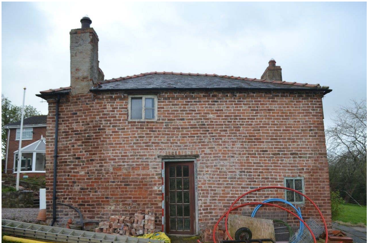
Plate 10: Sightline to the south showing the north-facing (rear) elevation highlighting the kitchen chimney, the off-set rear door and fenestration to the ground and first floors. Scale -=2m.
