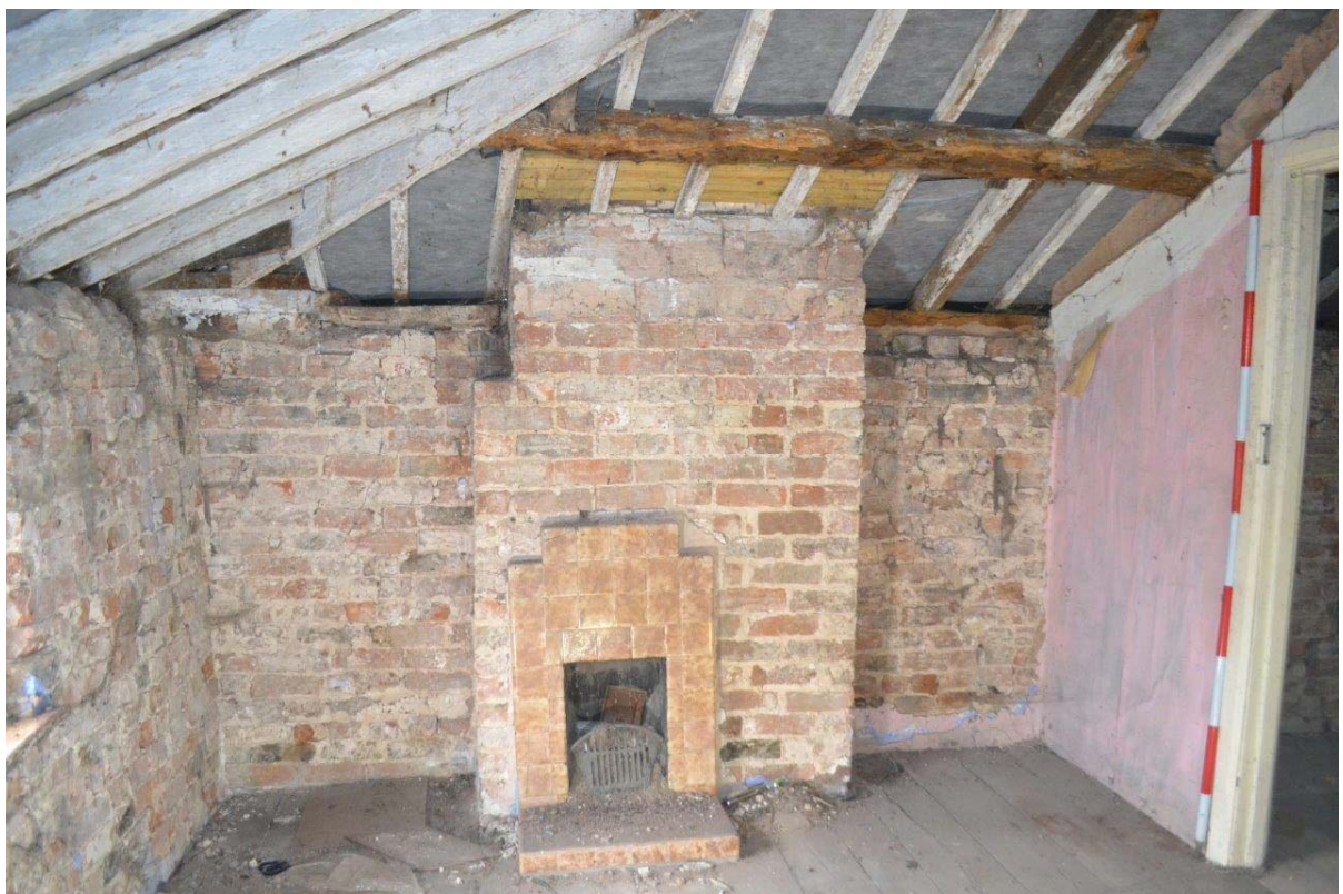
Plate 45: First Floor Bedroom 1. Chimney breast and off-centre mid-20 th century fireplace backing onto west-facing elevation wall. Also visible a canted purlin to the hip rafter and the above which are replacement/reused machine-sawn creeper rafters and underfelt.
