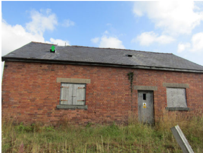
Photo 4: Brandt's bat emerged from beneath ridge tile near West gable-end (green arrow).
