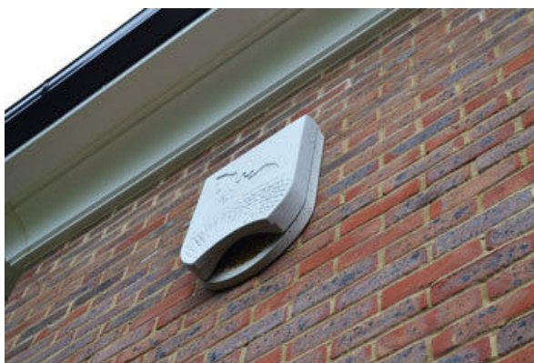
Figure 14: Schwegler (1WQ) bat box fitted to wall.
