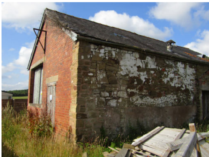
Photo 6: North elevation and East gable-end.
