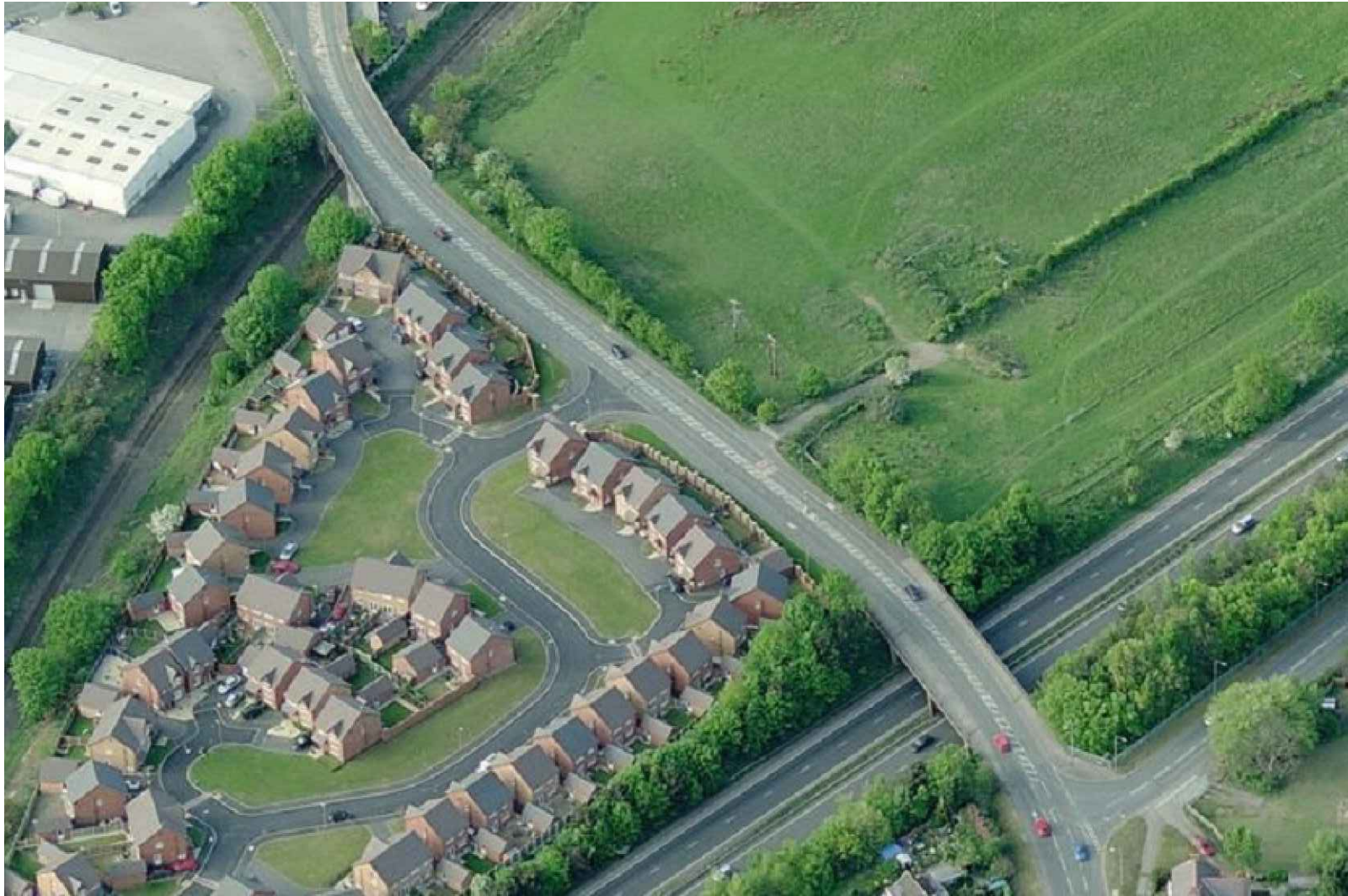
NORTH SOUTH AERIAL VIEW
