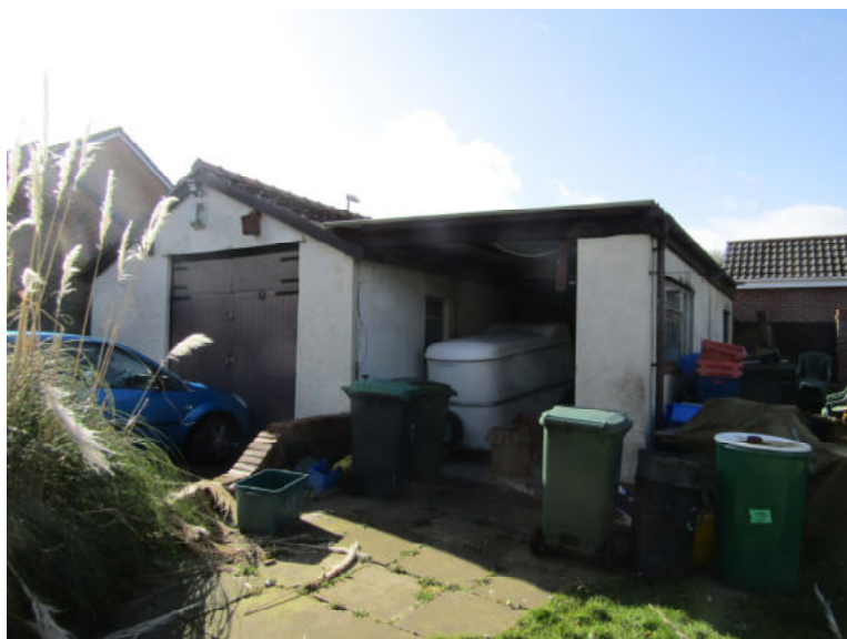
Garage and workshop.
