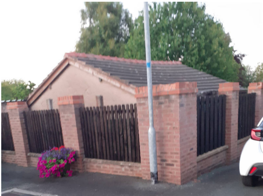
Photo 2: Rear (West) elevation of garage and adjoining workshop.
