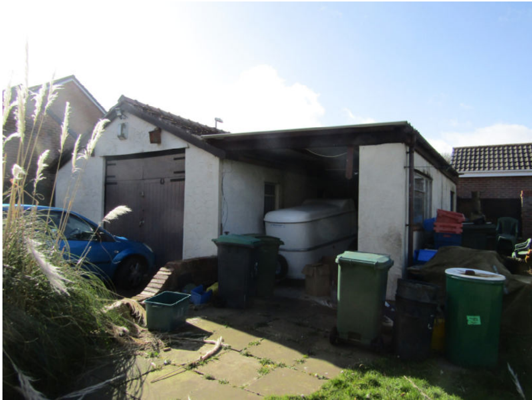
Photo 1: Front (East) elevation of garage and adjoining workshop.
