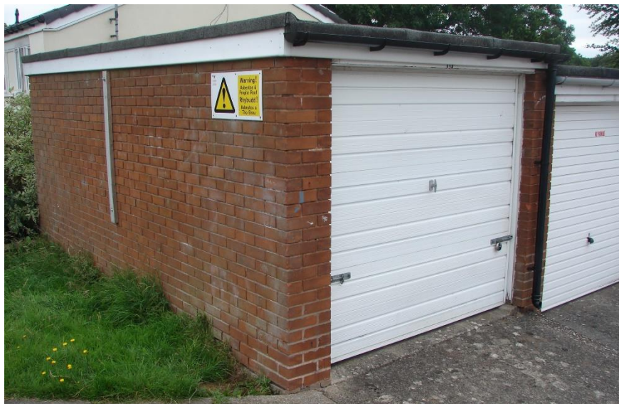
Garage Unit 10, Target Note 5 .
