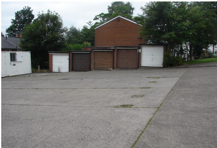
View towards the garages at Target Note 6 .
