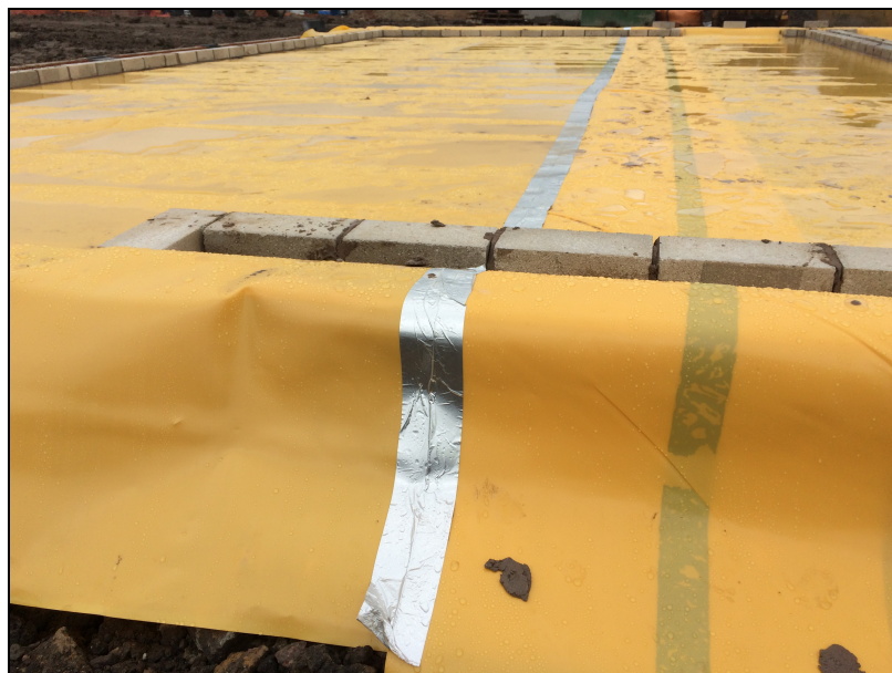
Photographs 11 and 12: Check >150mm overlaps of membranes and proprietary tapes placed and sealed with photographs taken. Note membrane shown is not specific for radon protection on this site and is only used as an example.
