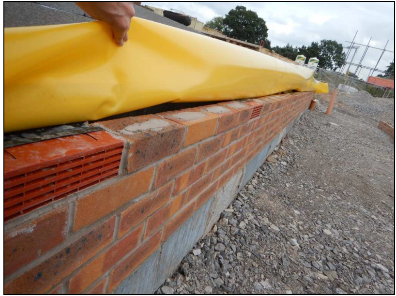
Photographs 8 and 9: Verify presence of cranked vents along the external walls and sufficient spacing. Areas of access points to internal garages or external adjoining garages may not be possible to have cranked venting and alternative construction options should be discussed where necessary. Note membrane shown is not specific for radon protection on this site and is only used as an example.
