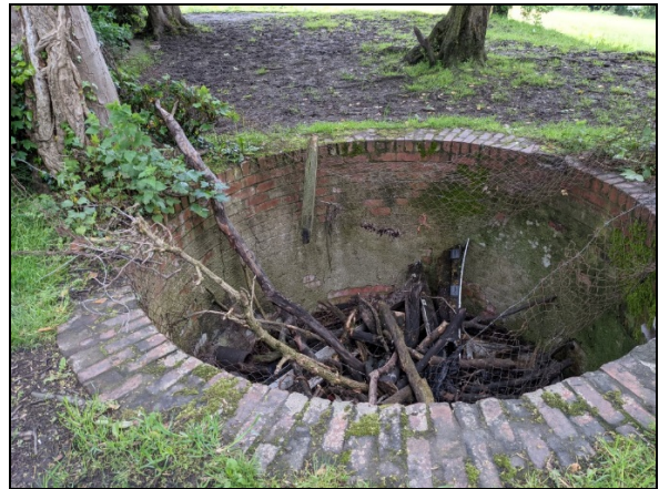
Photograph 4: Showing the smaller circular brick structure adjacent to the infilled reservoir
