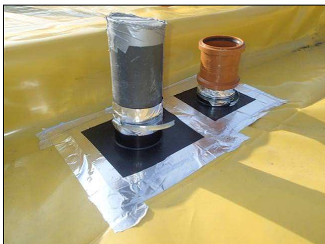
Photographs 13 and 14: Check tophat is sealed to membrane and pipework with tapes, and Jubilee clip. Note membrane shown is not specific for radon protection on this site and is only used as an example.
