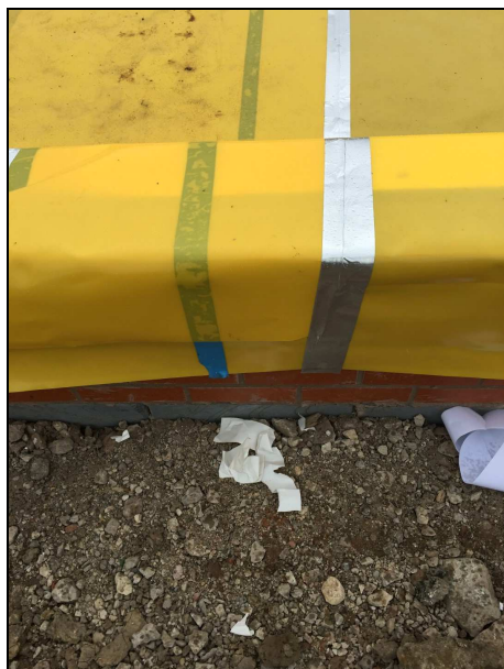
Photographs 11 and 12: Check >150mm overlaps of membranes and proprietary tapes placed and sealed with photographs taken. Note membrane shown is not specific for radon protection on this site and is only used as an example.
