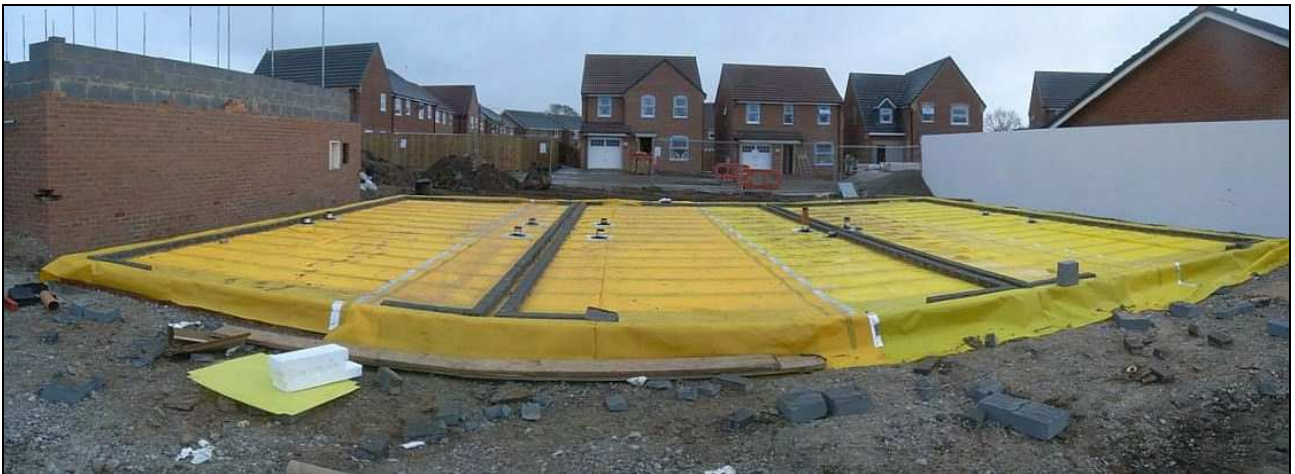
Photograph 10: Check general condition of membrane for punctures/tears etc – take panoramic photograph showing general condition. Note membrane shown is not specific for radon protection on this site and is only used as an example.
