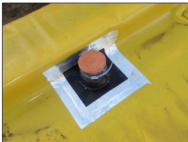
Photographs 13 and 14: Check tophat is sealed to membrane and pipework with tapes, and Jubilee clip. Note membrane shown is not specific for radon protection on this site and is only used as an example.
