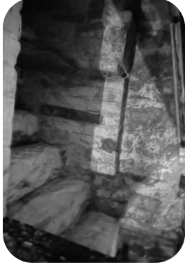
Underneath of original cellar stairs (blocked off)
