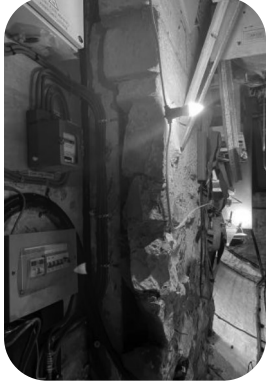
Original cellar access, now blocked off
