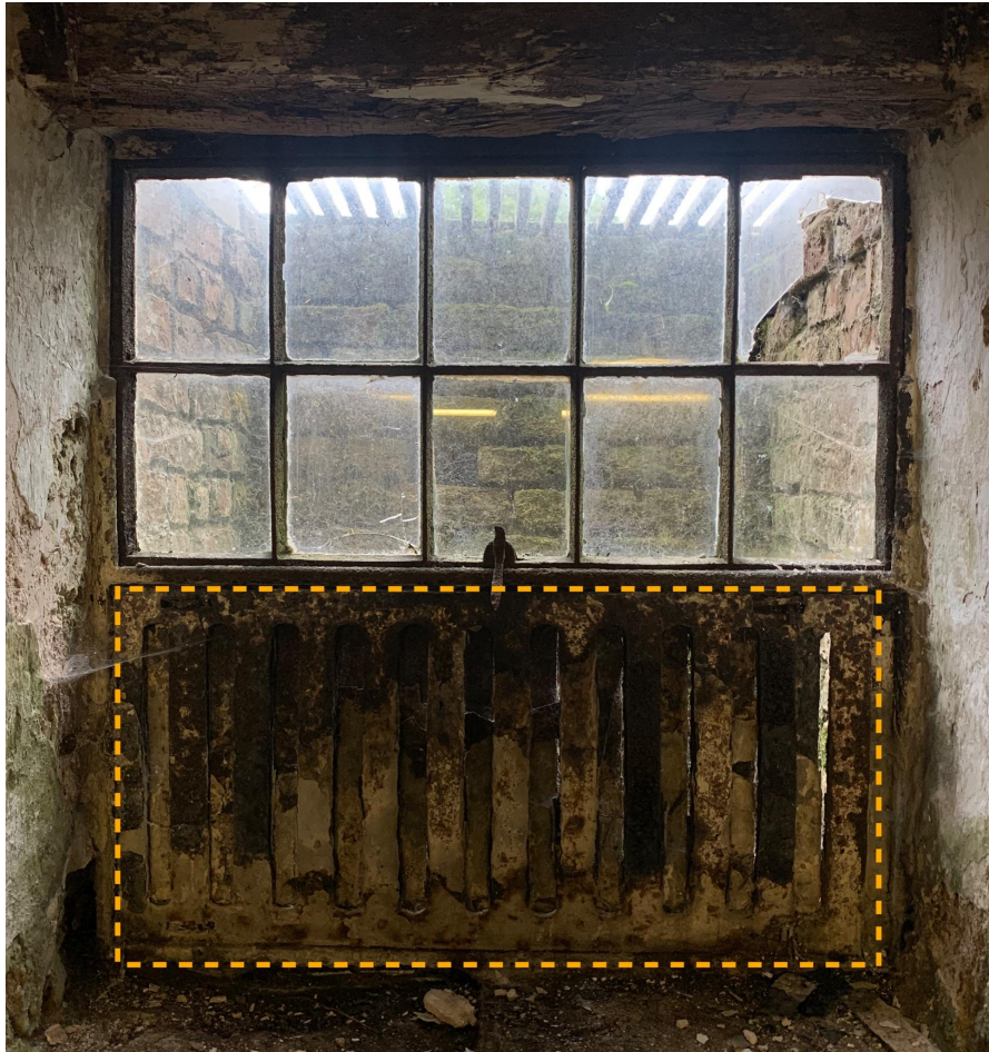
Figure 8 - Existing condition of small-paned iron framed window in cellar
