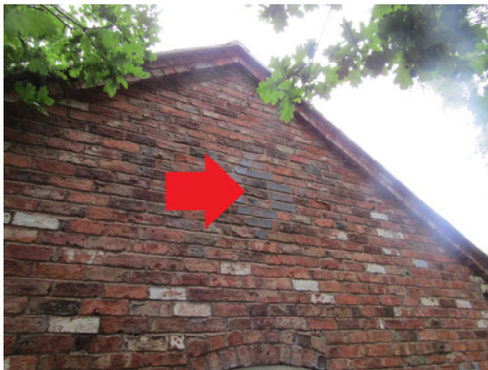
Photo 3: Removing 1 or 2 bricks from the East gable-end wall could create an open 'fly-in' access for void-dwelling bat species.
