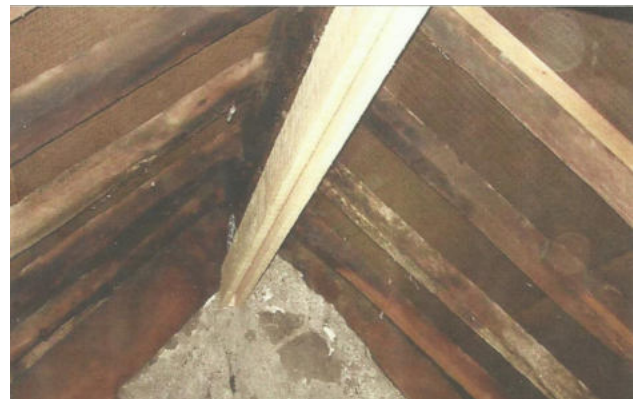
Figure 5: Crevice box in loft void.
