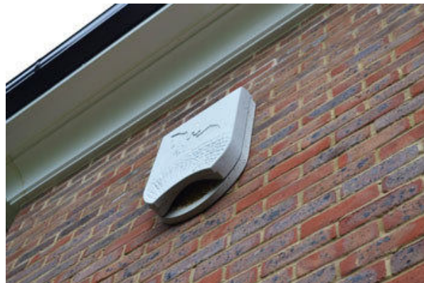
Figure 3: Schwegler (1WQ) bat box fitted to wall.
