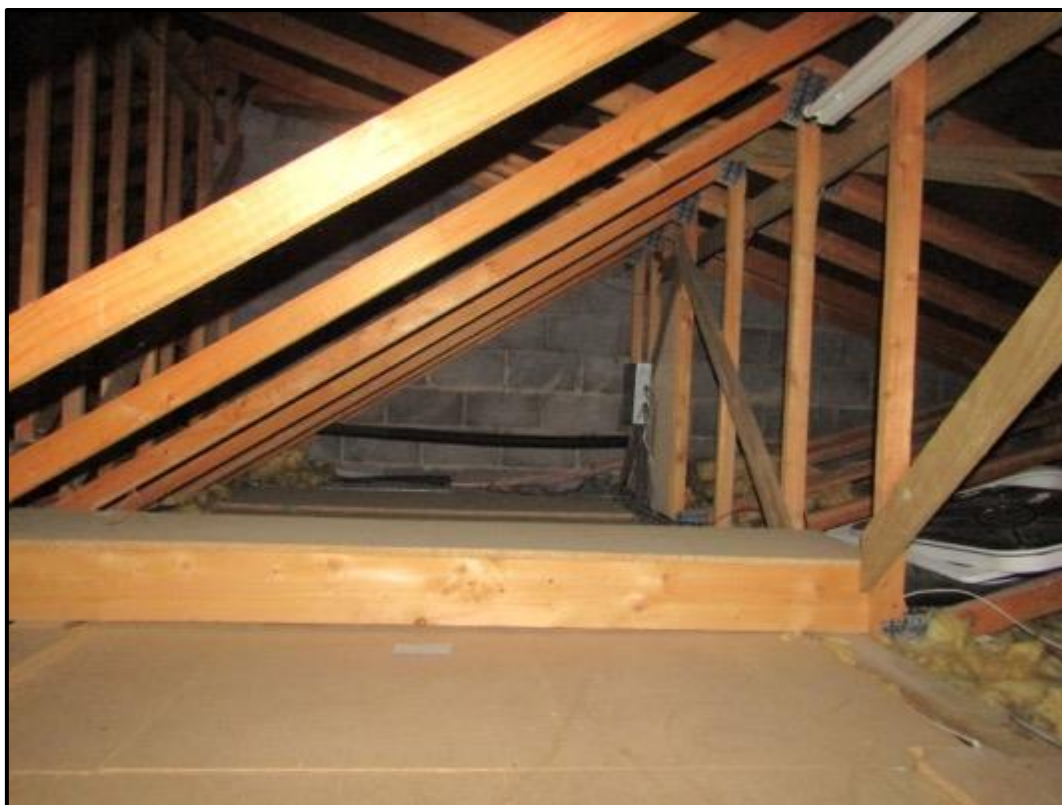
Fig 10: The roof void is configured into a complex A frame support structure.
