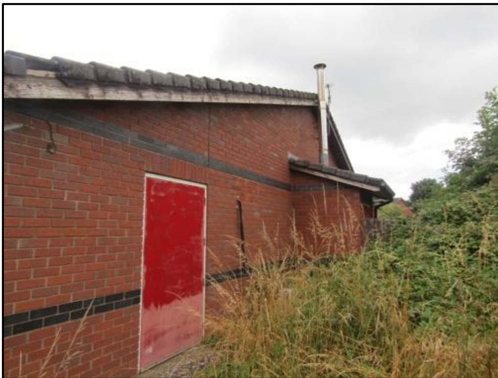
Fig 6: The side gable is well sealed; the wooden fascia board is weathered but well sealed. Also, the overlapping tiles are fitted tightly against the board.
