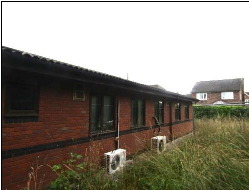
Fig 5: The rear elevation is in good condition; the yard/garden area is dominated by commoner succession grasses and weeds. No invasive species were noted.
