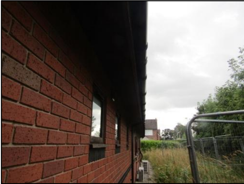
Fig 4: The fascia boards and soffits are all in good condition sealed to the exterior walls.
