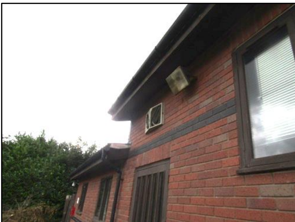
Fig 7: The frontage is also well sealed; the fascias are well sealed against the external wall and the roof.
