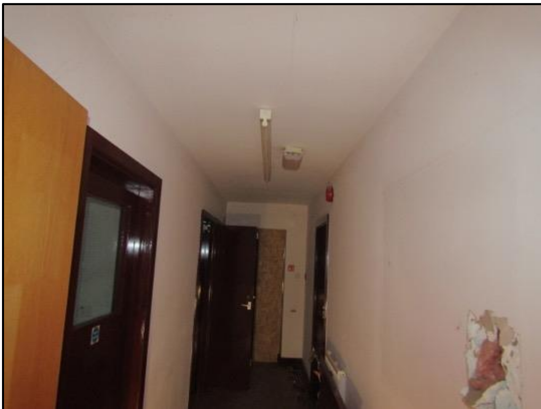
Fig 9: The remainder of the building is configured into corridors and small rooms; no signs of bats or birds were noted.
