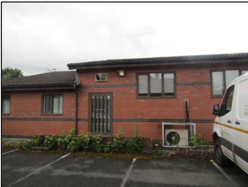
Fig 2: The target building, showing the front elevation. The building is circ <20 years old and in very good condition.
