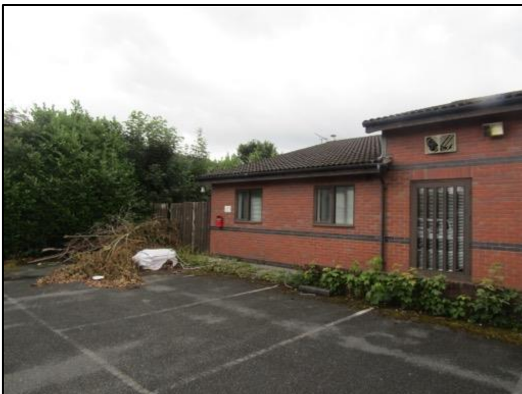
Fig 3: The building is set on hard standing and bounded by laurel, privet hedges.
