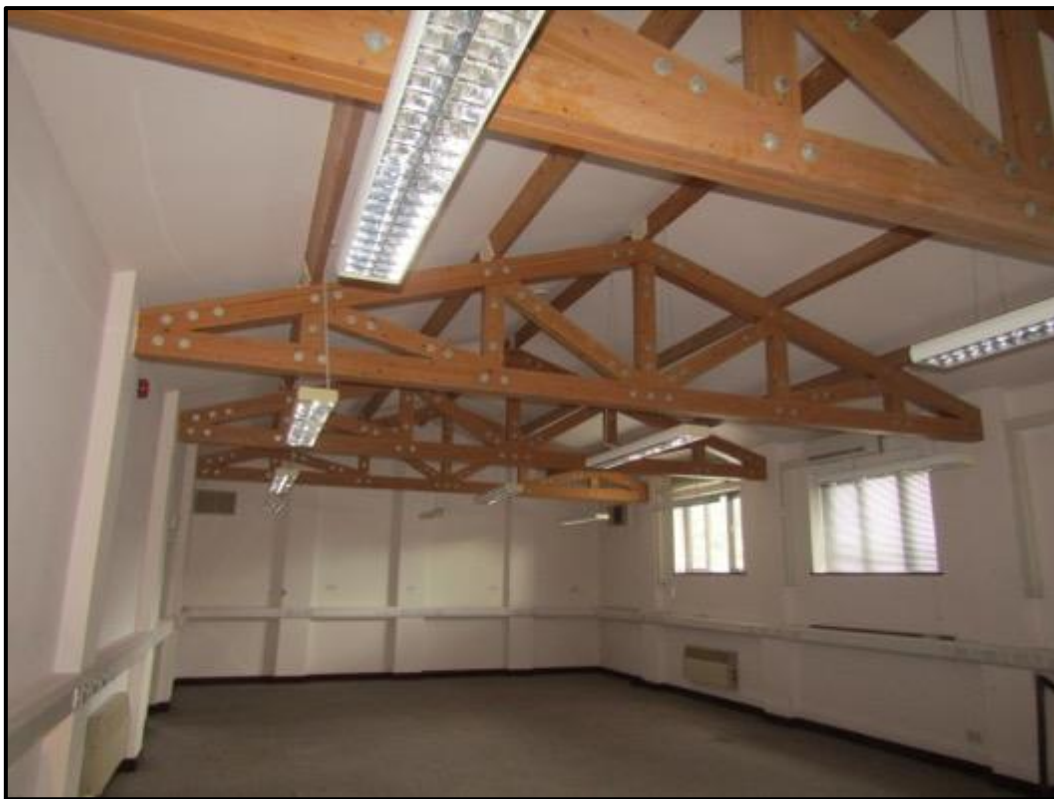
Fig 8: The ground floor is configured into an open assembly hall.
