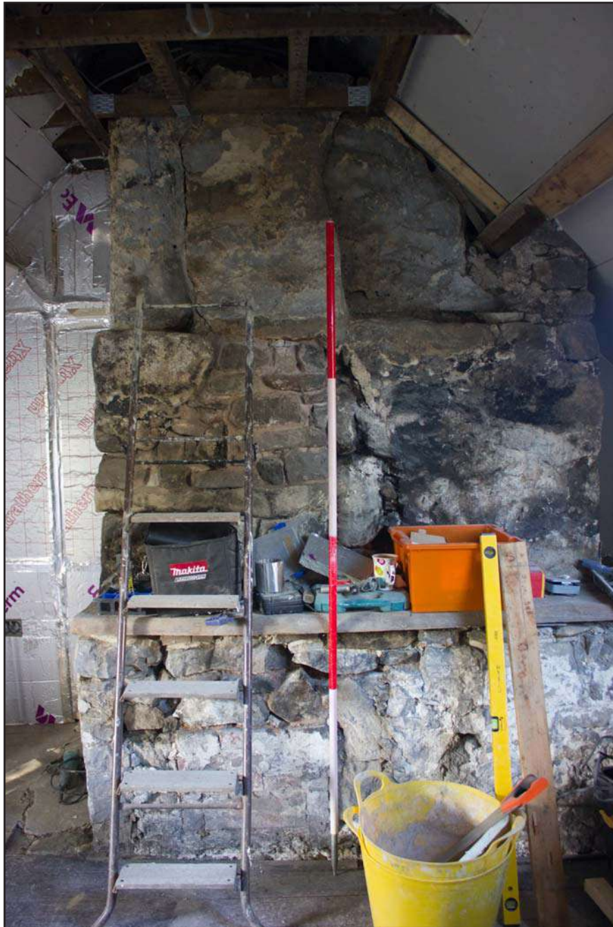
Plate 18: Internal shot of chimney breast within the first floor room at Brookside Cottage, Trevor Hall Road, Garth, Llangollen, Wrexham - from the east - 2.00m scale
