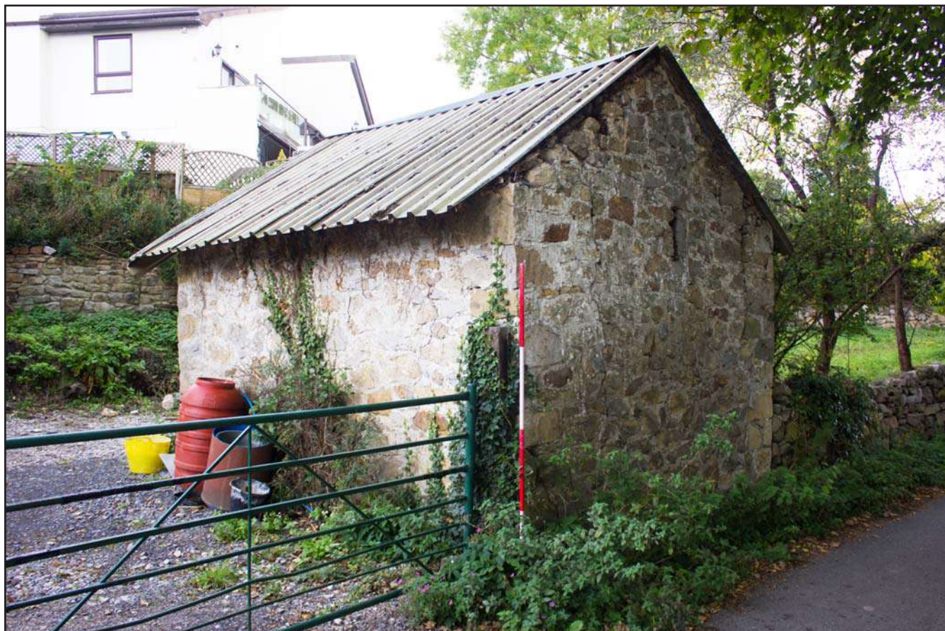
Plate 21: External shot of outbuilding at Brookside Cottage, Trevor Hall Road, Garth, Llangollen, Wrexham - from the south - 2.00m scale
