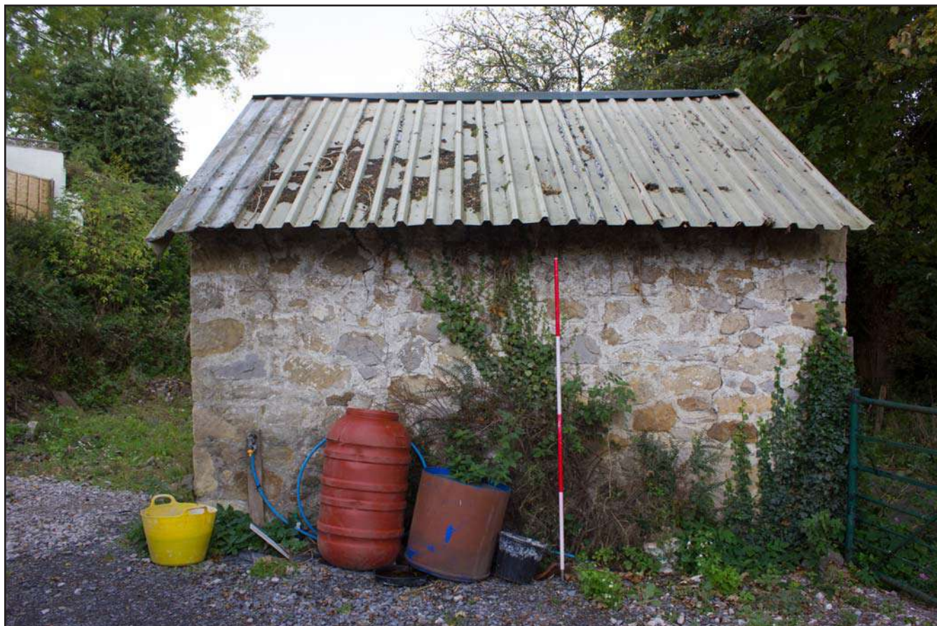
Plate 22: External shot of outbuilding at Brookside Cottage, Trevor Hall Road, Garth, Llangollen, Wrexham - from the southwest - 2.00m scale
