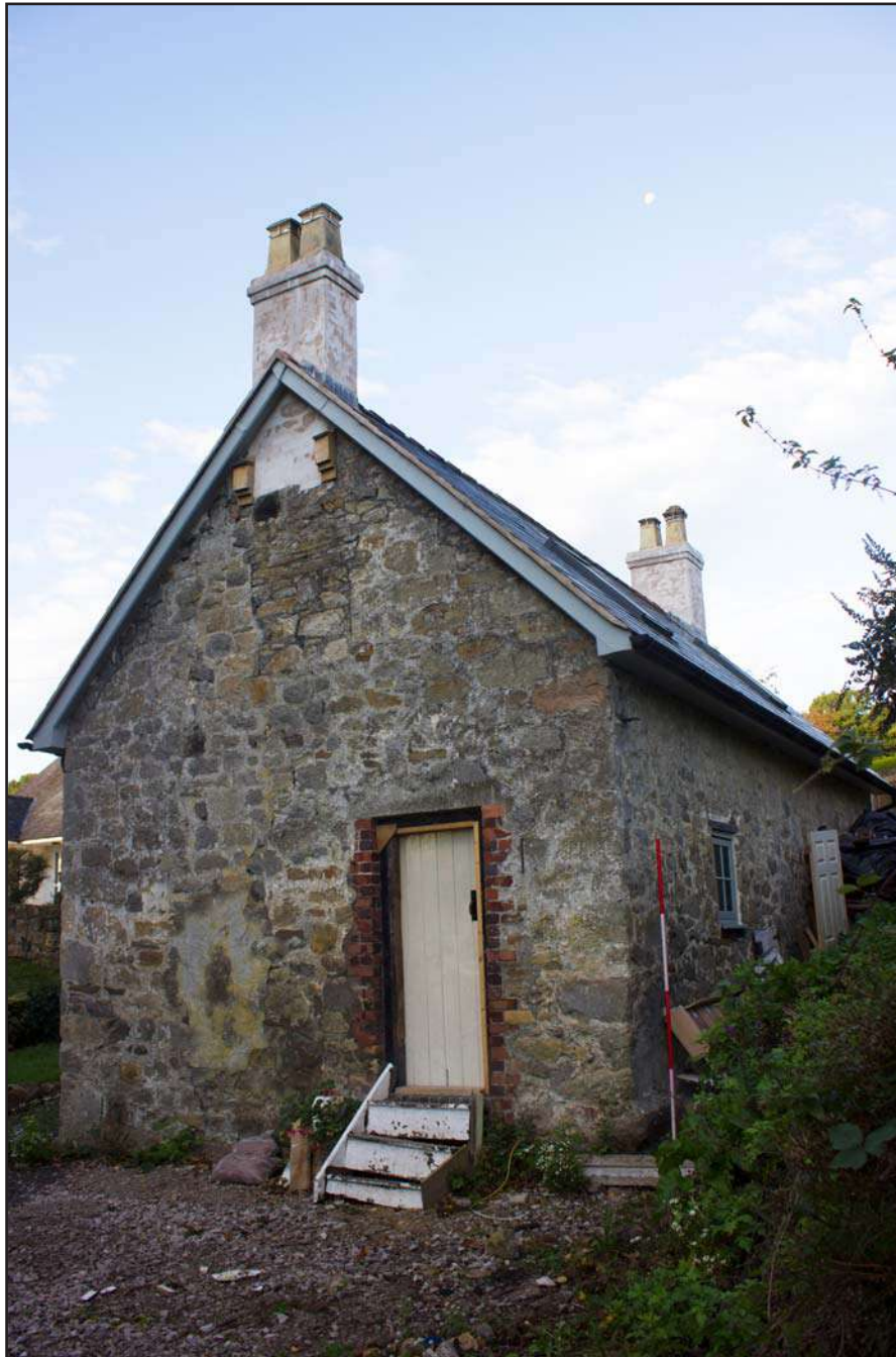
Plate 07: Oblique shot of eastern and northern elevations of Brookside Cottage, Trevor Hall Road, Garth, Llangollen, Wrexham - from the southeast - 2.00m scale
