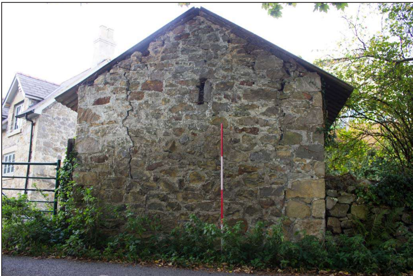
Plate 20: External shot of outbuilding at Brookside Cottage, Trevor Hall Road, Garth, Llangollen, Wrexham - from the southeast - 2.00m scale
