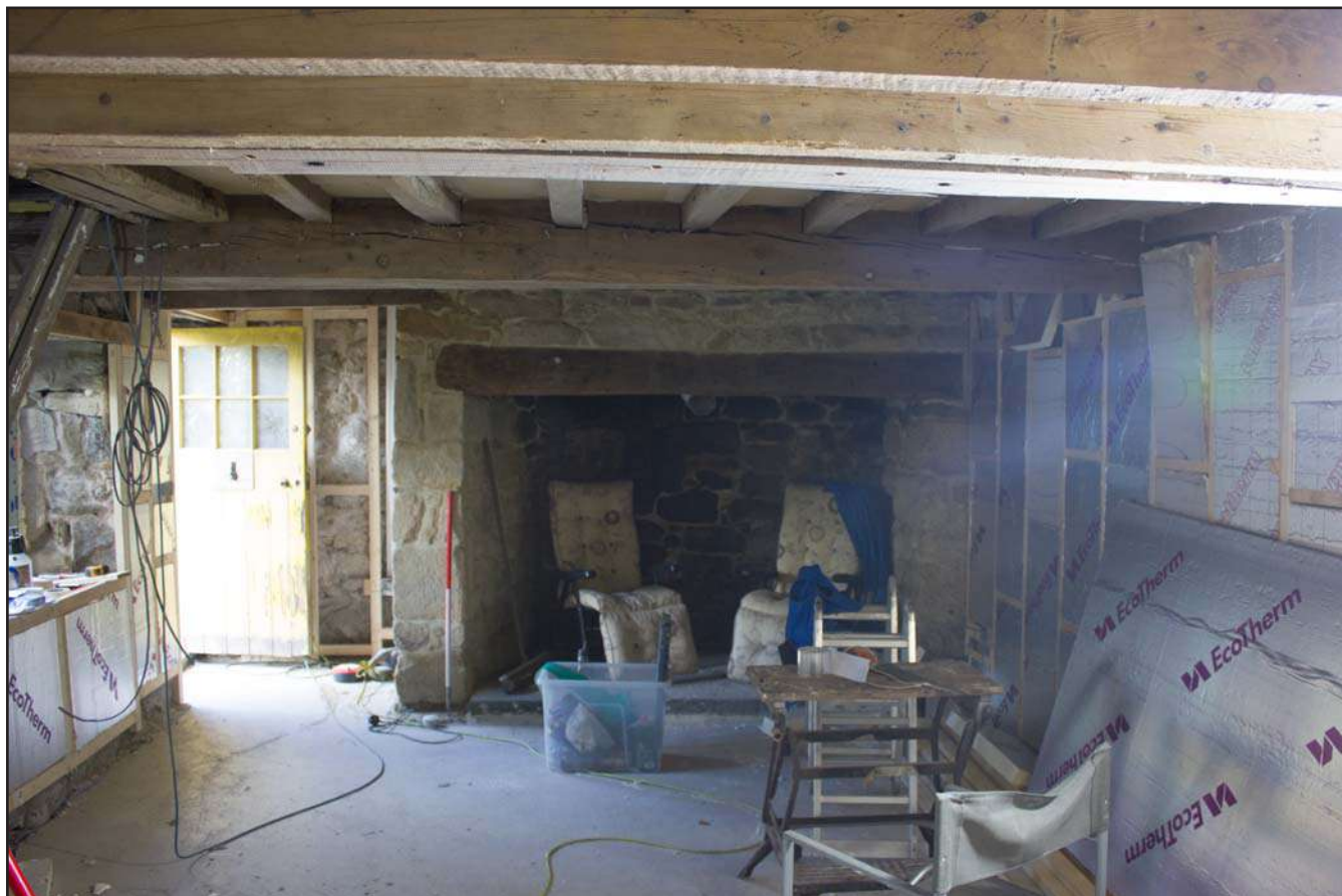
Plate 14: Internal shot of ground floor room within Brookside Cottage, Trevor Hall Road, Garth, Llangollen, Wrexham - from the east - 1.00m scale
