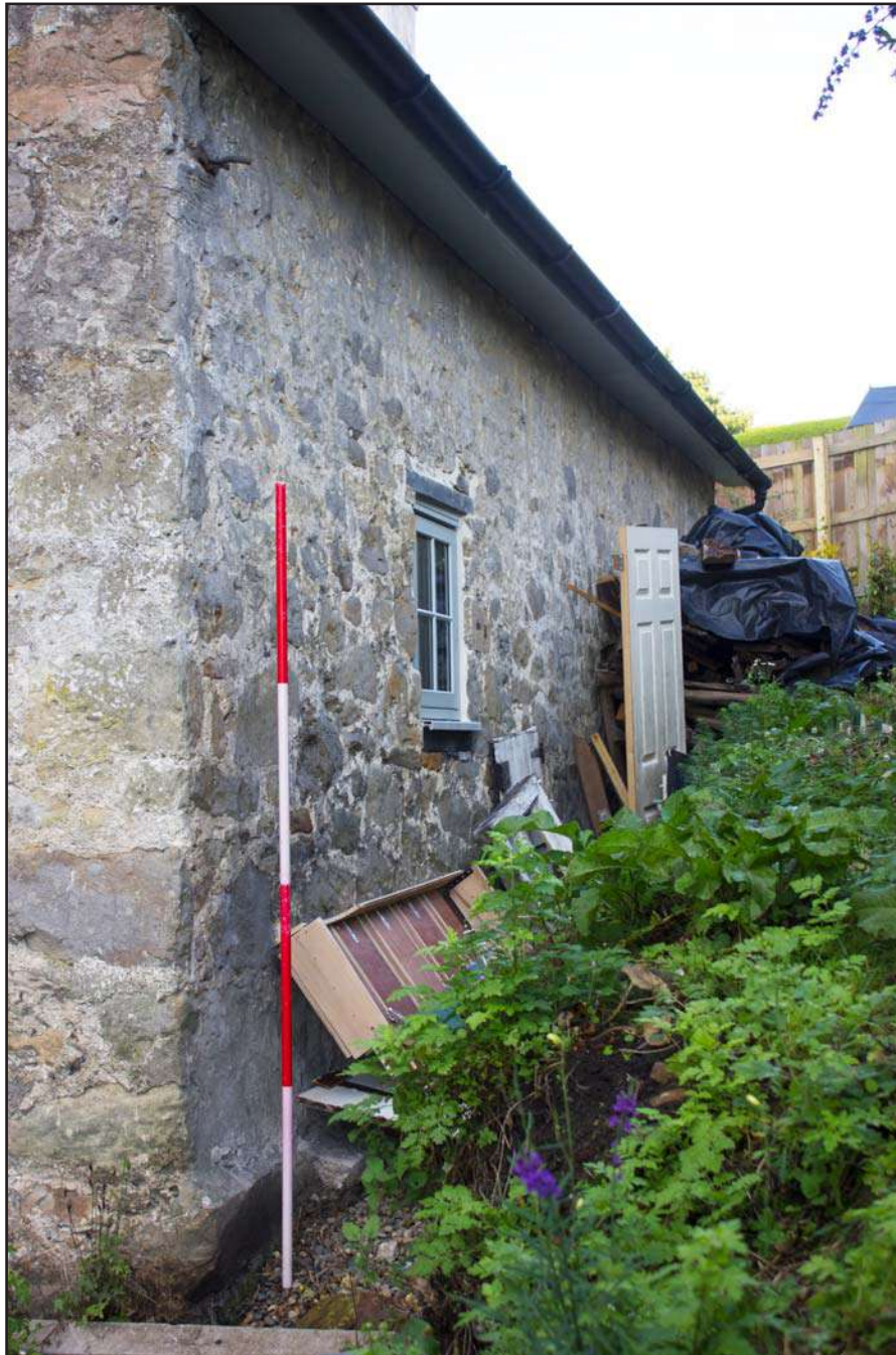
Plate 08: Northern elevation (oblique) of Brookside Cottage, Trevor Hall Road, Garth, Llangollen, Wrexham - from the east/northeast - 2.00m scale
