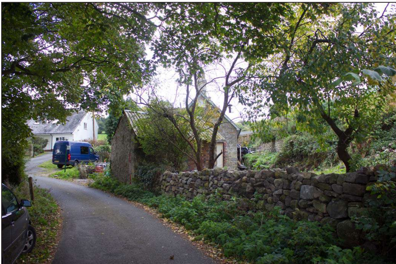
Plate 02: Context shot of Brookside Cottage, Trevor Hall Road, Garth, Llangollen, Wrexham - from the southeast - 2.00m scale
