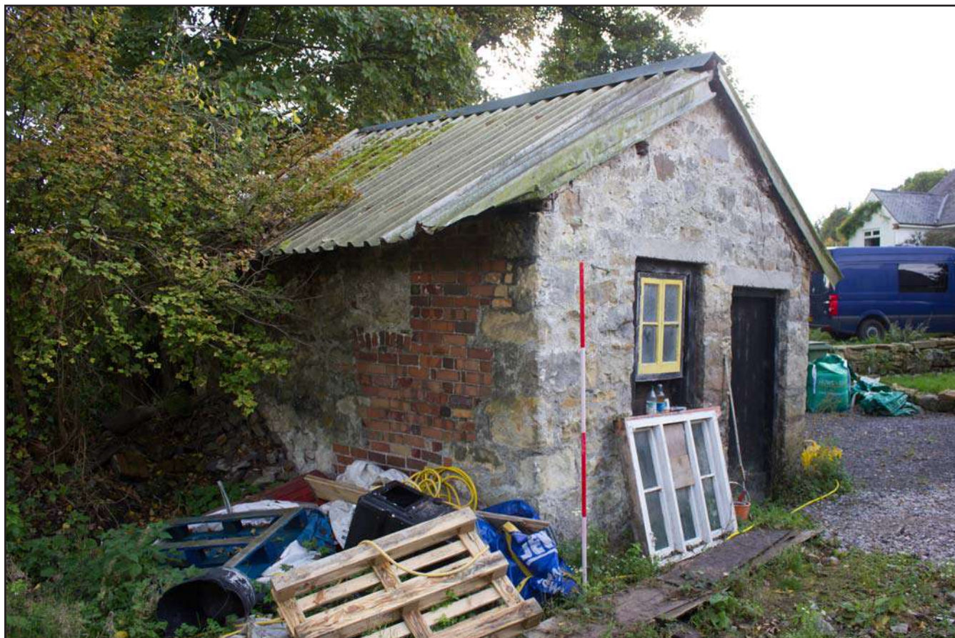
Plate 25: External shot of outbuilding at Brookside Cottage, Trevor Hall Road, Garth, Llangollen, Wrexham - from the north - 2.00m scale
