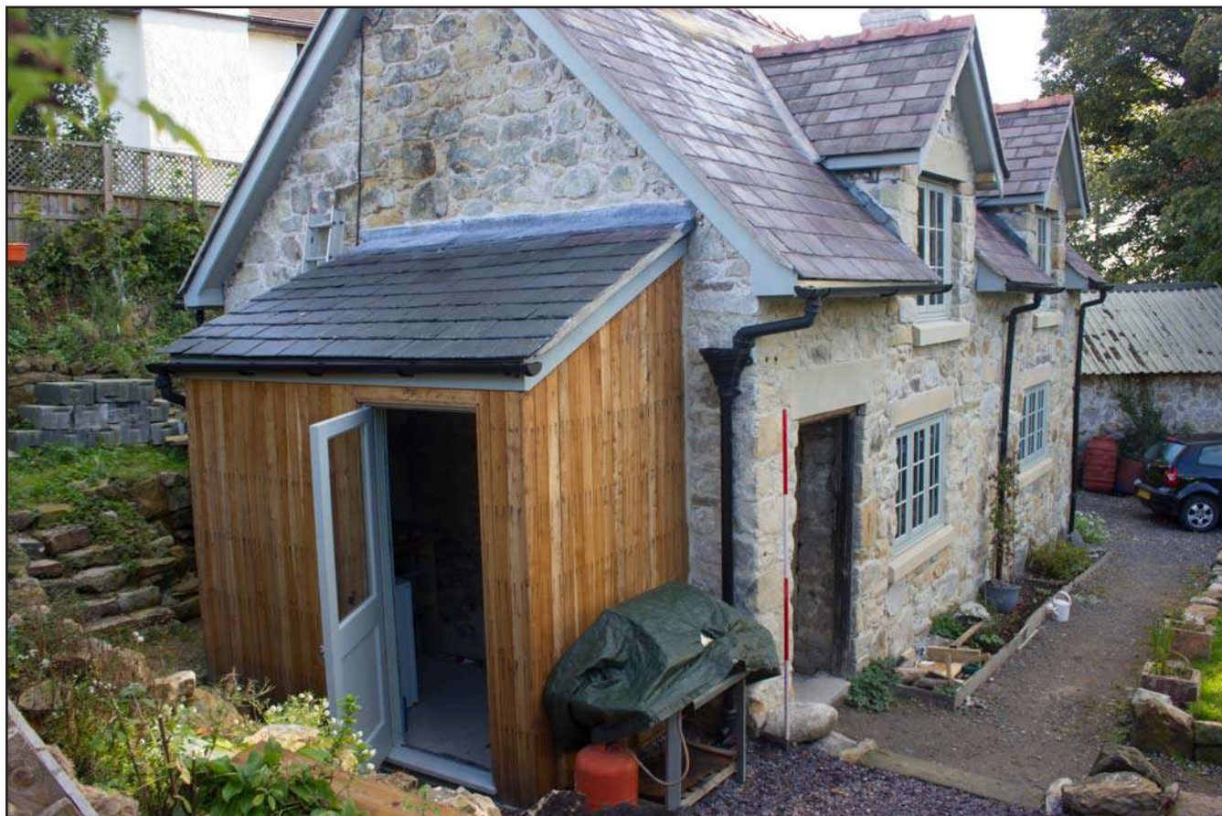
Plate 12: Oblique shot of western and southern elevations of Brookside Cottage, Trevor Hall Road, Garth, Llangollen, Wrexham - from the southwest - 2.00m scale
