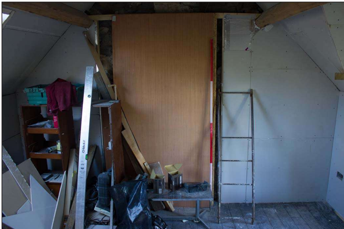
Plate 16: Internal shot of first floor room within Brookside Cottage, Trevor Hall Road, Garth, Llangollen, Wrexham - from the west - 2.00m scale
