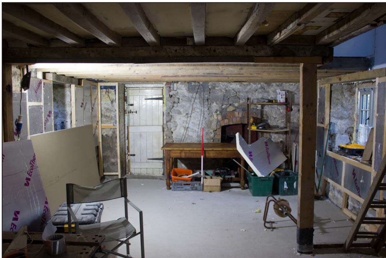
Plate 13: Internal shot of ground floor room within Brookside Cottage, Trevor Hall Road, Garth, Llangollen, Wrexham - from the west - 1.00m scale
