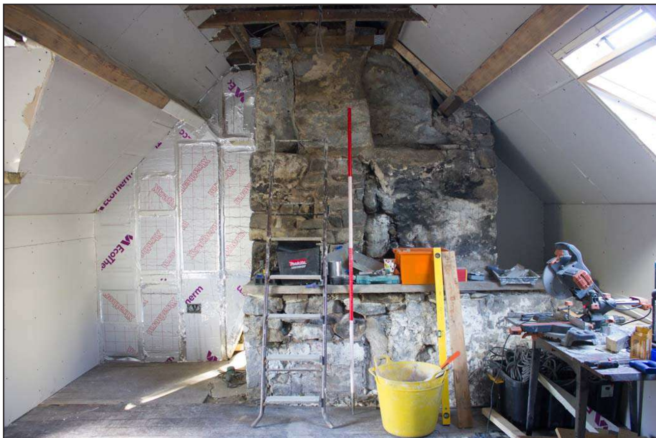
Plate 17: Internal shot of first floor room within Brookside Cottage, Trevor Hall Road, Garth, Llangollen, Wrexham - from the east - 2.00m scale
