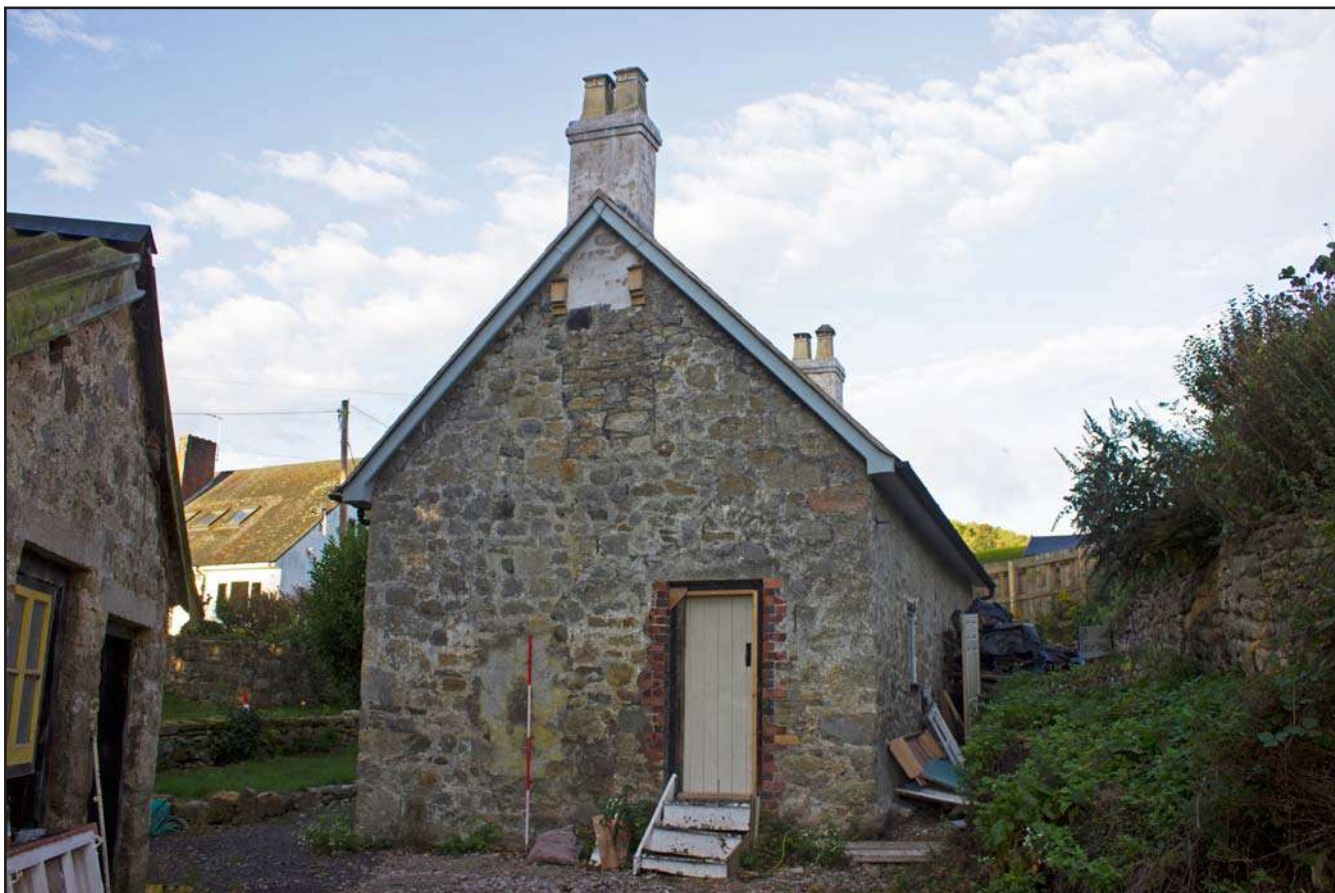
Plate 06: Eastern elevation of Brookside Cottage, Trevor Hall Road, Garth, Llangollen, Wrexham - from the east - 2.00m scale
