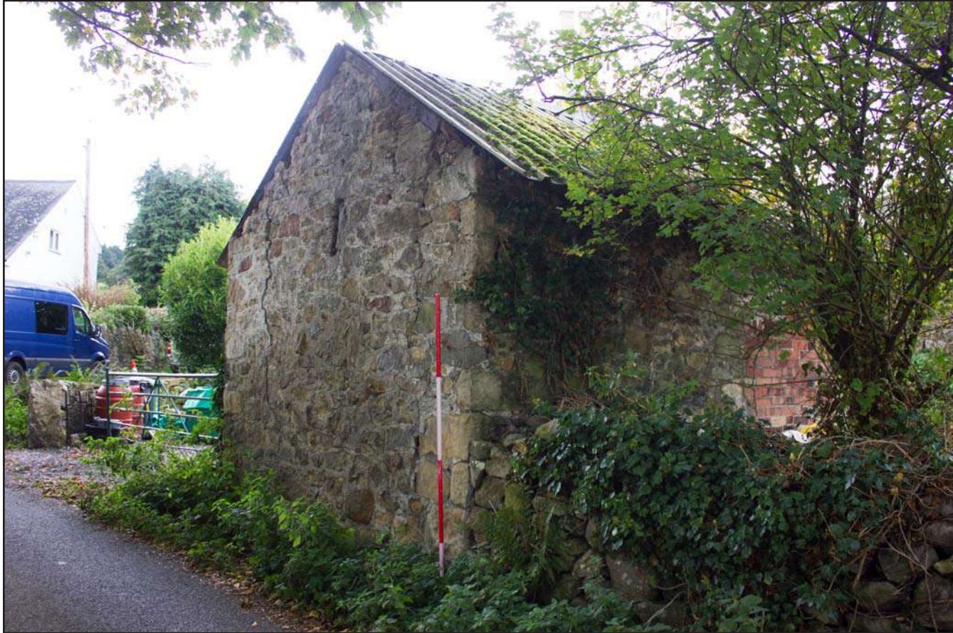
Plate 19: External shot of outbuilding at Brookside Cottage, Trevor Hall Road, Garth, Llangollen, Wrexham - from the east - 2.00m scale
