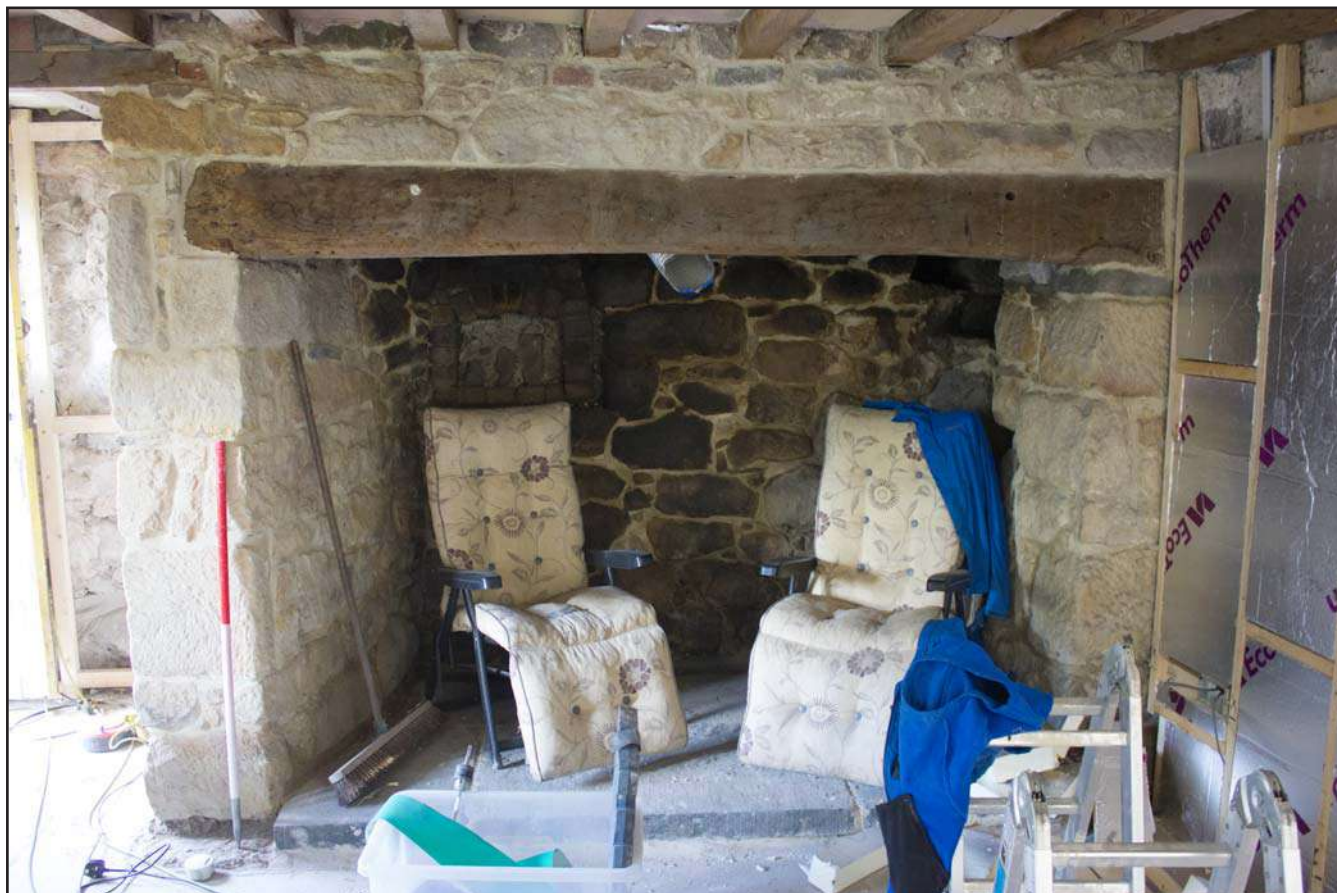
Plate 15: Internal shot of inglenook fireplace within ground floor room at Brookside Cottage, Trevor Hall Road, Garth, Llangollen, Wrexham - from the east - 1.00m scale
