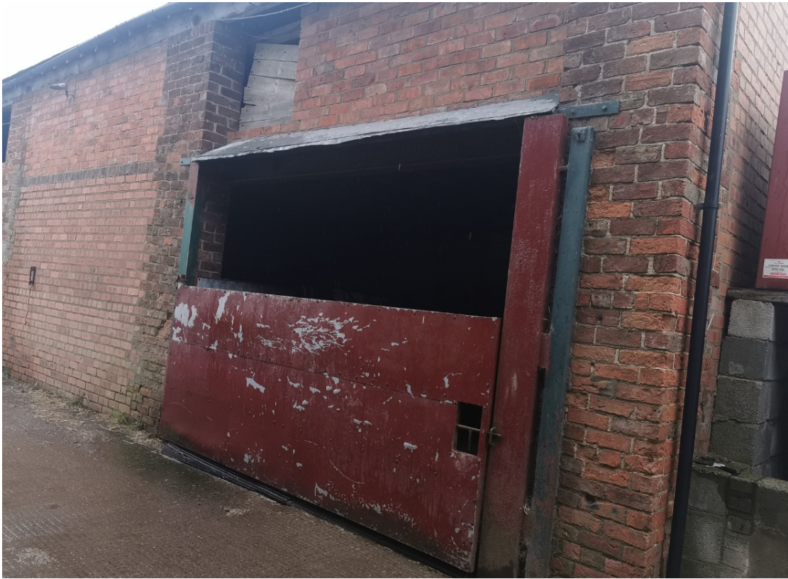
Image of the north west elevation again showing the original corner pier and intermediate pier and later infill panels of brickwork.
