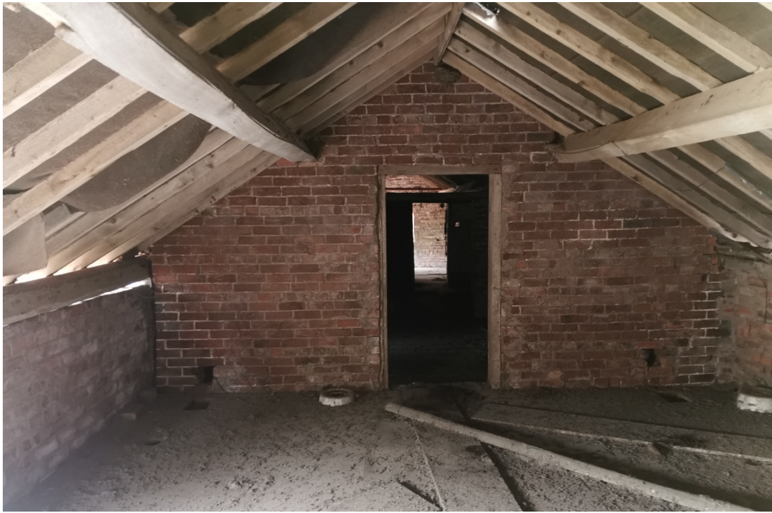
Image of the interior of the building at first floor level from a central position looking north east indicated the vacant condition of the first floor and quality of the traditional roof structure.
