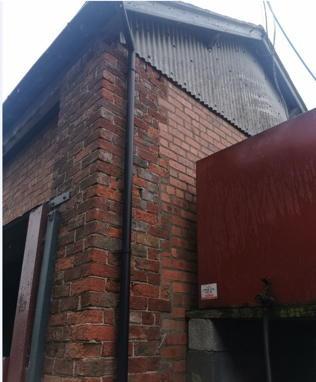
Image of the westernmost corner of the building clearly showing the original hand-made brickwork pier at the corner of the building with later infill brickwork panel to the north west and south west elevations.
