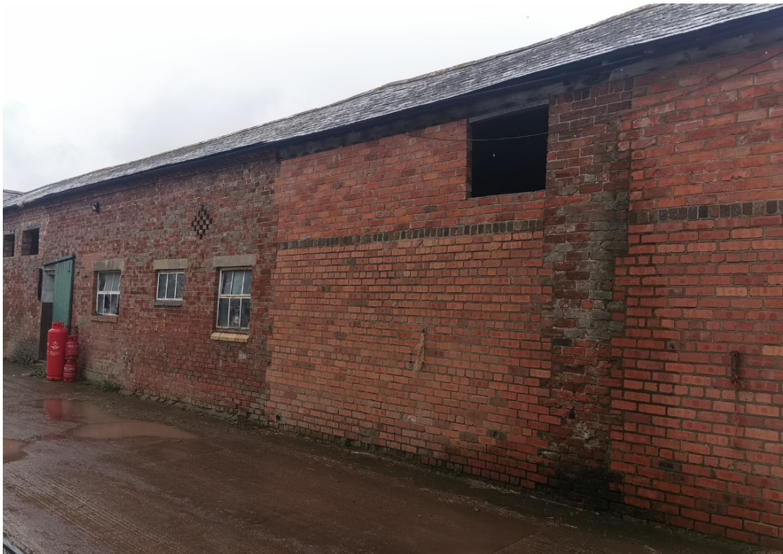
Further image of the north west elevation showing the second and third modern brickwork infill panels.
