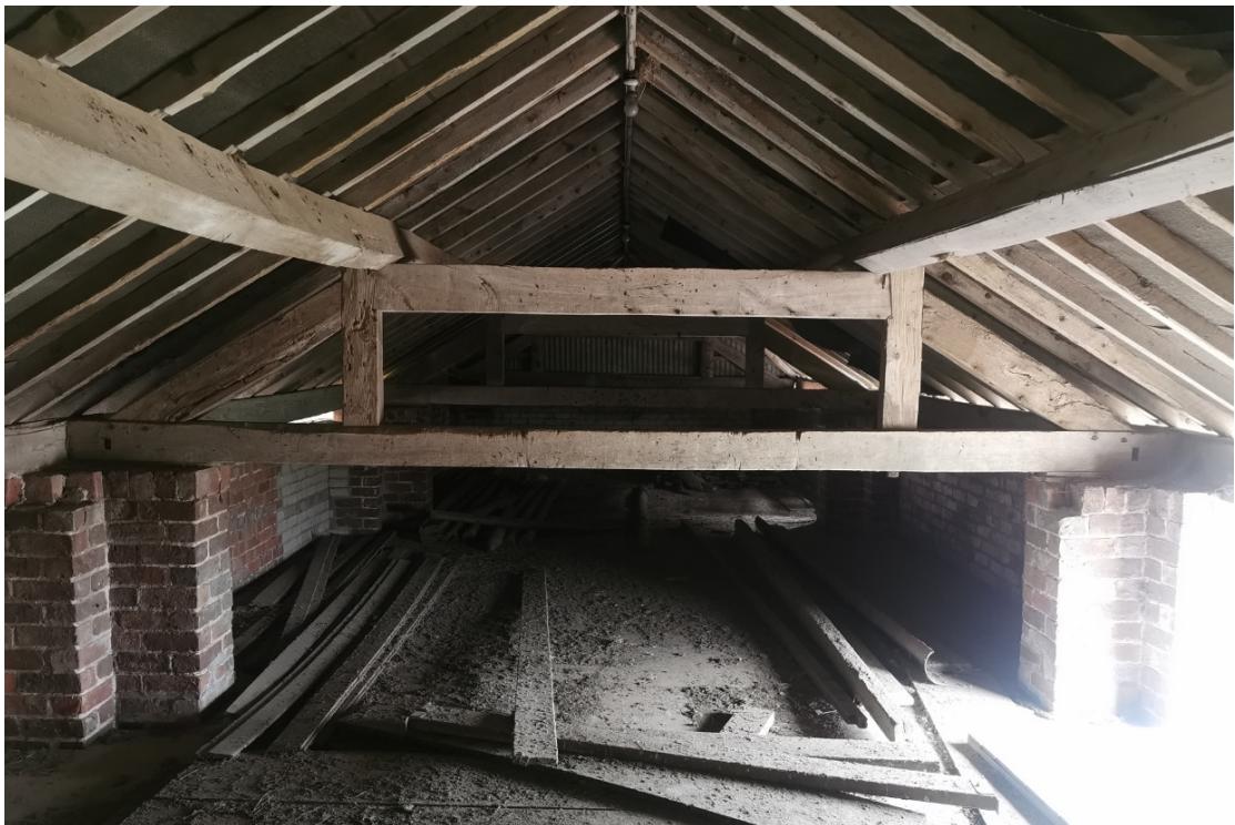
Image of the interior of the building at first floor level from a central position looking south west and showing the Oak Queen Post Trusses supporting the purlins which will require modification to allow unimpeded access to all parts of the building at first floor level.
