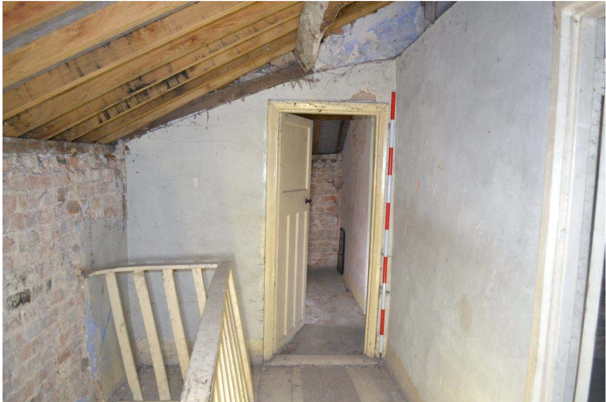
Plate 42: First Floor, Landing.
