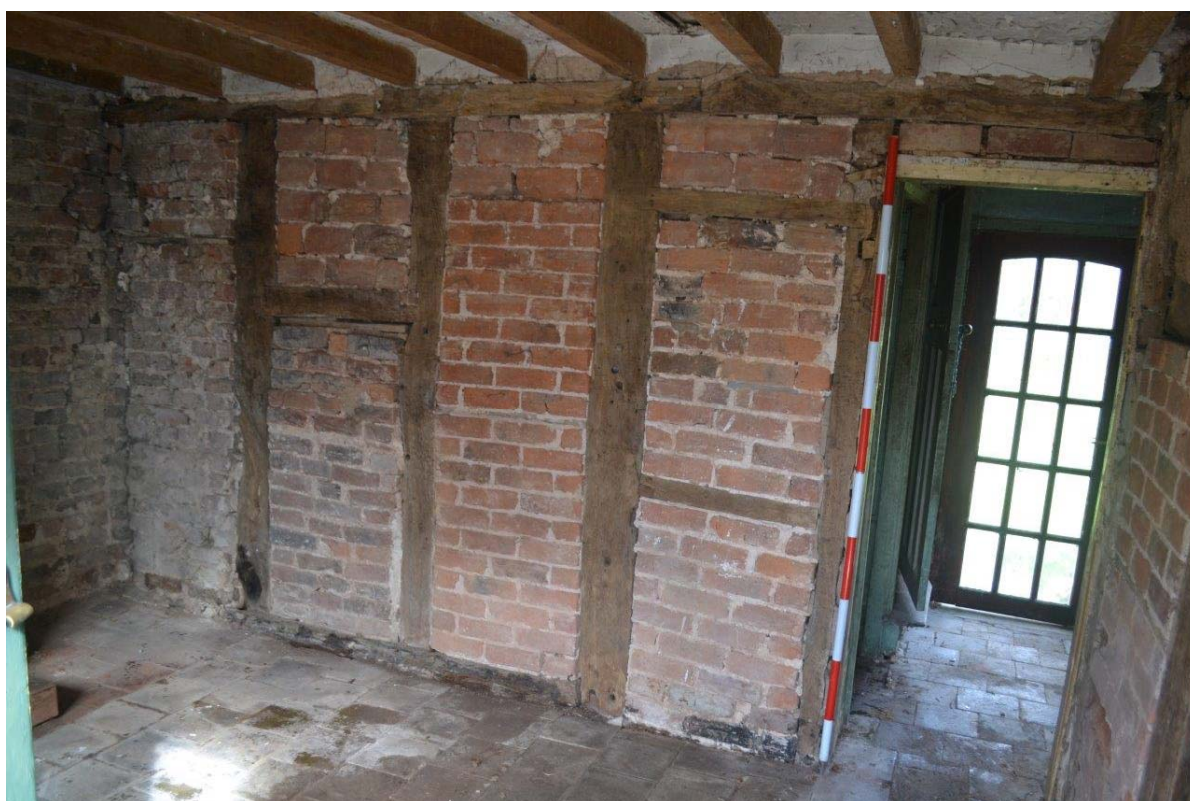
Plate 17: Ground Floor, Principal Living Room, The internal wall separating the principal living room from the pantry. Constructed from orthogonal small-framing in the form of timber studs and rails with infilling horizontal brick nogging. Brick nogging often replaced wattle and daub. Scale =2m.
