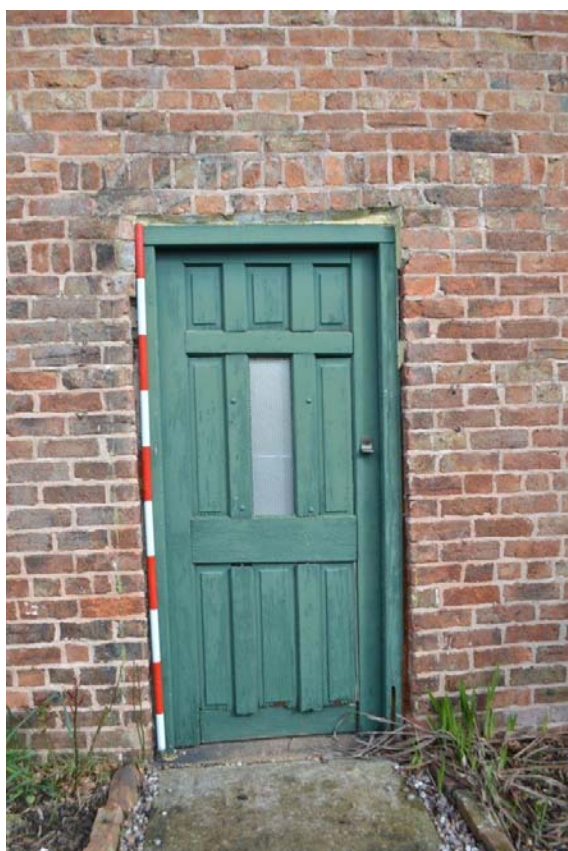
Plate 4: Timber entrance door to south-facing façade. Nine panels with central given over to fenestration. Timber door case and flat rowlock course above.
