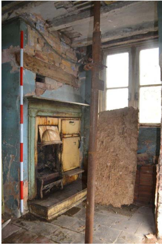
Plate 28: Ground Floor Kitchen. Cooking range with open fire to left and two oven to right. Scale = 2m.
