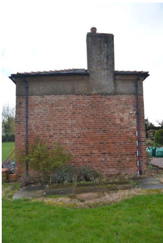
Plate 13: Sightline to the east showing the window-less west-facing elevation, plastic rain-water goods and the chimney integrated into the side-wall. There is cementitious render to the final few brick courses. Scale =2m
