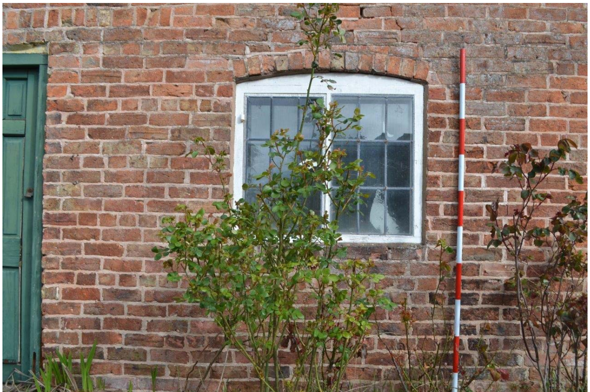
Plate 6: Sightline to the ground floor window serving the private room, under a cambered, single-course, rowlock segmental arch head to the right of the entrance door. Window details as per left-hand side. Scale = 2m.
