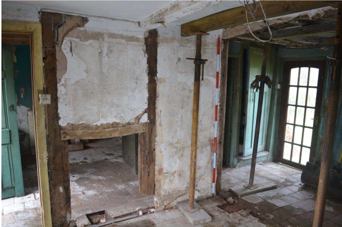
Plate 26: Ground Floor, Private Room showing the studs, rails and plastered panels to the wall separating the Private Room from the Principal Living Room. Scale = 2m
