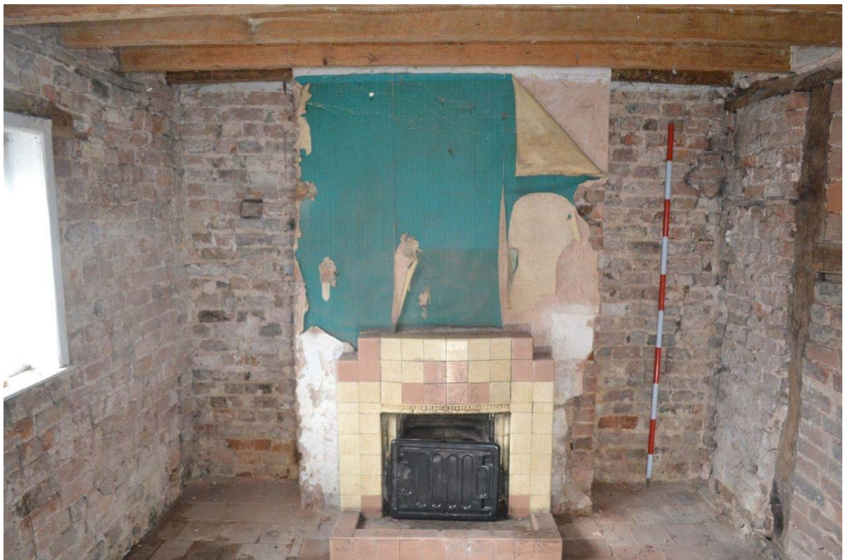
Plate 15 Ground Floor, Principal Living Room. Chimney breast and mid-20 th century fireplace. Scale =2m
