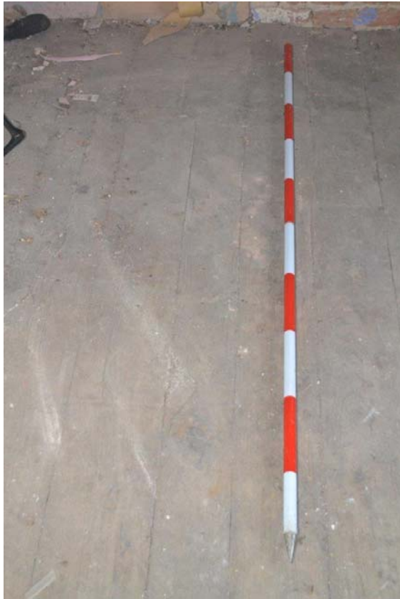
Plate 48: First Floor Bedroom 1. Deal boards forming bedroom floor.
