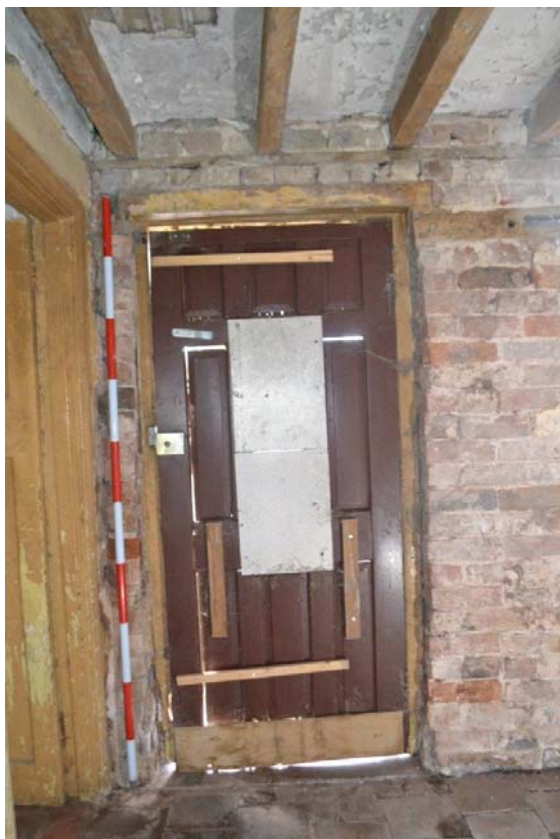
Plate 18: Ground Floor, Principal Living Room,
