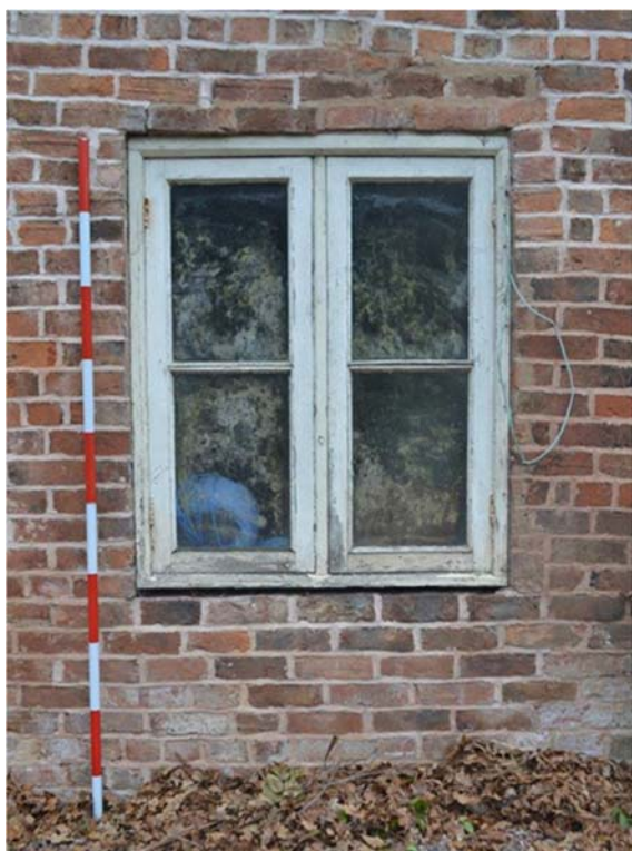
Plate 9: Sightline detailing the four-pane timber casement window to the kitchen. Scale =2m
