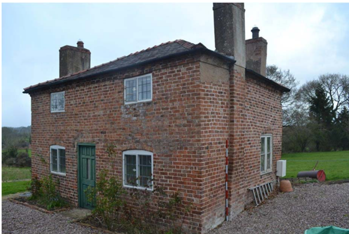
Plate 7: Oblique sightline to the north-west showing the south-facing entrance façade and the east-facing elevation. Scale =2m.
