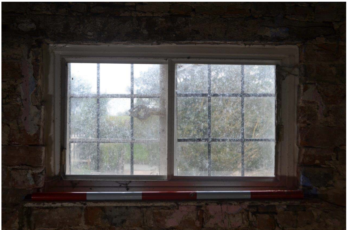
Plate 47: First Floor Bedroom 1. Multi-paned casement window. Scale = 1m.
