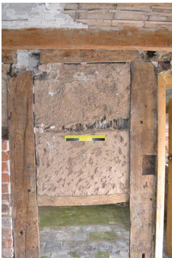
Plate 19: Ground Floor, Principal Living Room. Detail of the studs, rails and wattle and daub panel in the internal wall separating the principal living room from the private room. Scale = 30cm
