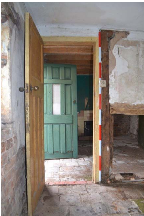
Plate 25: Ground Floor, Private Room. Looking through the door into the through passage and Principal Living Room. Note Ruabon quarry tiles providing the floor surface. Scale = 2m.
