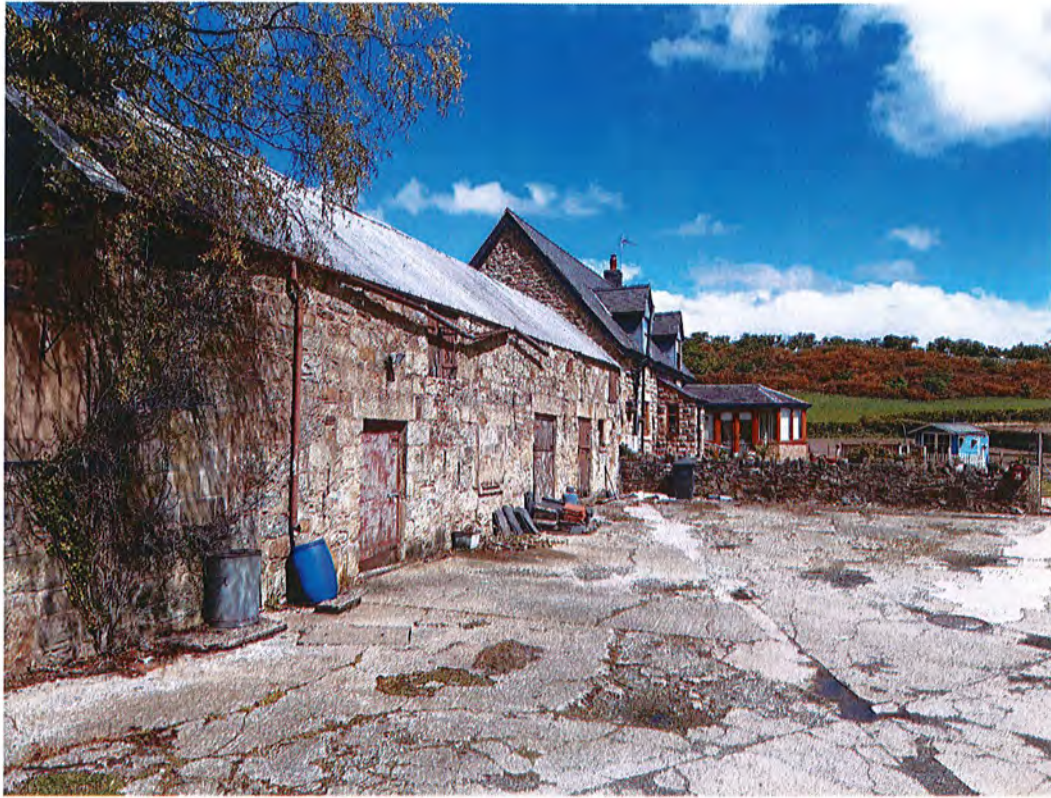
Photograph 7: Southern side of barn
