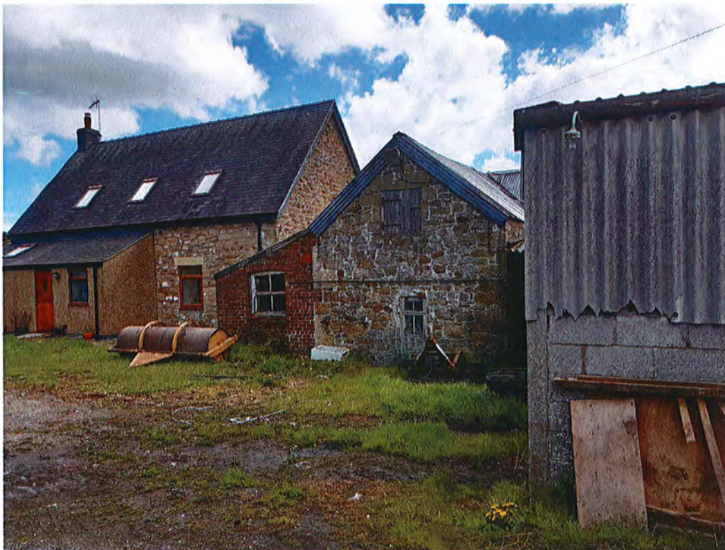
Photograph 6: Showing north east corner of site
