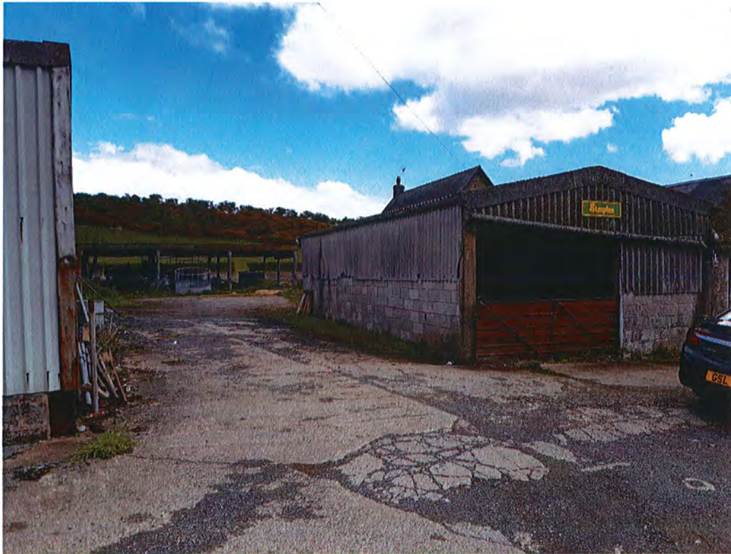
Photograph 5: Showing access road to north of site and farm building
