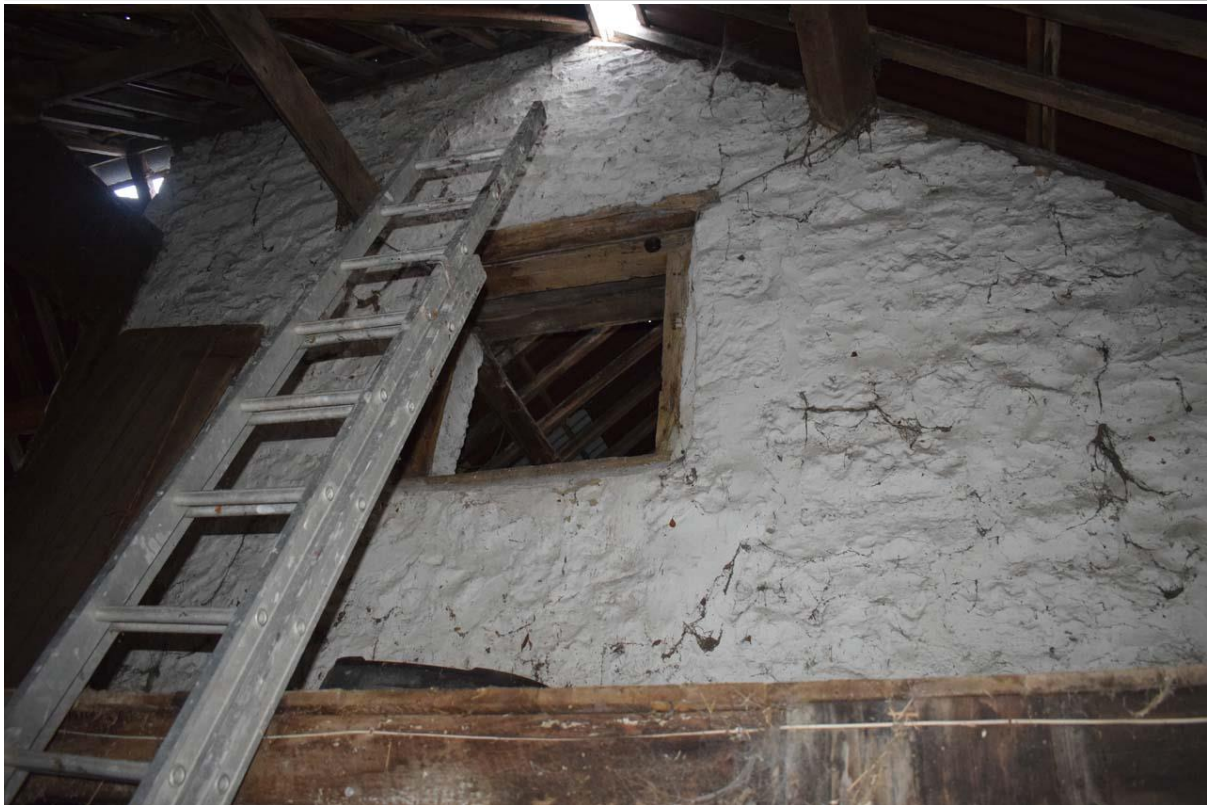
Fig. 12 Eastern hay loft entrance., possibly not primary entrance. CPAT photo 4950-0036
