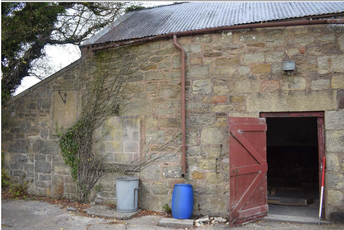
Fig. 7 Detail view of southern face of barn, west end, viewed from south. CPAT photo 4950-0039
