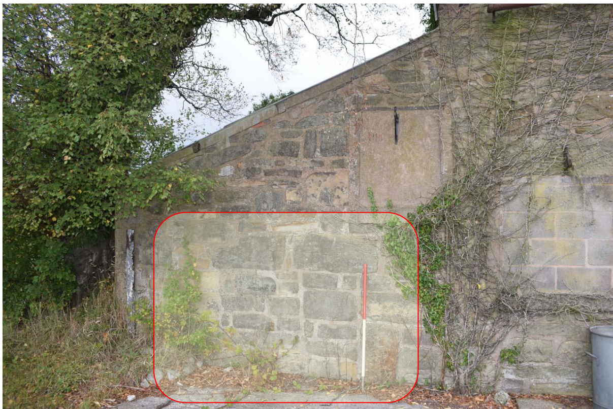
Fig. 21 Edited photograph with red box showing former points of ingress which may indicate animal pens. From CPAT photo 4950-0072
