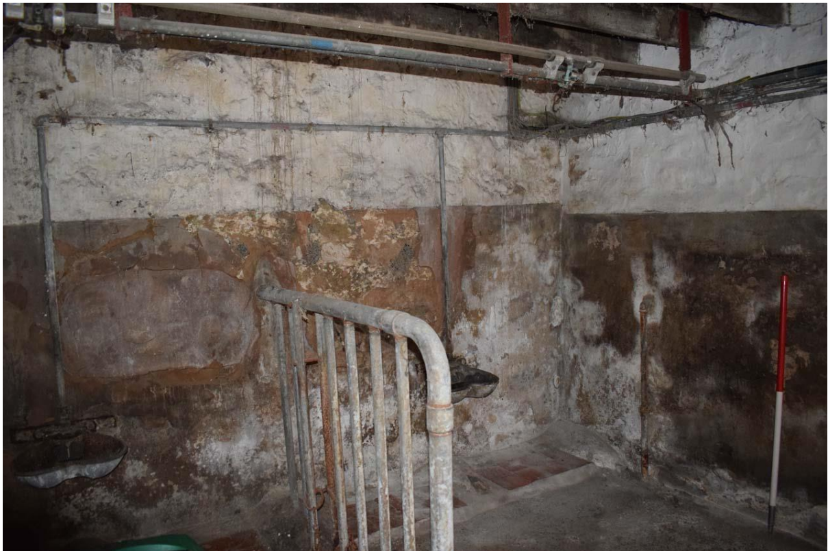
Fig. 9 cattle cleaning stations in the easternmost room. CPAT photo 4950-0004
