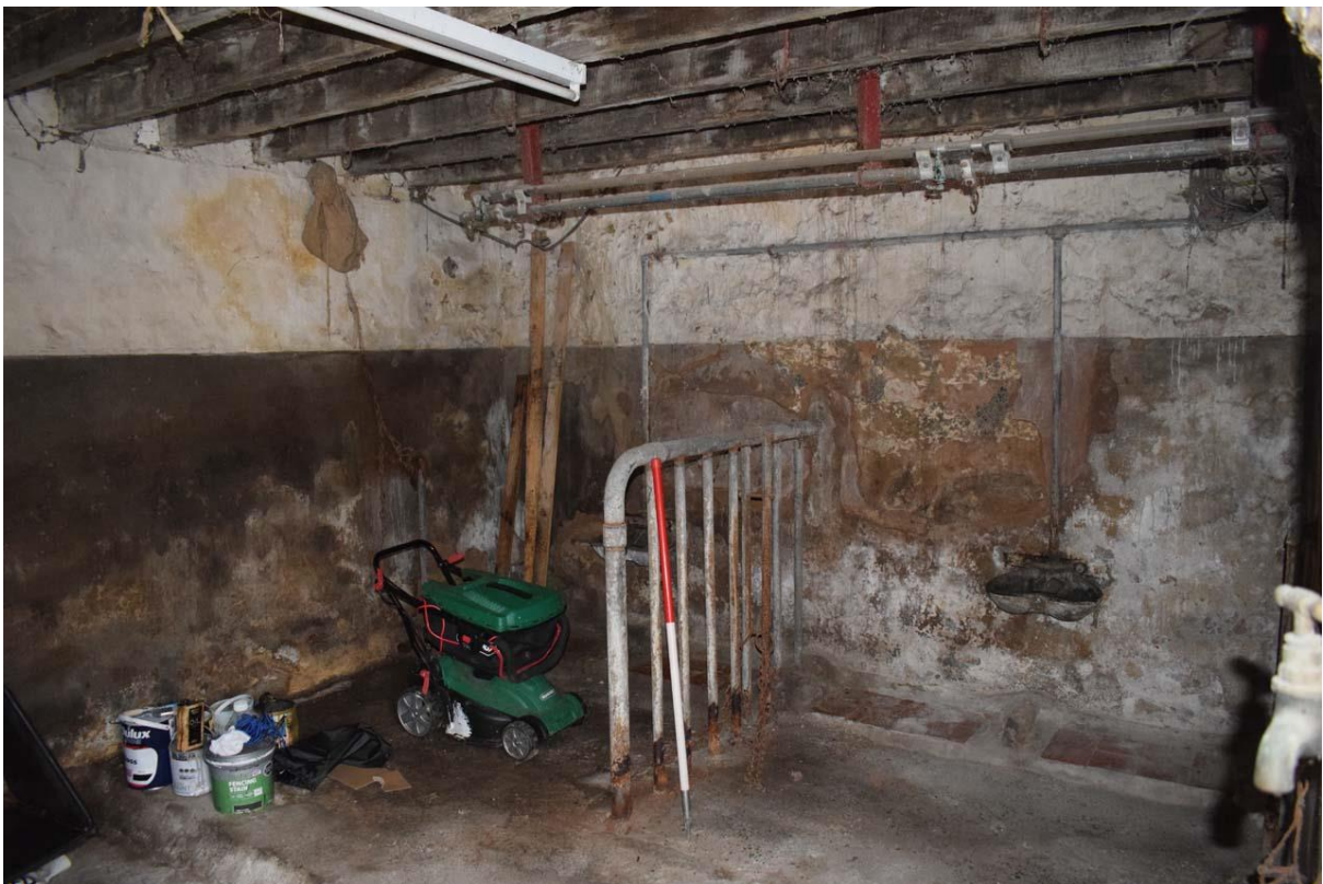
Fig. 10 Cattle cleaning stations in the easternmost room. CPAT photo 4950-0006
