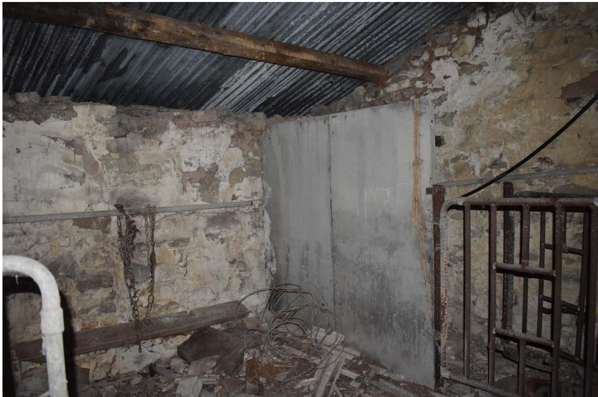
Fig. 19 Smaller room with sloped roof, interior. CPAT photo 4950-0064
