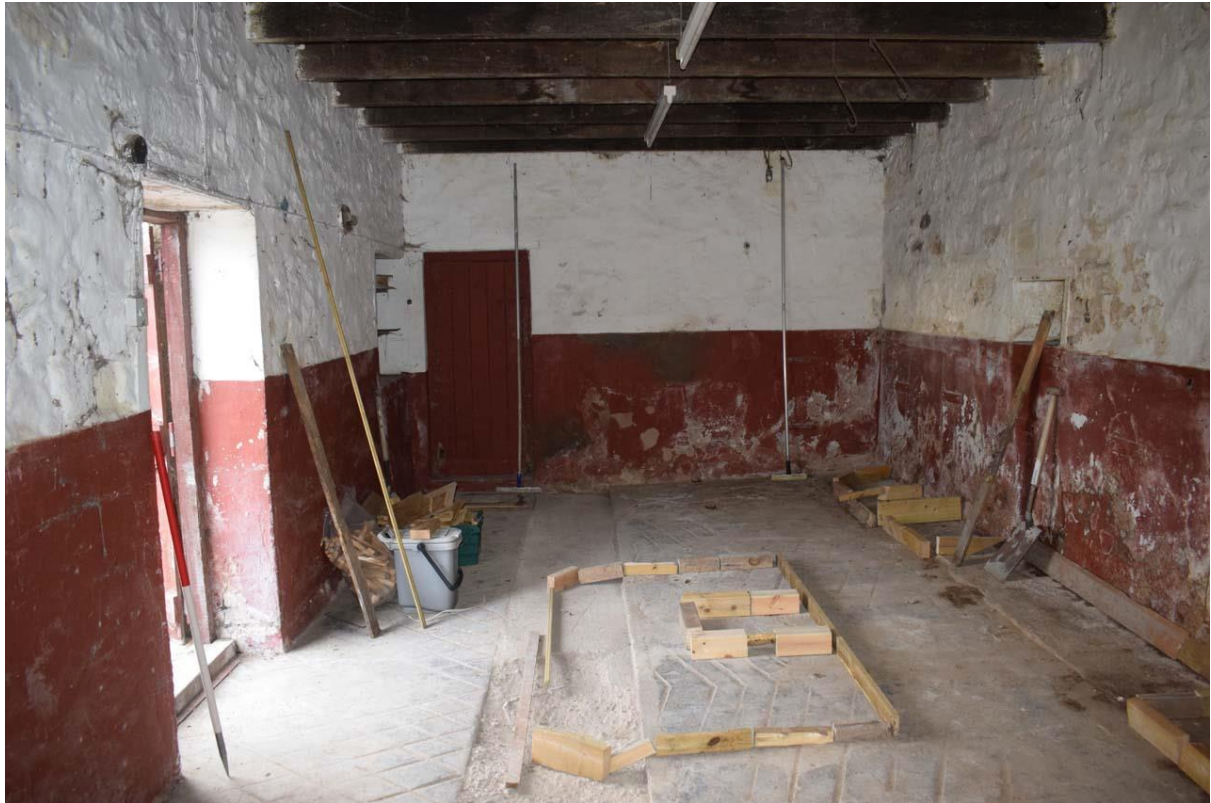
Fig. 17 Large room in the west of the barn, looking west. CPAT photo 4950-0044
