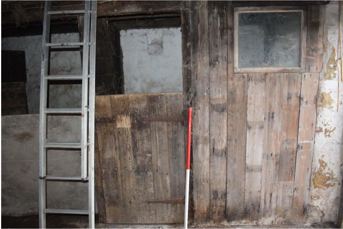
Fig. 16 Small shed structure within central room of barn. CPAT photo 4950-0028
