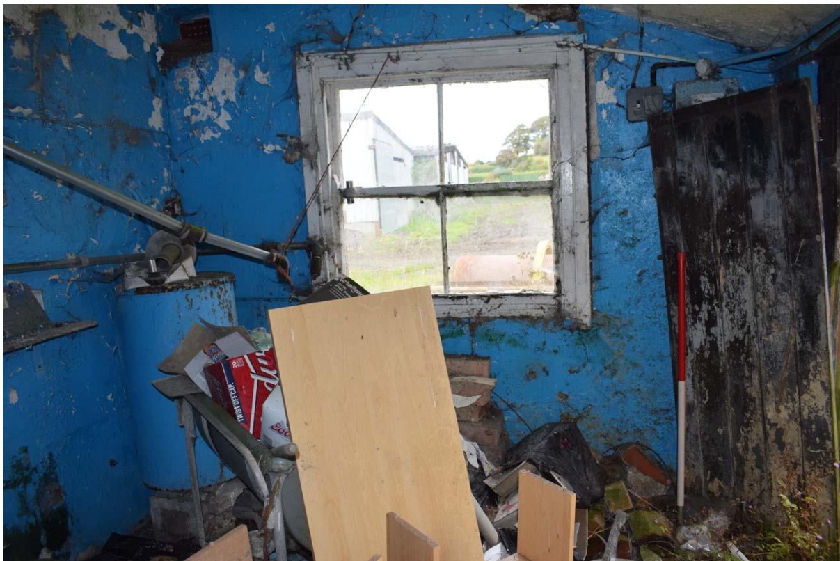
Fig. 25 Interior of brick extension. CPAT photo 4950-0053
