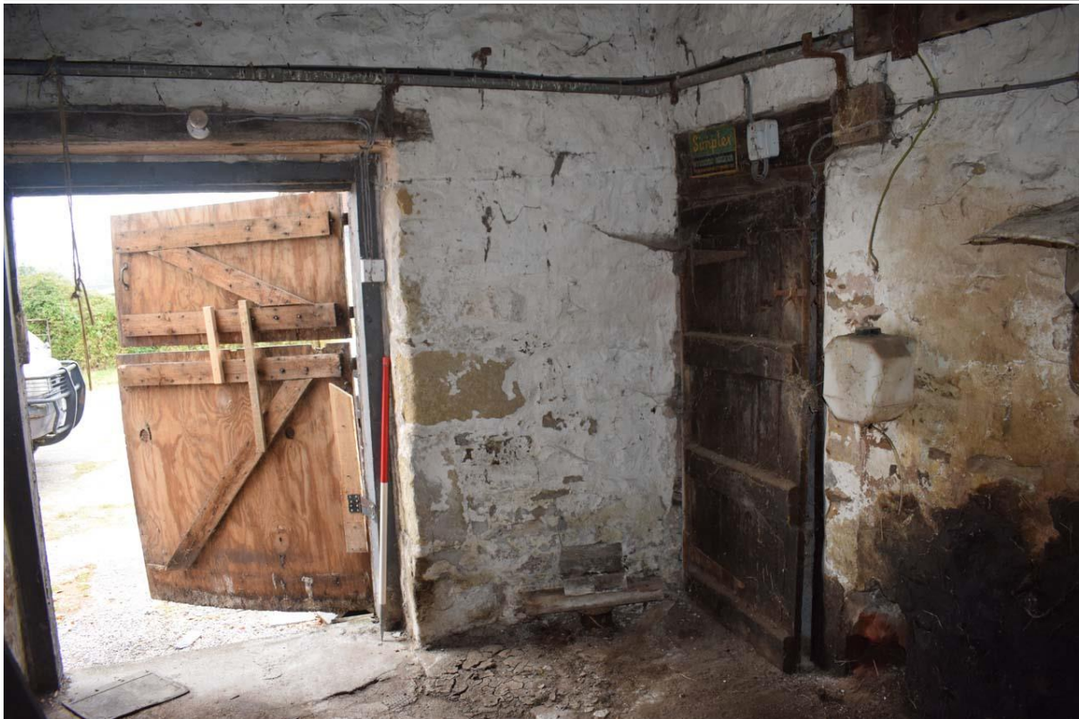
Fig. 8 Interior view of exterior doorway and an interior doorway. CPAT photo 4950-0013
