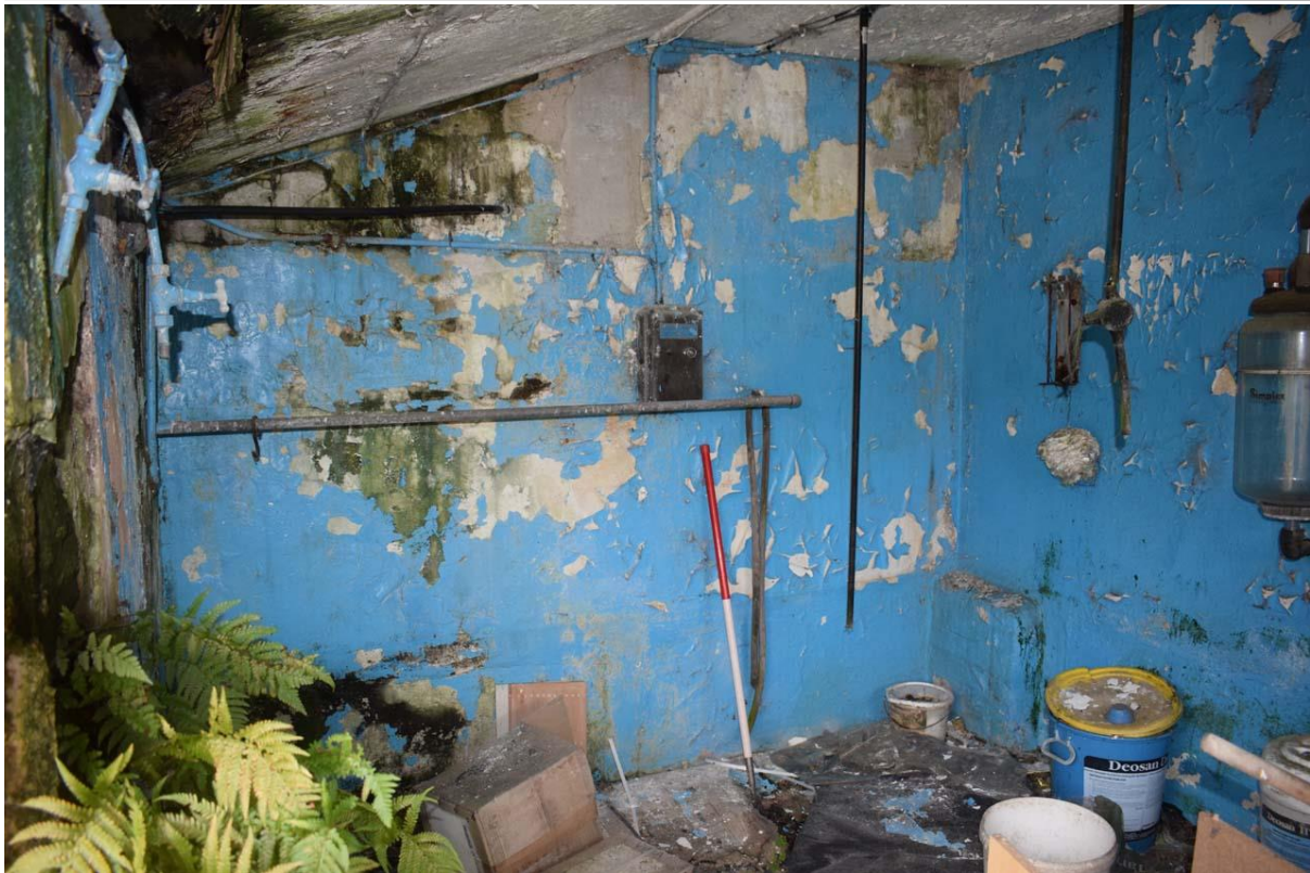
Fig. 24 Interior of brick extension. CPAT photo 4950-0051
