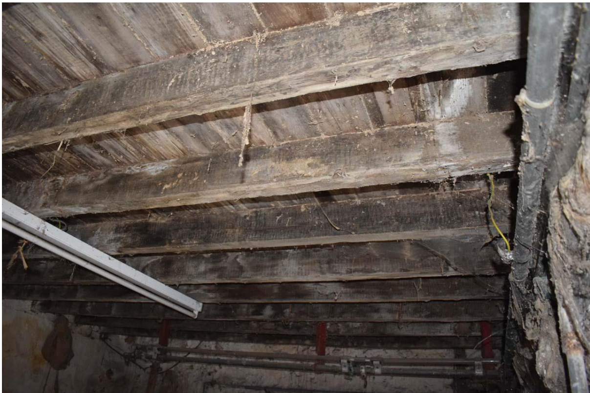
Fig. 13 Joists forming the floor to the hay loft above the easternmost room. CPAT photo 4950-0011
