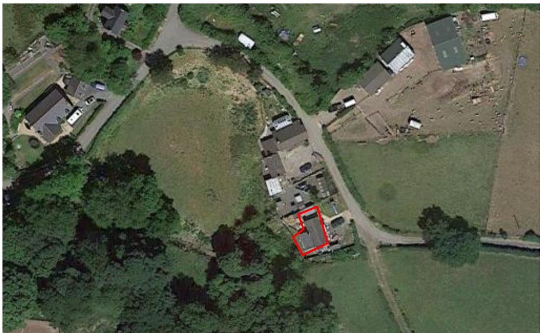
Aerial view of the building at Target Note 2 and immediate surroundings. Base Image © Google 2021.
