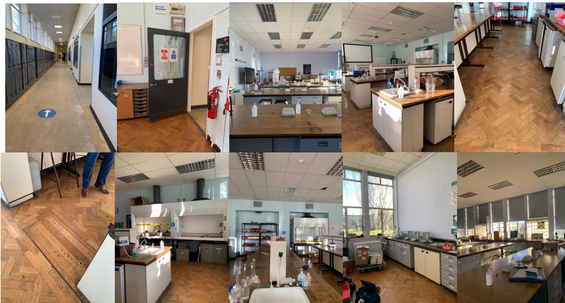
Fig 6. Corridor C, doors to the labs, modern desks, parquet flooring in herringbone pattern, dockets in floor to access air ducts, extract cupboards (some removed). Note suspended ceiling, fenestration and view out to the courtyard, and the room orientation.
