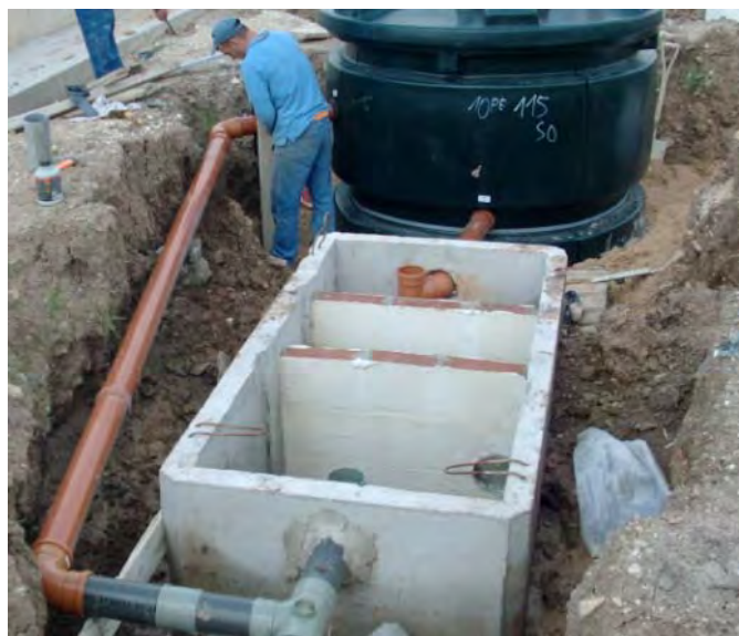
Picture of 3 chamber settling tank for 5 PE system built on site.
