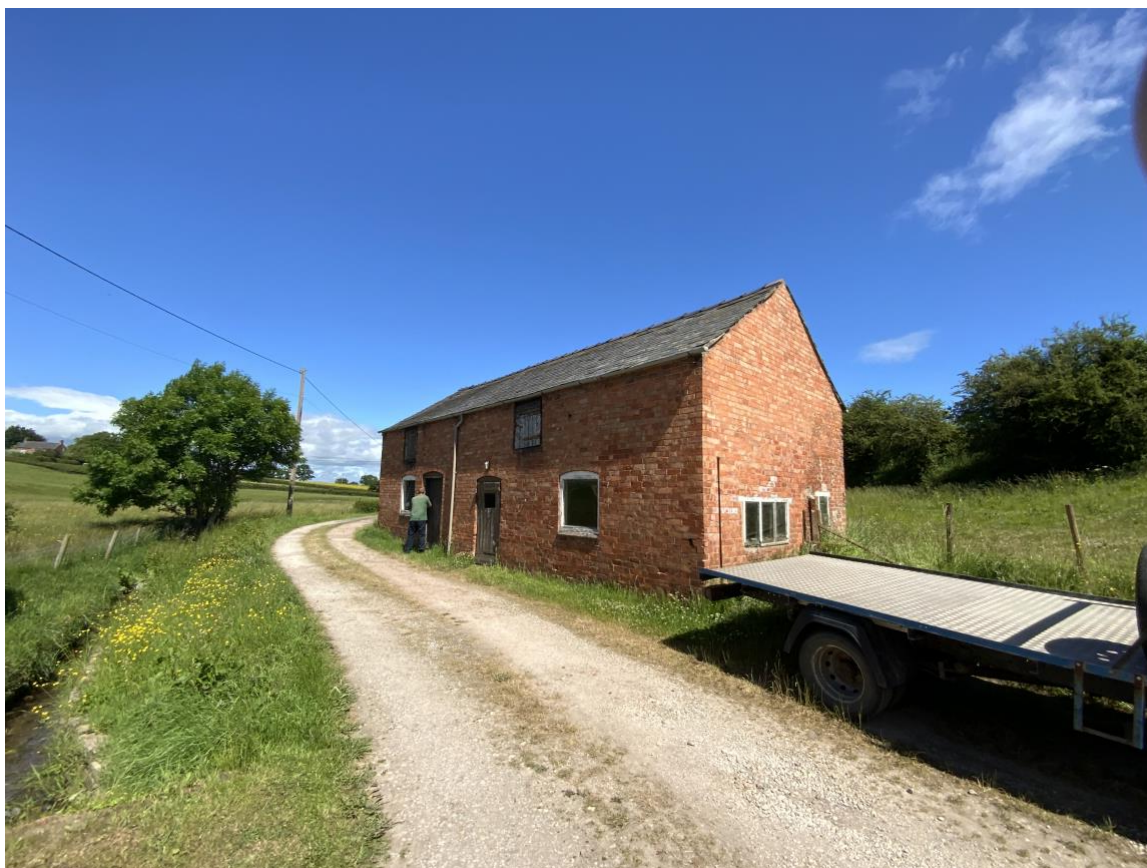
View from the south west side of the building.
