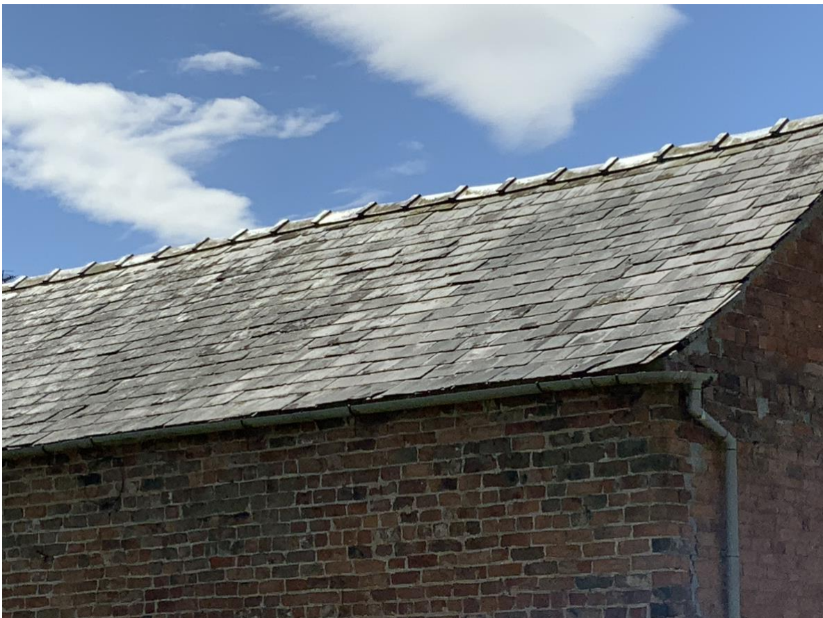
The roof slates are in fairly good condition and there are few roosting opportunities beneath the slates.
