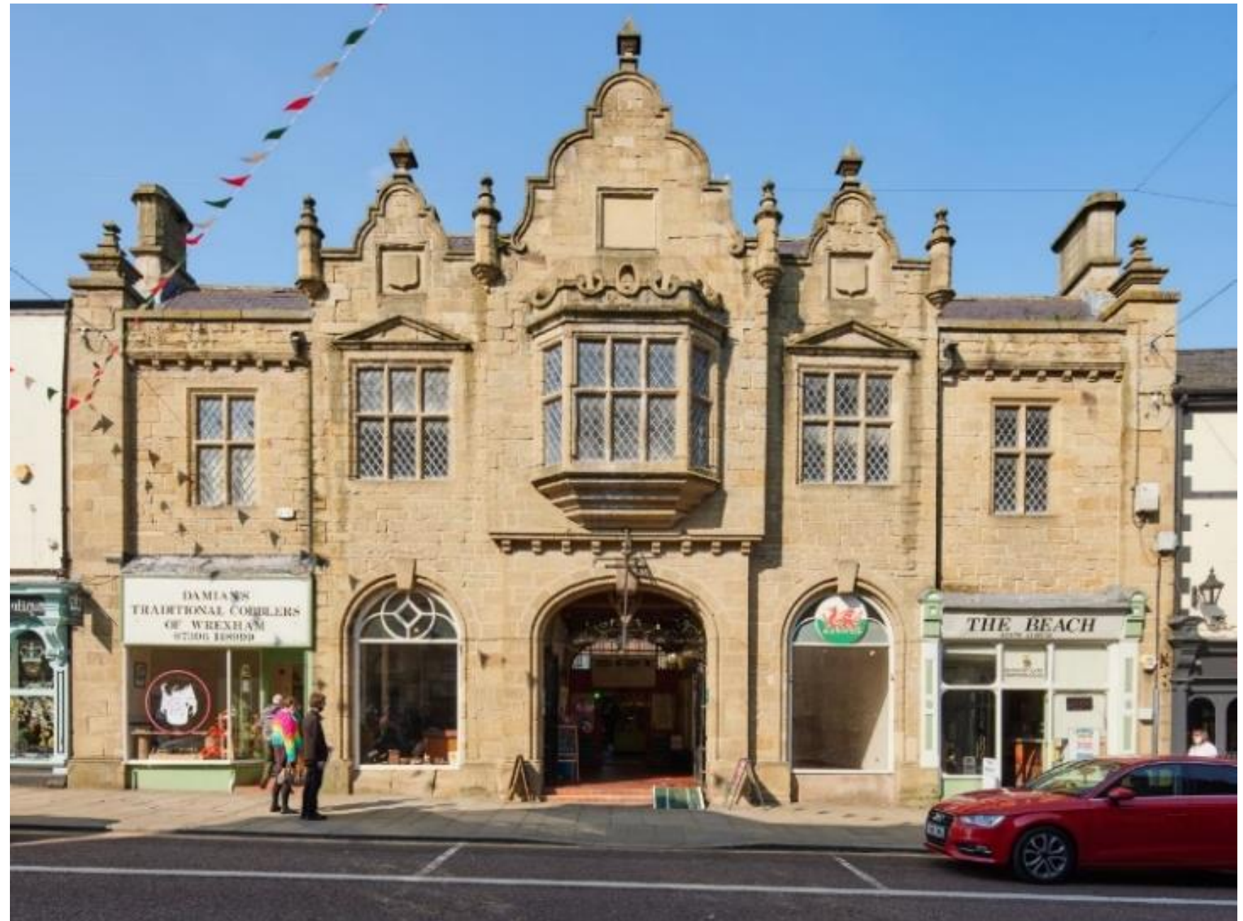
Existing Butchers Market frontage to High Street:
