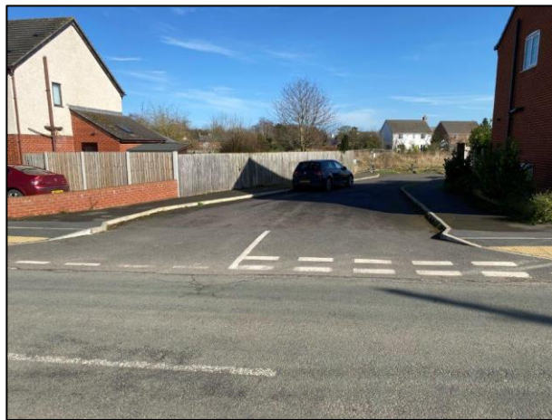
Figure 3: Existing Shared Access Road
