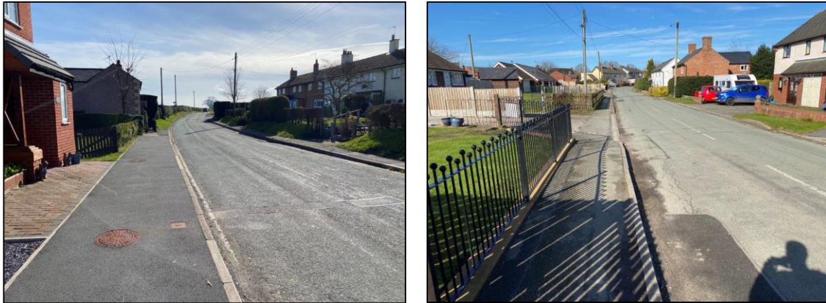
Figure 9: Pedestrian Footways on Bettisfield Road
