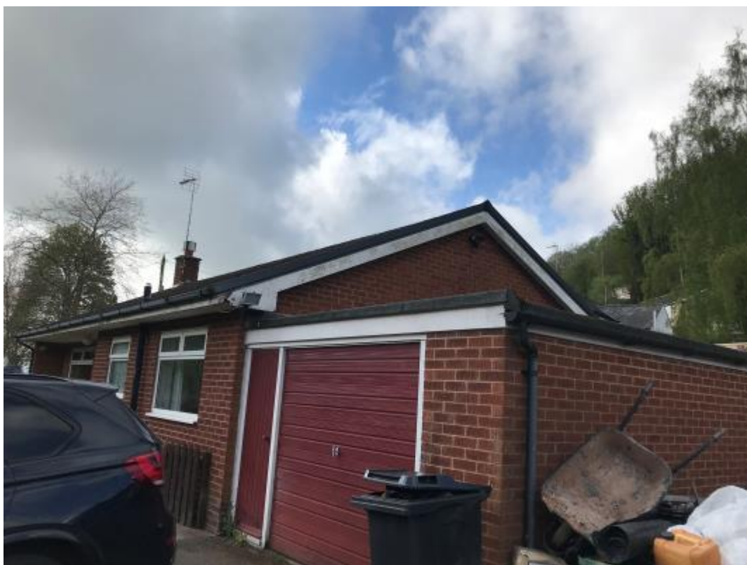
Plate 3 – A view of the flat-roofed garage
