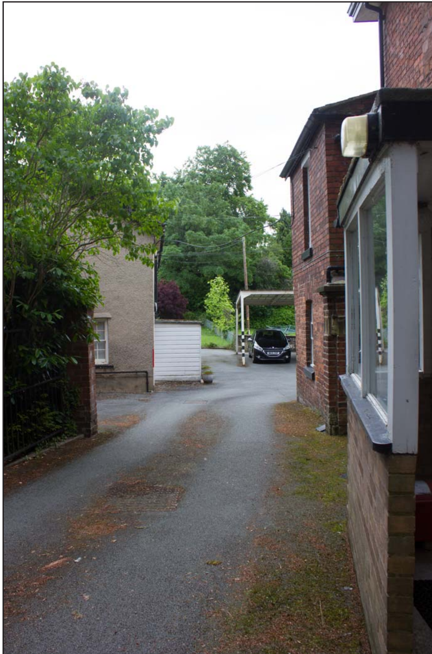
Plate 18: Context shot of the Diocesan Office situated to northeast of The Bishop's House, 17 Sontley Road, Wrexham - from the west - 1.00m scale
