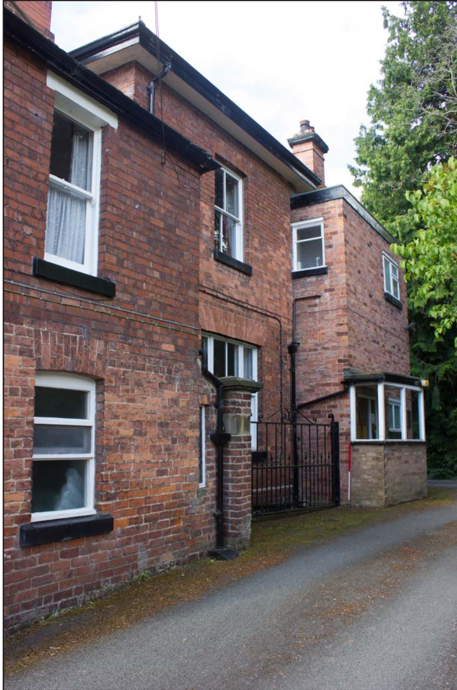
Plate 04: Northern extension, oblique shot on the The Bishop's House, 17 Sontley Road, Wrexham - from the east-northeast - 1.00m scale
