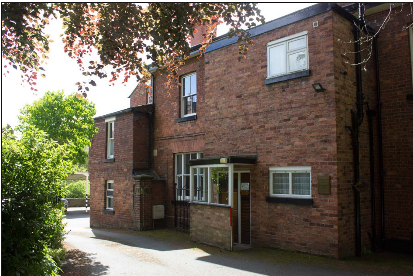
Plate 05: Northern extension, oblique shot on the The Bishop's House, 17 Sontley Road, Wrexham - from the northwest - 1.00m scale
