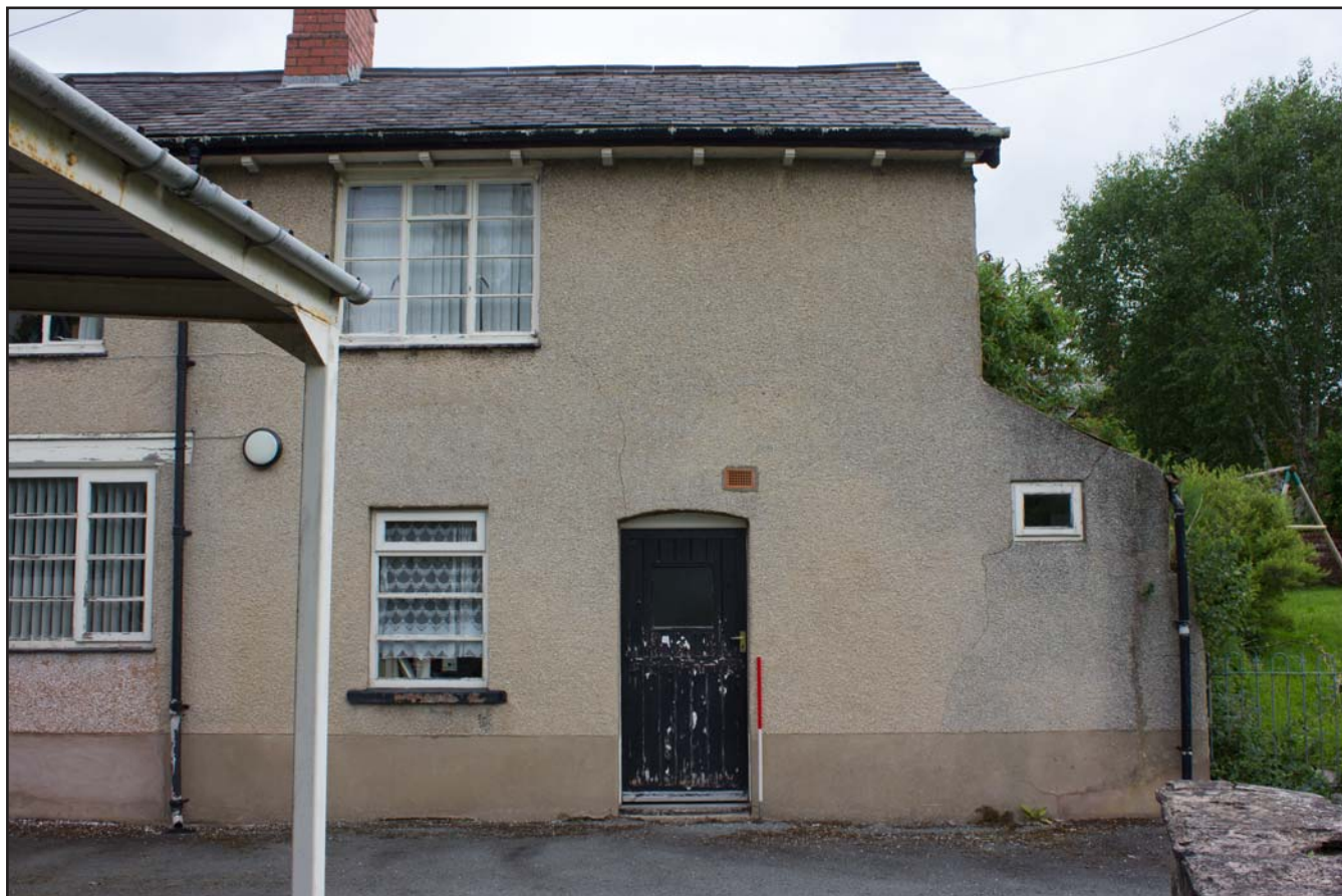
Plate 24: Southern elevation (right) of the of the diocesan office at The Bishop's House, 17 Sontley Road, Wrexham - from the south - 1.00m scale
