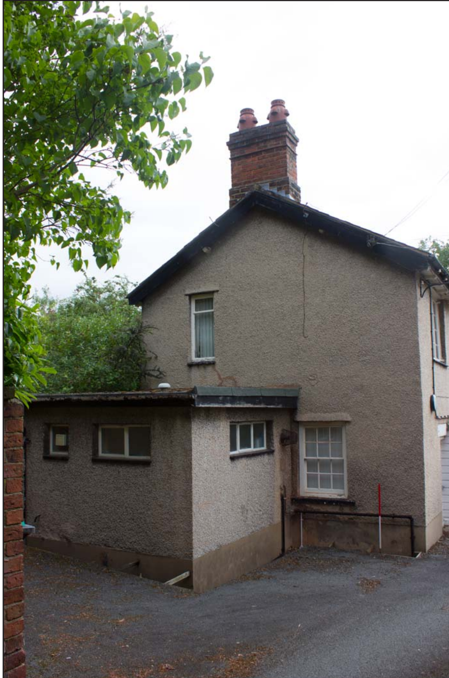
Plate 29: Western elevation of the of the diocesan office at The Bishop's House, 17 Sontley Road, Wrexham - from the west - 1.00m scale
