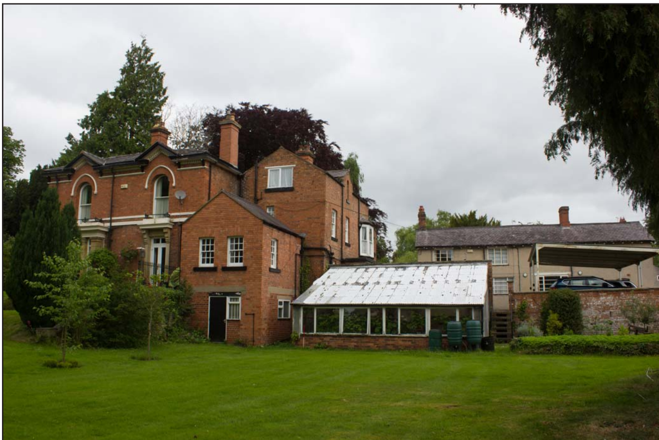
Plate 08: Context shot of the greenhouse situated to south of house, The Bishop's House, 17 Sontley Road, Wrexham - from the west-southwest - 1.00m scale
