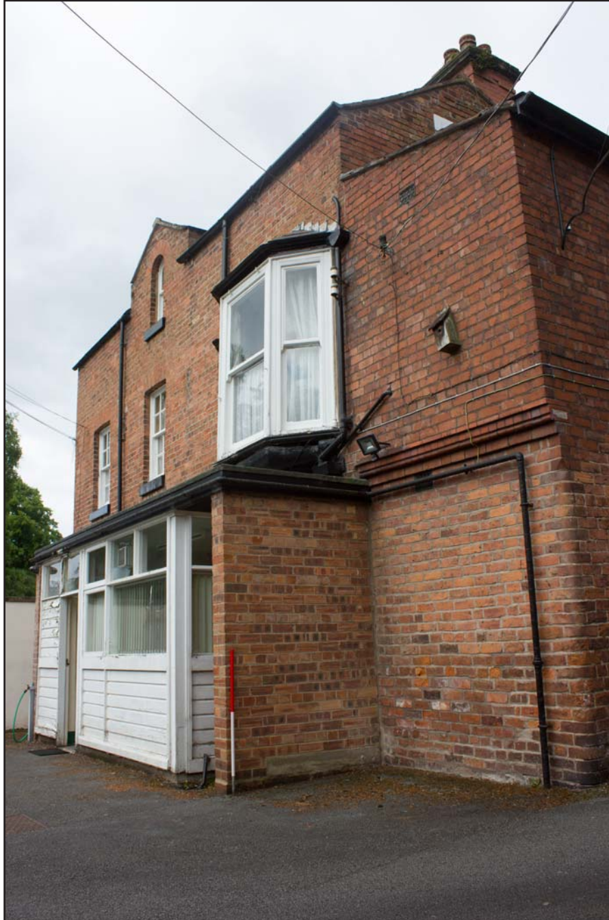
Plate 01: Rear extension, oblique shot - north & east elevations of The Bishop's House, 17 Sontley Road, Wrexham - from the northeast - 1.00m scale
