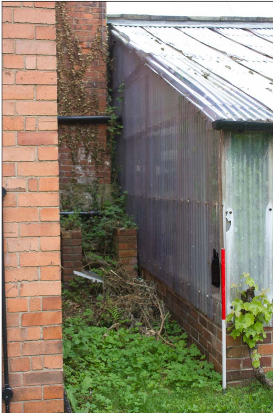
Plate 13: Western elevation of the greenhouse in the garden at The Bishop's House, 17 Sontley Road, Wrexham - from the south-southwest - 1.00m scale
