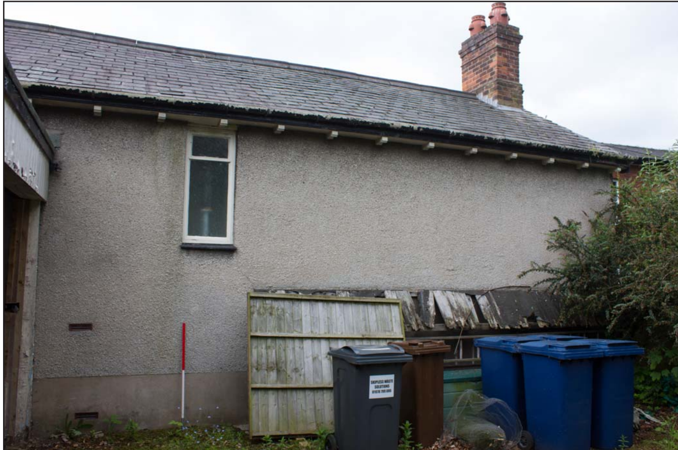
Plate 30: Northern elevation of the of the diocesan office at The Bishop's House, 17 Sontley Road, Wrexham - from the north - 1.00m scale
