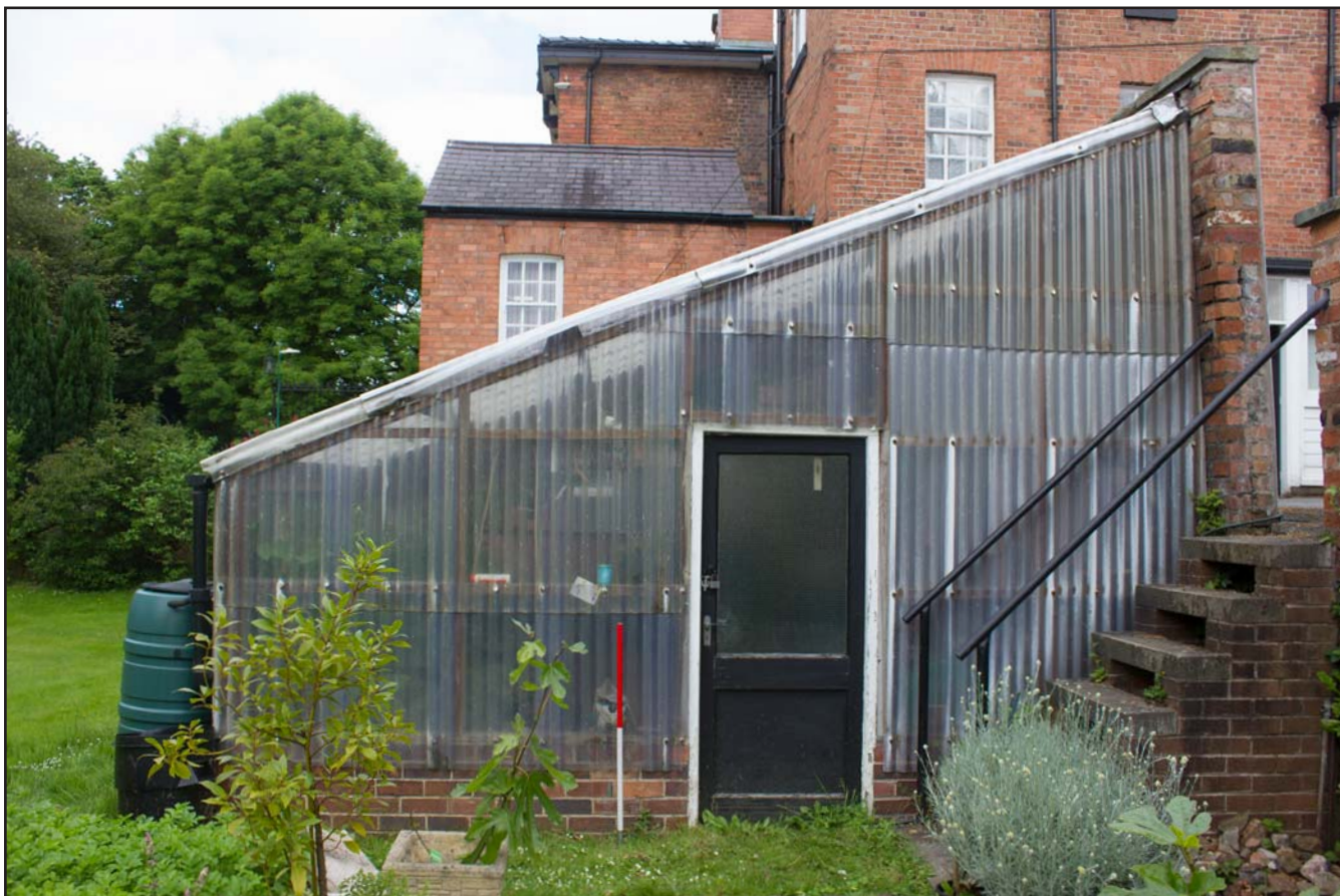
Plate 09: Eastern elevation of the greenhouse in the garden at The Bishop's House, 17 Sontley Road, Wrexham - from the east - 1.00m scale
