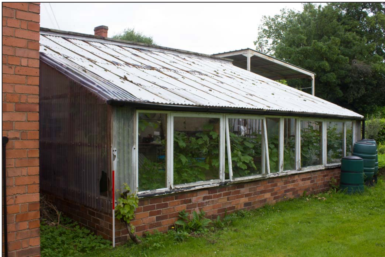
Plate 12: Oblique shot of the greenhouse, southern and western elevations at The Bishop's House, 17 Sontley Road, Wrexham - from the southwest - 1.00m scale
