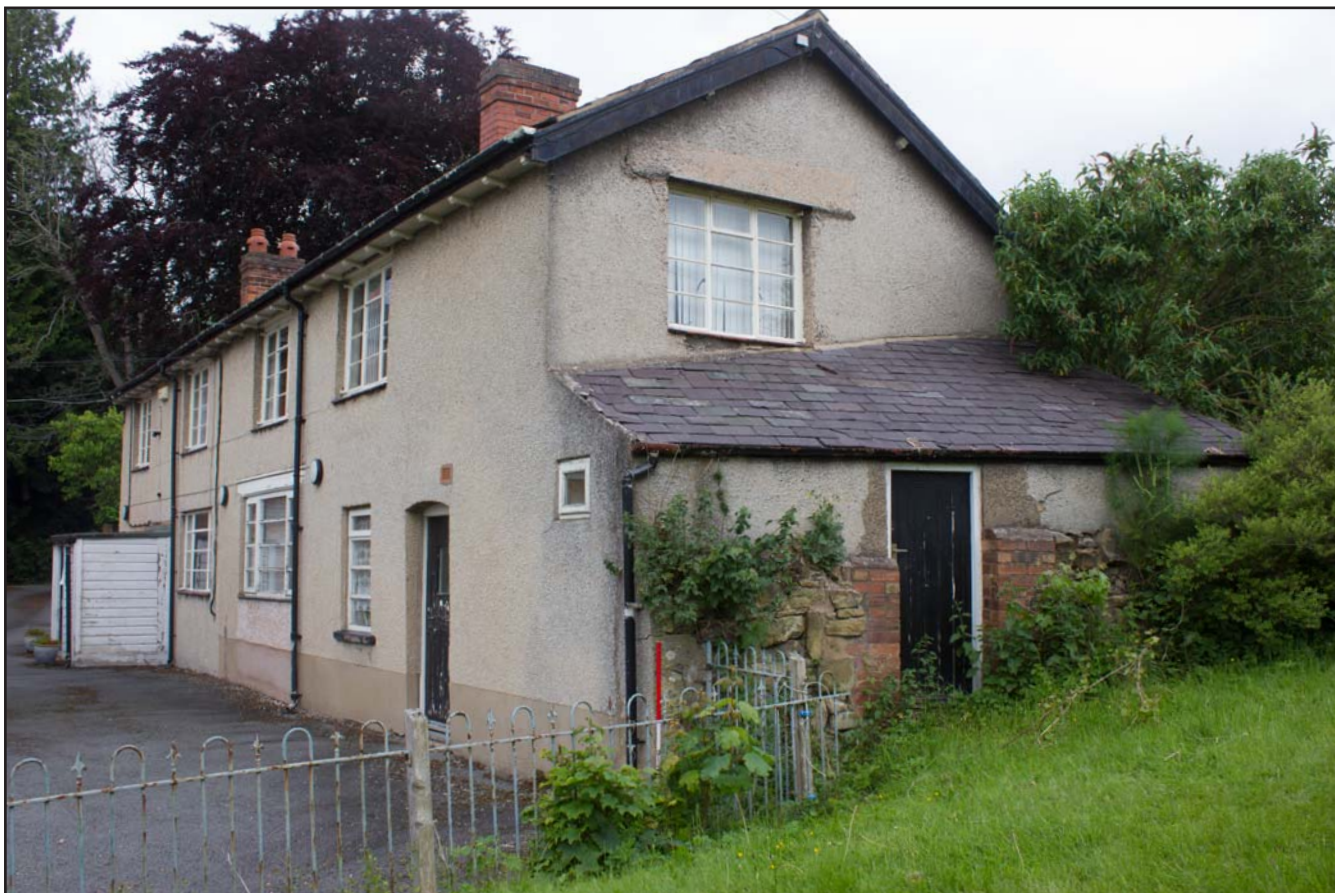
Plate 23: Oblique shot of the diocesan office, eastern and southern elevations at The Bishop's House, 17 Sontley Road, Wrexham - from the southeast - 1.00m scale
