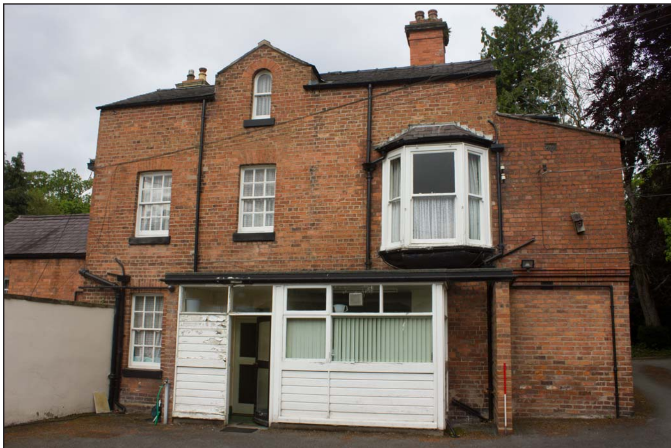
Plate 02: Rear extension, eastern elevation of The Bishop's House, 17 Sontley Road, Wrexham - from the east - 1.00m scale
