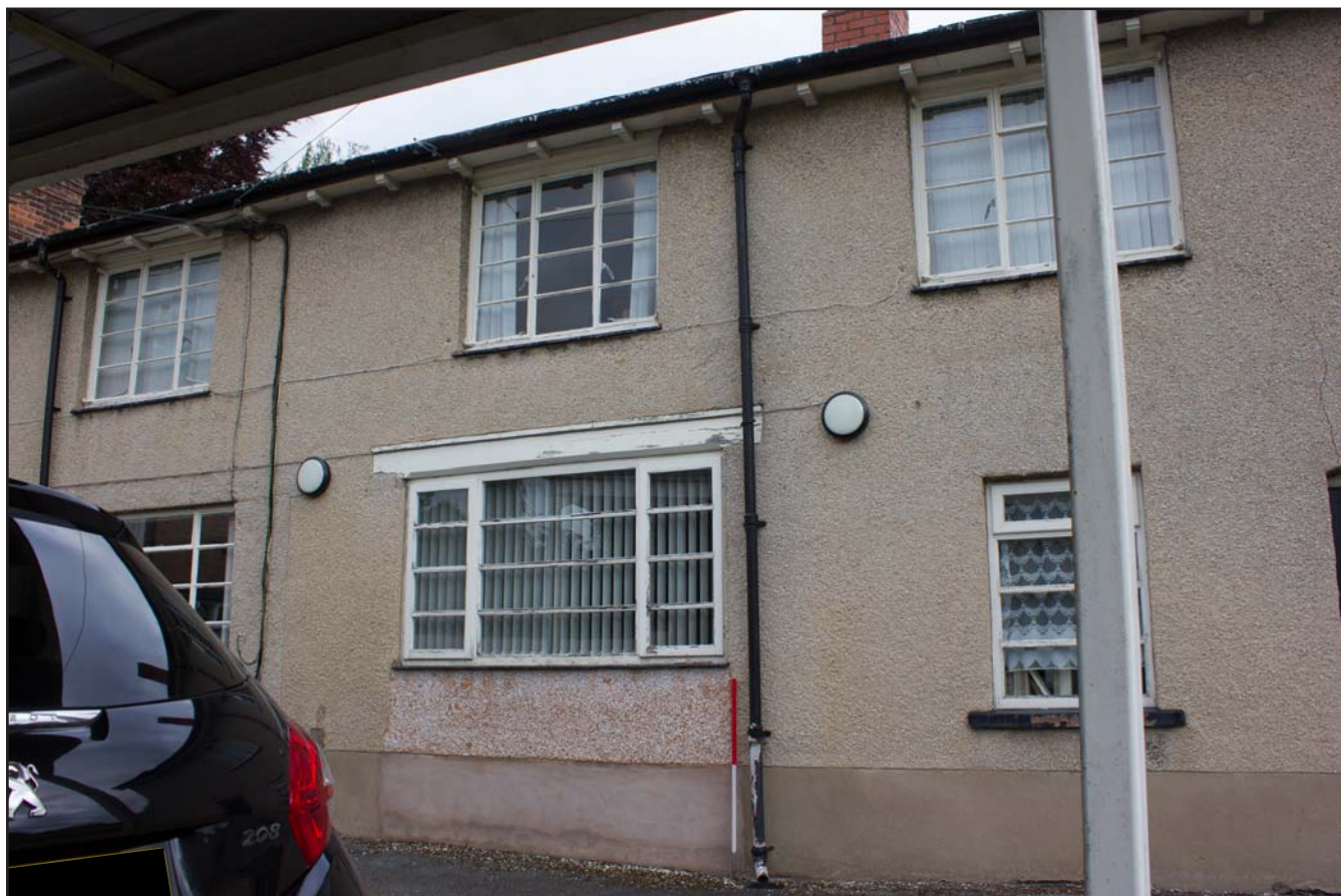
Plate 25: Southern elevation (centre) of the of the diocesan office at The Bishop's House, 17 Sontley Road, Wrexham - from the south - 1.00m scale
