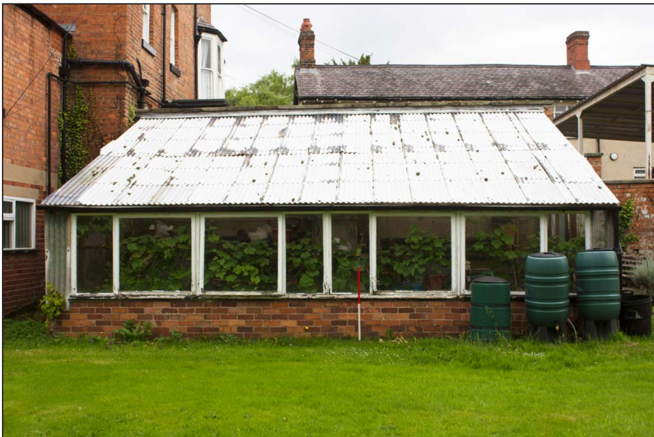
Plate 11: Southern elevation of the greenhouse in the garden at The Bishop's House, 17 Sontley Road, Wrexham - from the south - 1.00m scale
