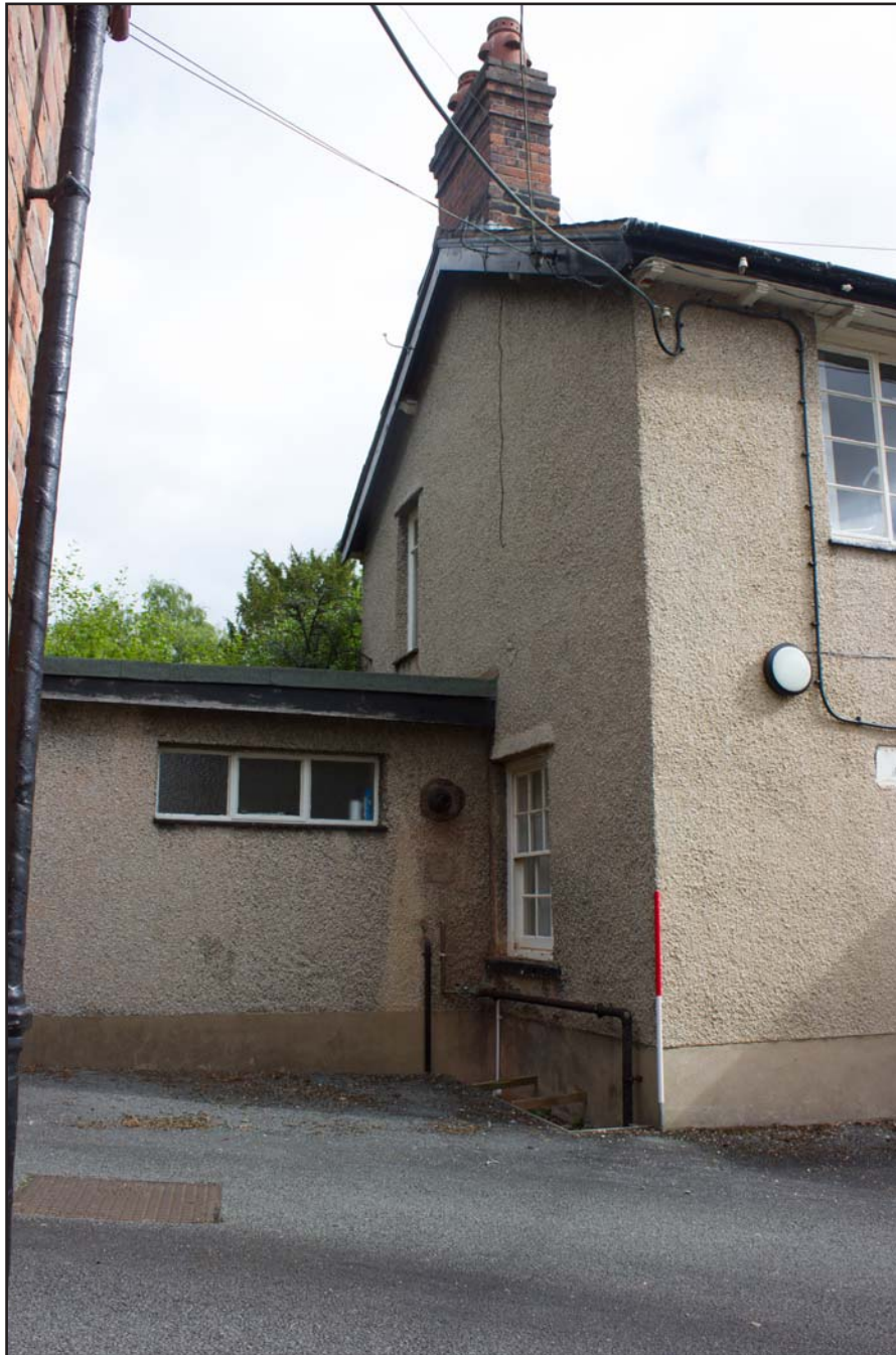
Plate 28: Oblique shot of the diocesan office, western elevation at The Bishop's House, 17 Sontley Road, Wrexham - from the southwest - 1.00m scale
