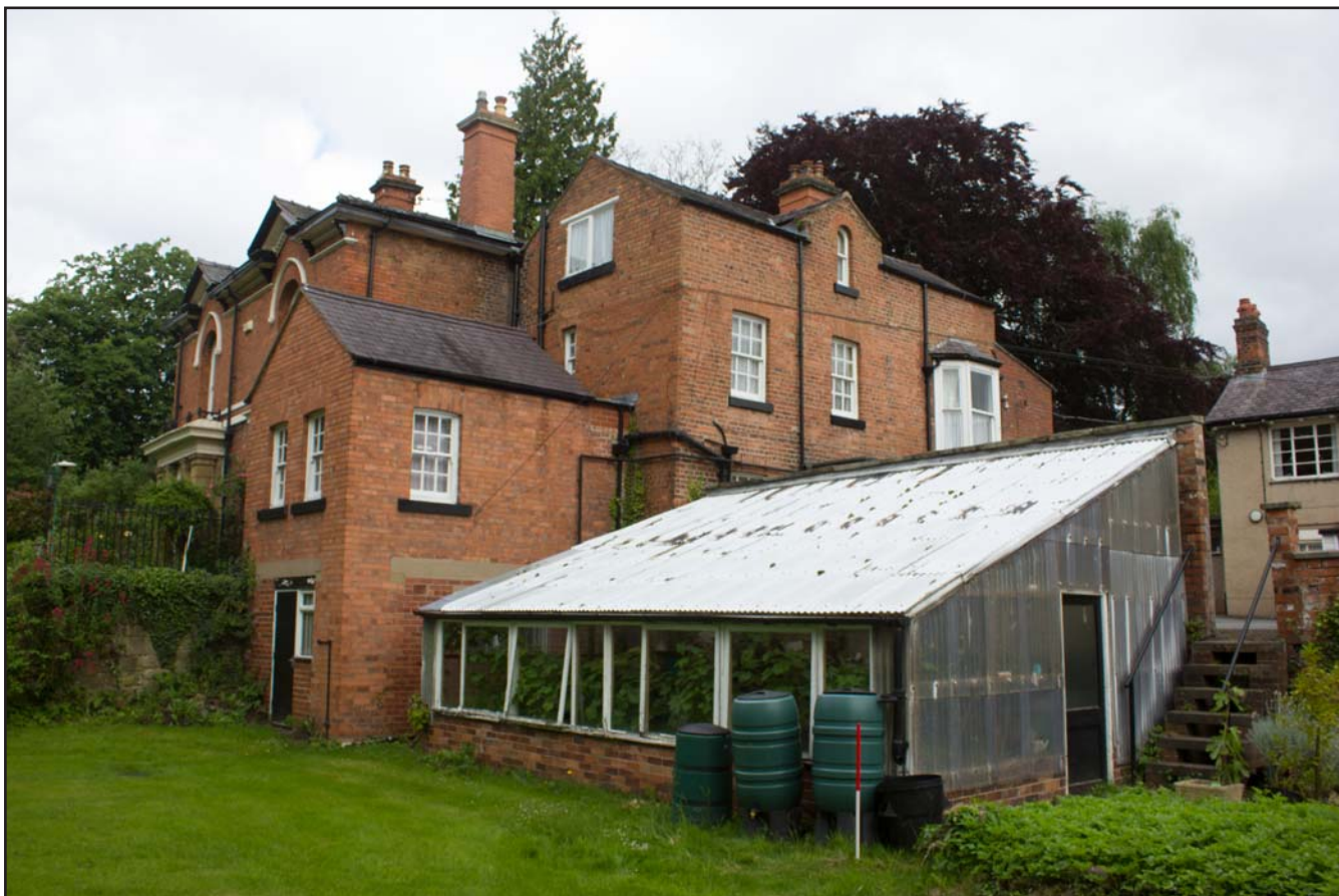
Plate 07: Context shot of the greenhouse situated to south of house, The Bishop's House, 17 Sontley Road, Wrexham - from the southeast - 1.00m scale
