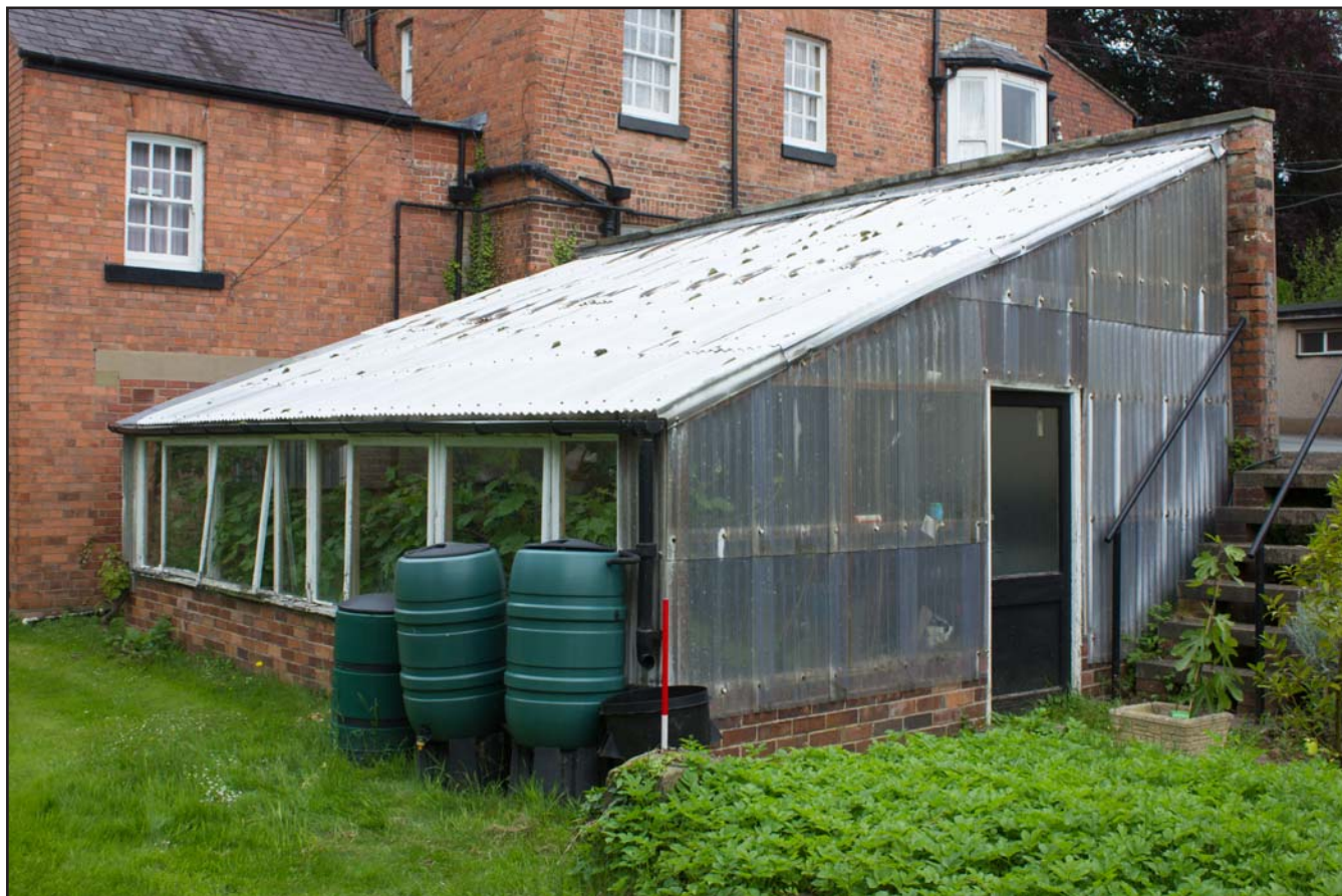
Plate 10: Oblique shot of the greenhouse, eastern and southern elevations at The Bishop's House, 17 Sontley Road, Wrexham - from the southeast - 1.00m scale
