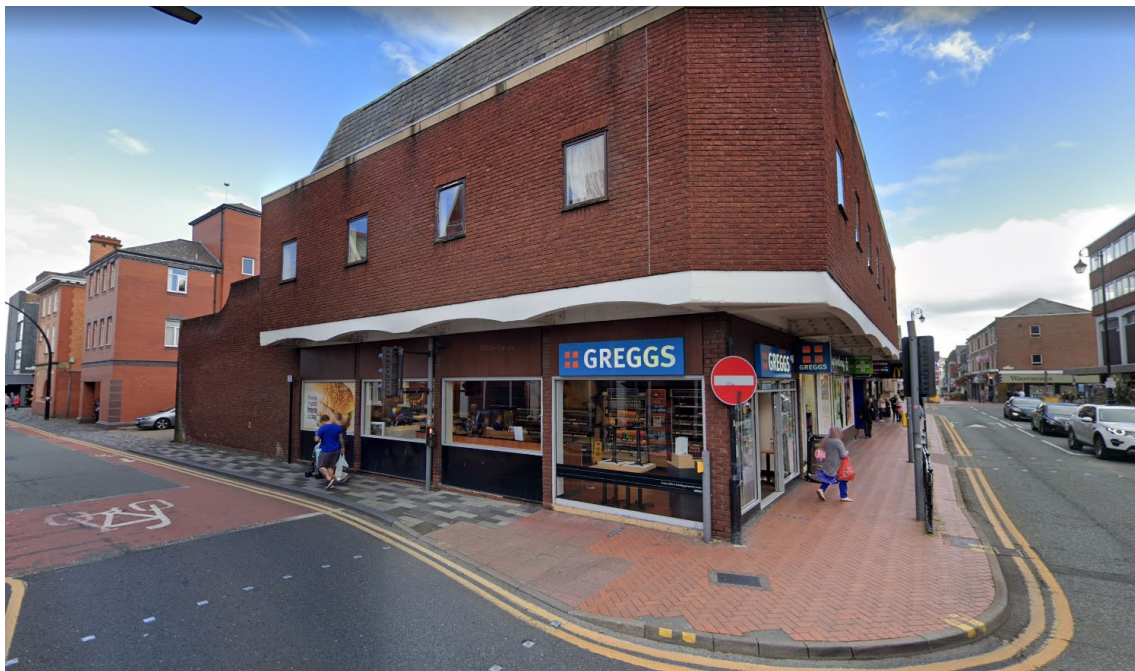
Existing shopfront – return elevation
