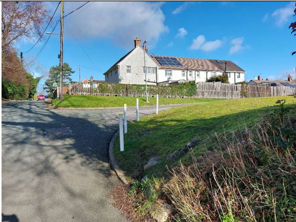
Photograph 2 – Facing north up Vicarage Hill at the site entrance
