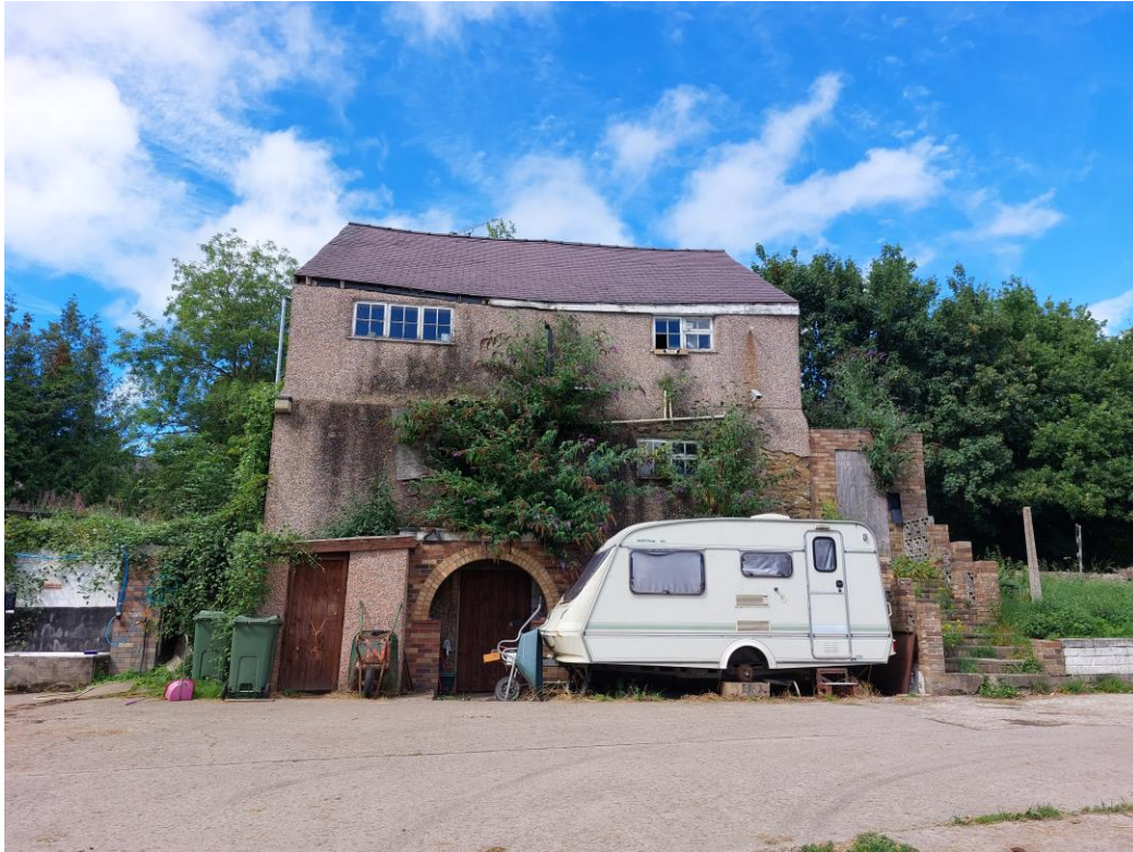
Figure 3. Front of Chapel Farmhouse currently.
