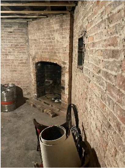
View of the ground floor front room.
