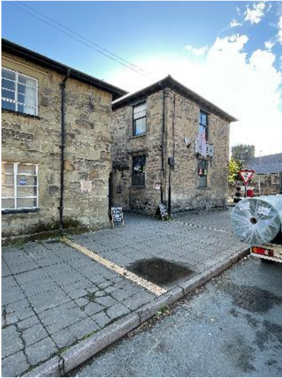
View of the front NW elevation
