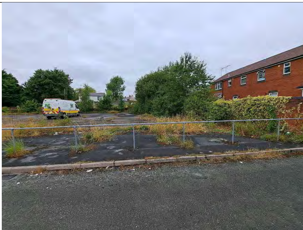
2 – Northwestern area of site, concrete slab visible and adjacent residential properties
