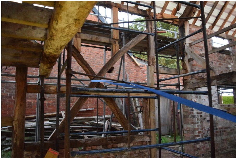
Figure 4.3. View from interior through eastern elevation
