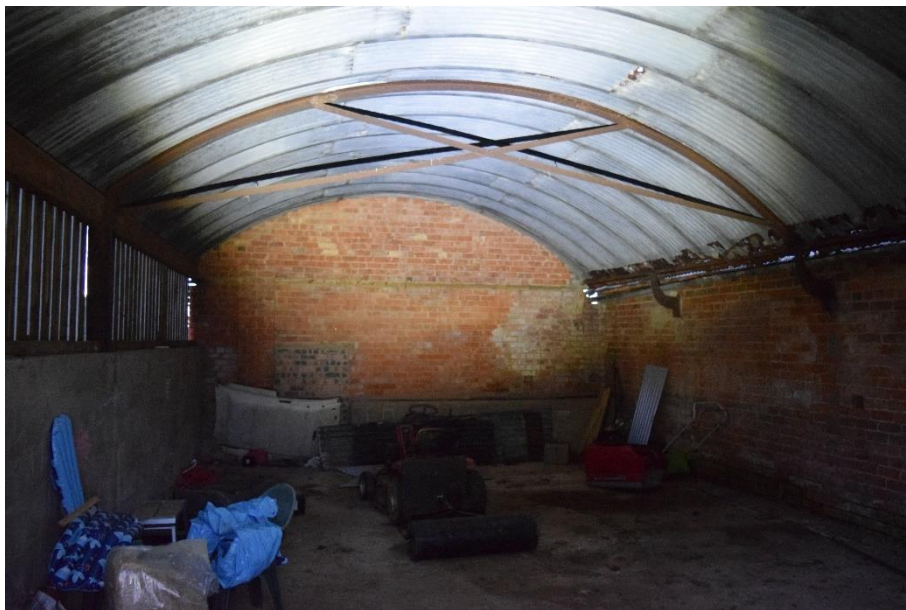
Figure 4.12. Interior of B1.4
