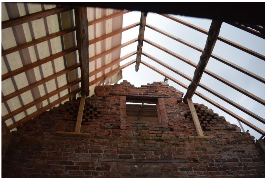
Figure 4.5. Southern gable end
