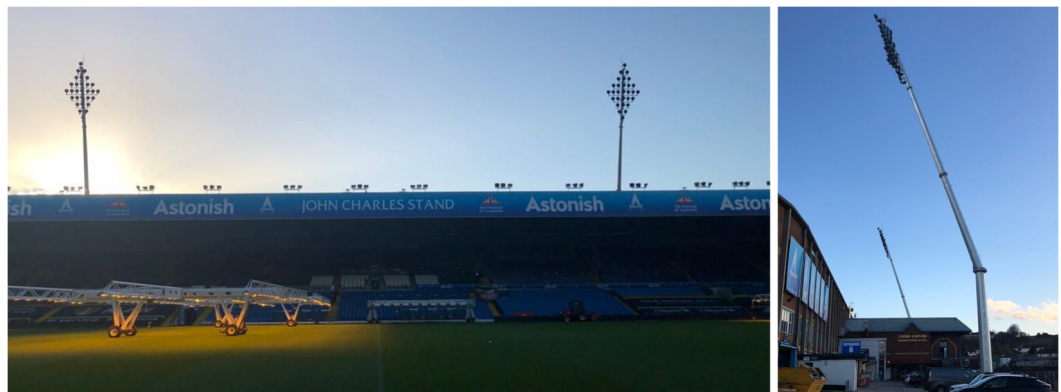
Figure 2 – Lighting Columns with Cantilever Tilt at Leeds UTD Ground
