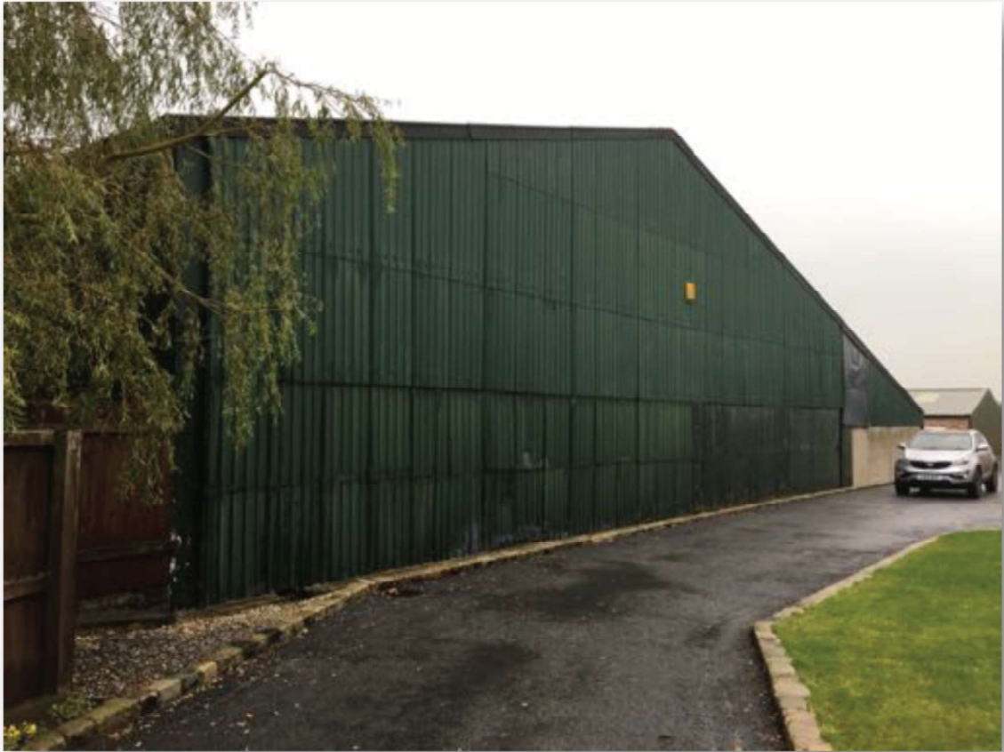
PHOTOGRAPH 3: NORTH ELEVATION OF FORMER OUTBUILDING PREVIOUSLY GRANTED CONSENT TO BE REMOVED AS PART OF PLANNING APPLICATION (P/2016/0409)
