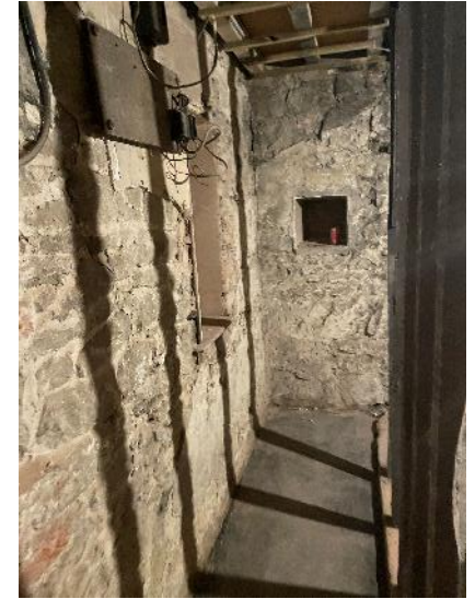
View of the partition to be removed from the ground floor front room.
