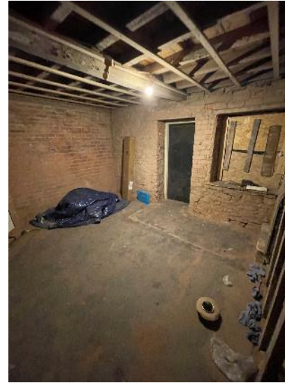
View of the rear elevation of the ground floor rear room.
