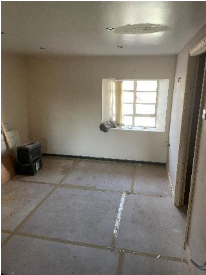
View of the first floor rear room.
