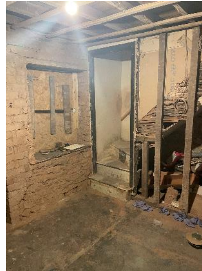
View of the existing staircase
