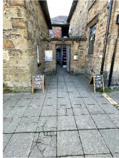
View of the passage between the two buildings.
