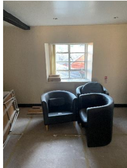
View of the first floor front room.
