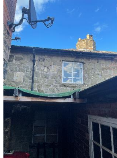
View of the rear SW elevation
