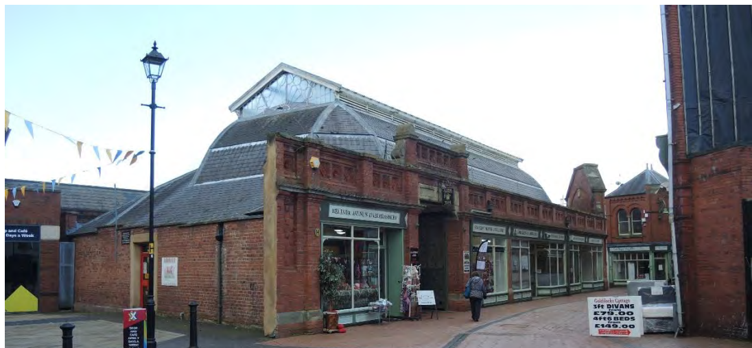
Figure 18 - Photograph of the north and west facing elevations to Henblas Street and Henblas Square
