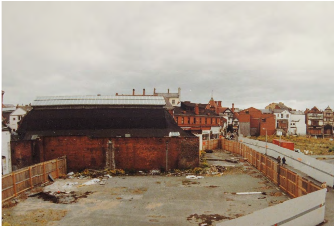
Figure 14 - Photograph taken following the demolition of The Vegetable Market Site of the east elevation to The General Market (note the 'Turnerised' roof coating and east wall details minus the current boiler room © Image from The Wrexham Museum Archive
