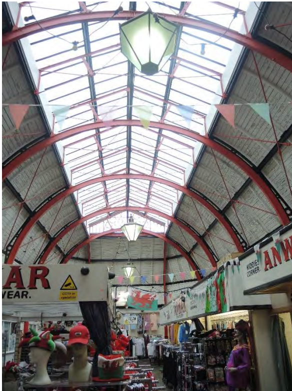
Existing internal view to the south
