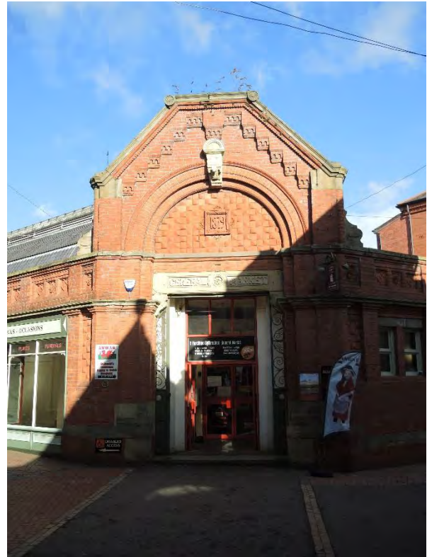
Existing entrance to the SW facing elevation
