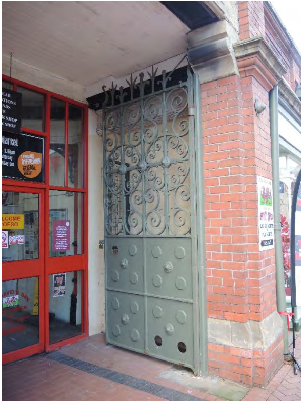
Existing Gates to the NW entrance on the West Elevation
