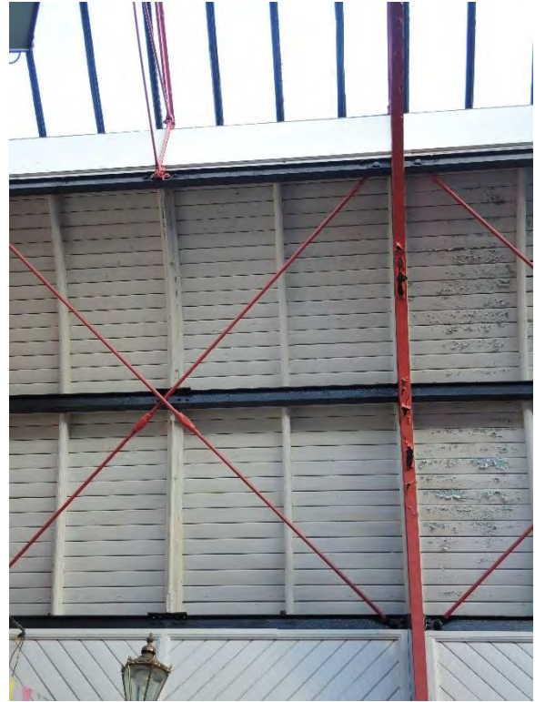
Existing roof structure
