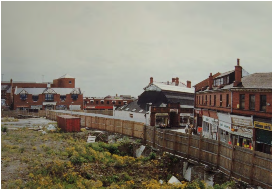
Figure 5 - Image of The General Market following the demolition of The Vegetable Market Site (note also the 'Turnerised' roof coating) © Image from The Wrexham Museum Archive
