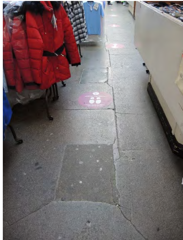
Location of previous column bases within the concrete floor
