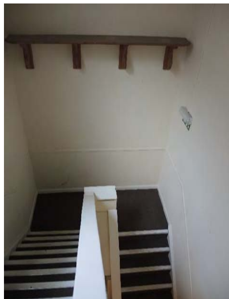
Location of existing staircase to be removed in unit 10
