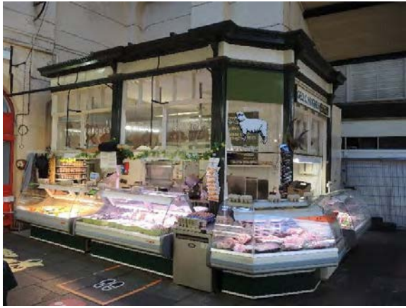
Existing permanent shopfronts to be repaired and retained
