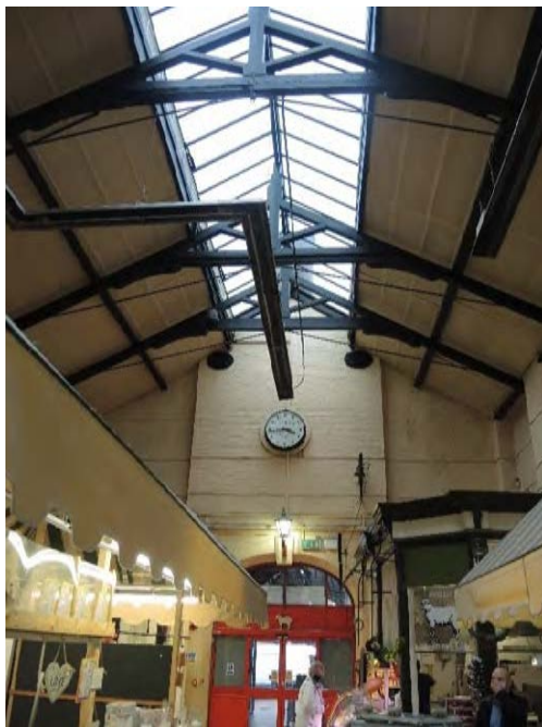
South wall into which the first floor window openings are proposed
