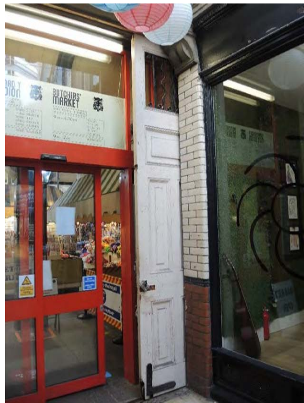
Central Arcade Entrance and Existing Sliding Doors
