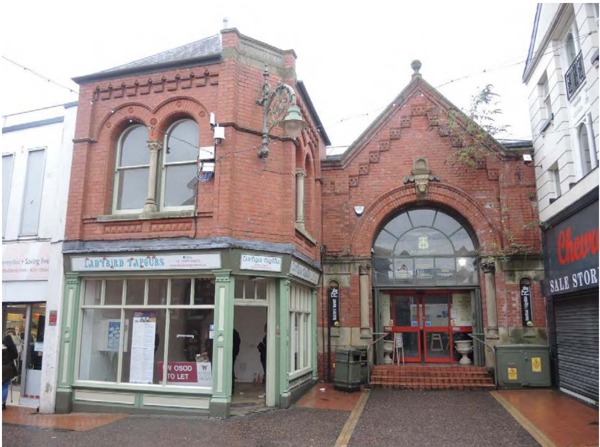
Existing Henblas Street Elevation and No.40 Henblas Street
