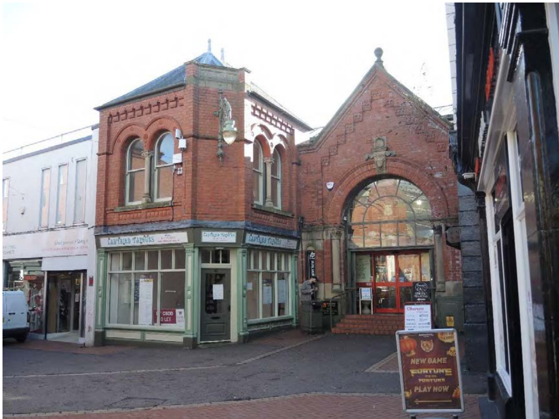
Figure 15 - Henblas Street Elevation and No.40 Henblas Street
