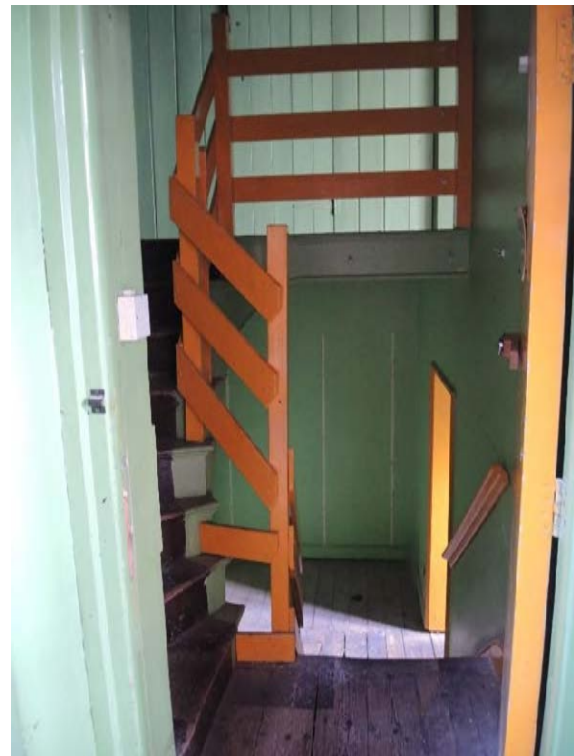
Location where staircase is to be removed above unit No.11
