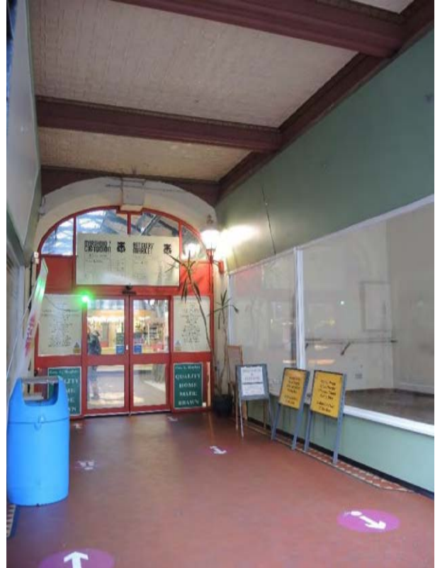
Existing inner High Street Lobby and Entrance
