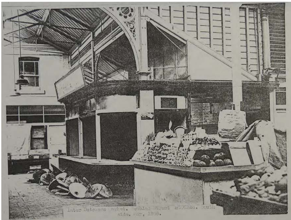
Figure 13 - Images of the Butchers Market Interior (May 1956)
