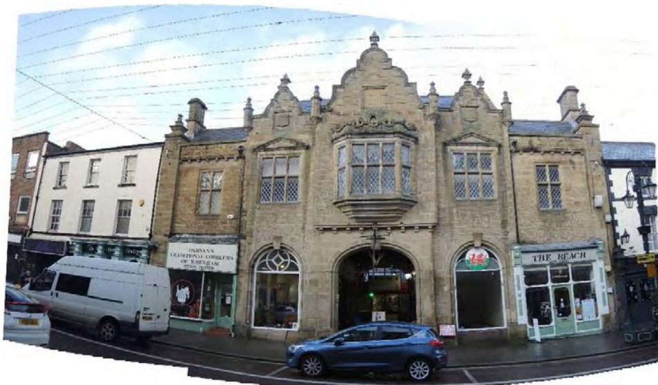
Figure 1-Existing South Facing Elevation to High Street
