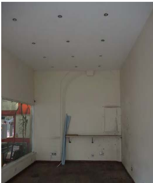
Location of existing opening to be re-established in unit 10a R/H side of the main entrance
