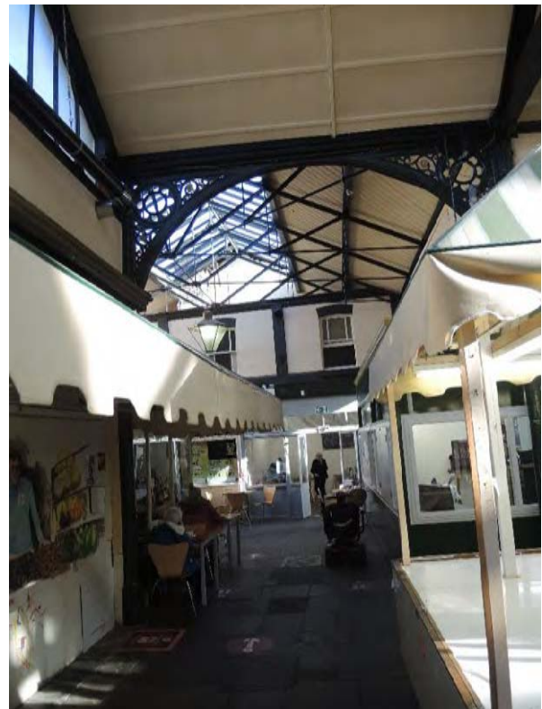
View towards units 16 & 17, north side of the Market Hall
