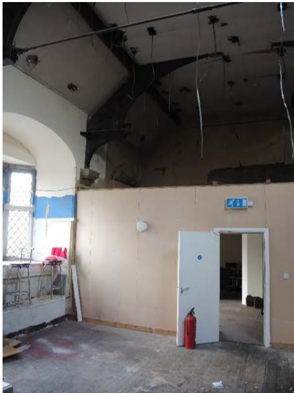
Main function room to be reinstated at first floor level
