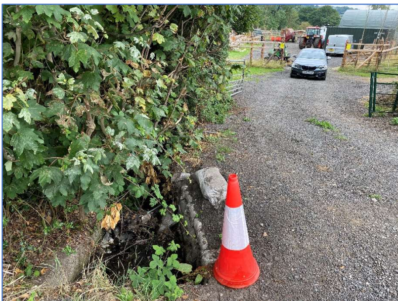
P8 – Exist of culvert adjacent to T14 – water course extends down into the site
