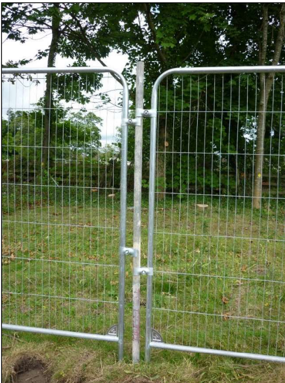
Tree Protective Fencing Specification
