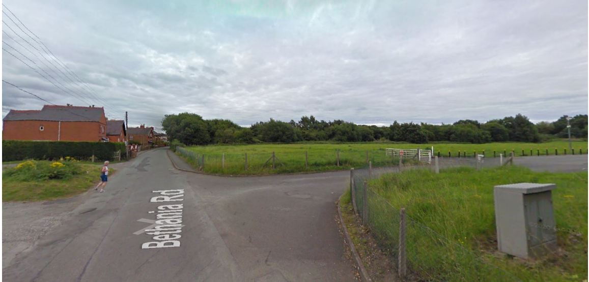
Existing site entrance
