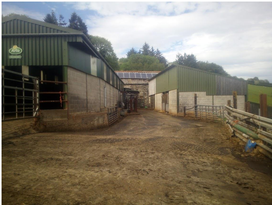
Picture showing the bottom end of the cattle dispersal area, showing the crash barriers to the right which form part of the slurry pit to be covered. The applicant states that the proposed roof will be approx. 500mm above these barriers.
